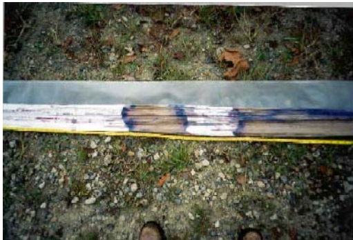
Stains on cover in 3" cored hole
