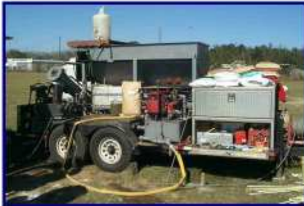
Photo 6. Photograph of hydraulic fracturing rig.
