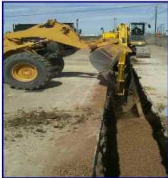
Photo 3. Backfilling PRB after installation of EHC and sand in the trench; southern USA.
