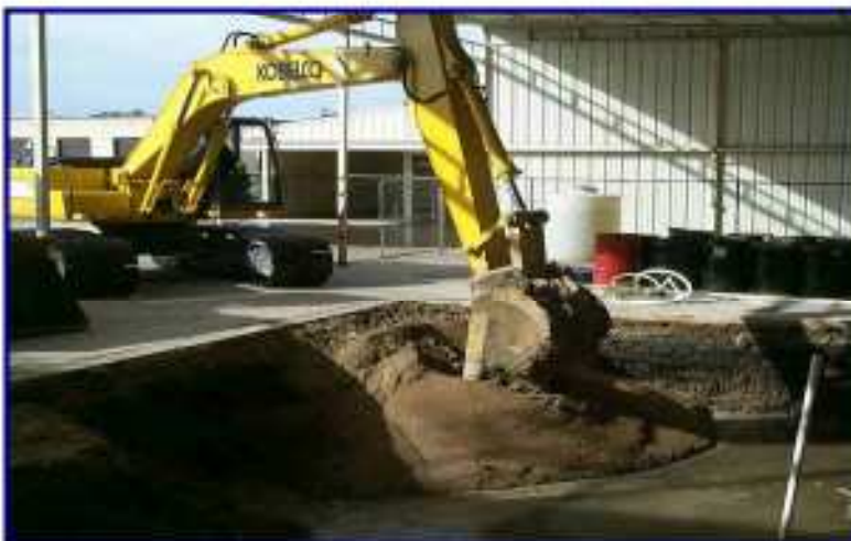
Photo 2. Picture of excavator leveling EHC and sand that were mixed together prior to placement into the excavated area
