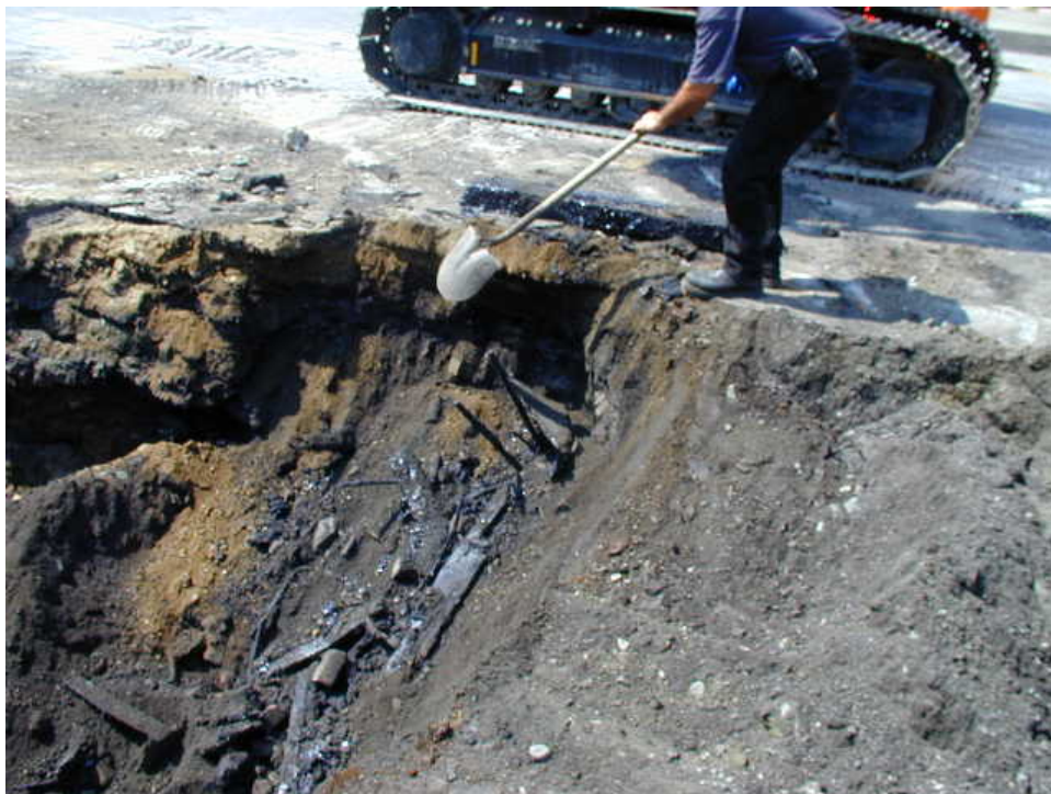
Photo 8 - Remains of one-foot by one-foot square wooden plank structure found in the center of the excavation.
