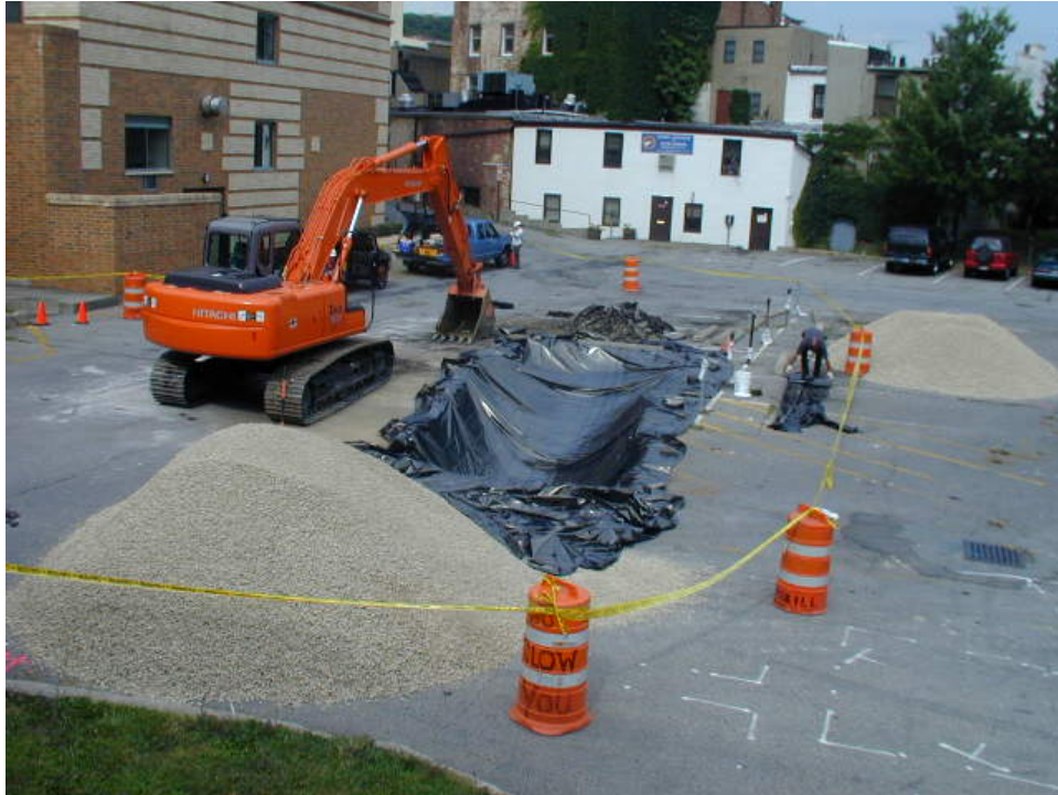
Photo 11 - Excavation secured for the night with plastic to prevent the release of odors. Backfill material (NYSDOT Item #4 stone) is shown stockpiled adjacent to the excavation for later use.
