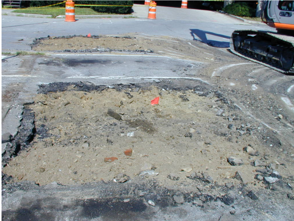
Photo 3 - View of the parking lot looking west showing the soil immediately beneath the asphalt in the excavation areas around soil boring SB-8 (background) and SB-6 (foreground). The red flags show the locations of the soil borings.
