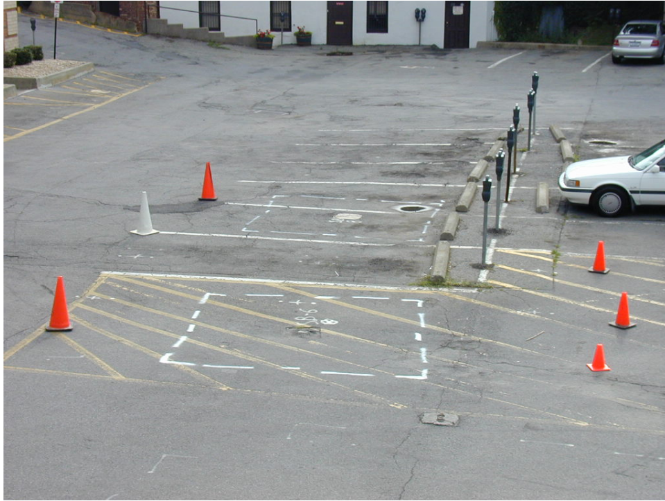
Photo 1 - View of the excavation area looking towards the east. The square areas outlined in white dashed lines show the initial areas to be excavated surrounding SB-6 (foreground) and SB-8 (background).
