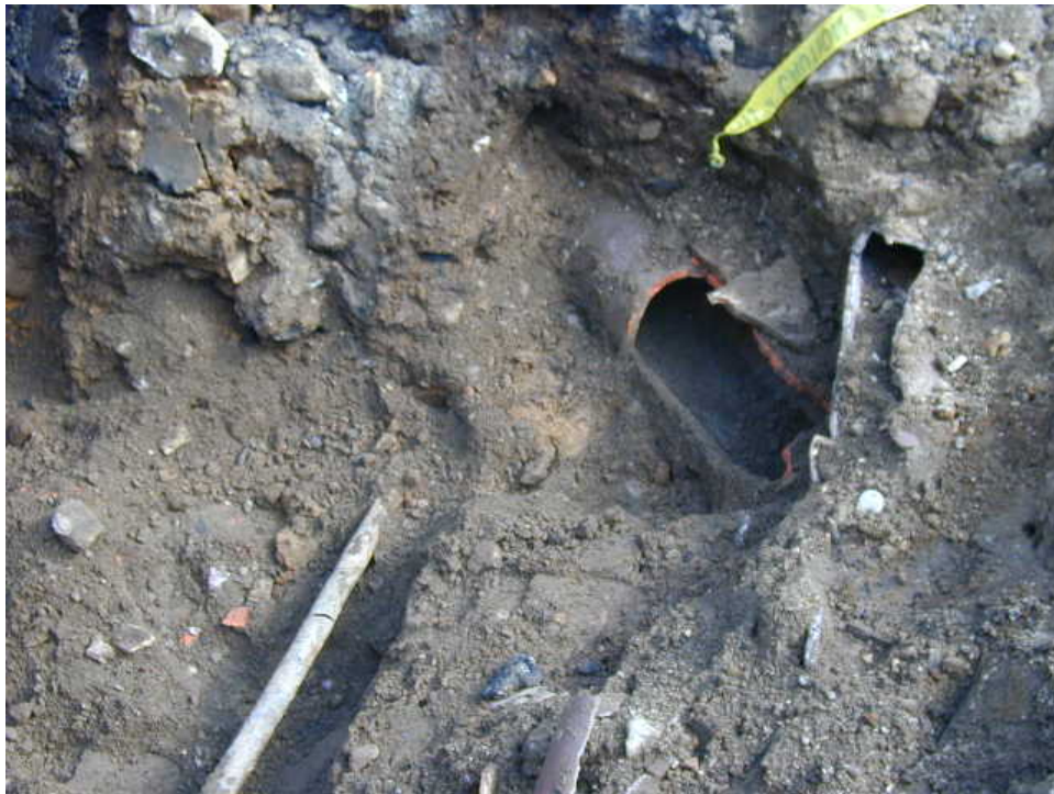
Photo 10 - Clay pipes uncovered beneath the southwest corner of the excavation.
