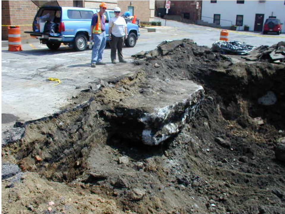
Photo 9 - View looking to the northeast showing the concrete slab along the north wall of the excavation. Note that removal of the affected soils required expansion of the initial excavations to create one excavation.
