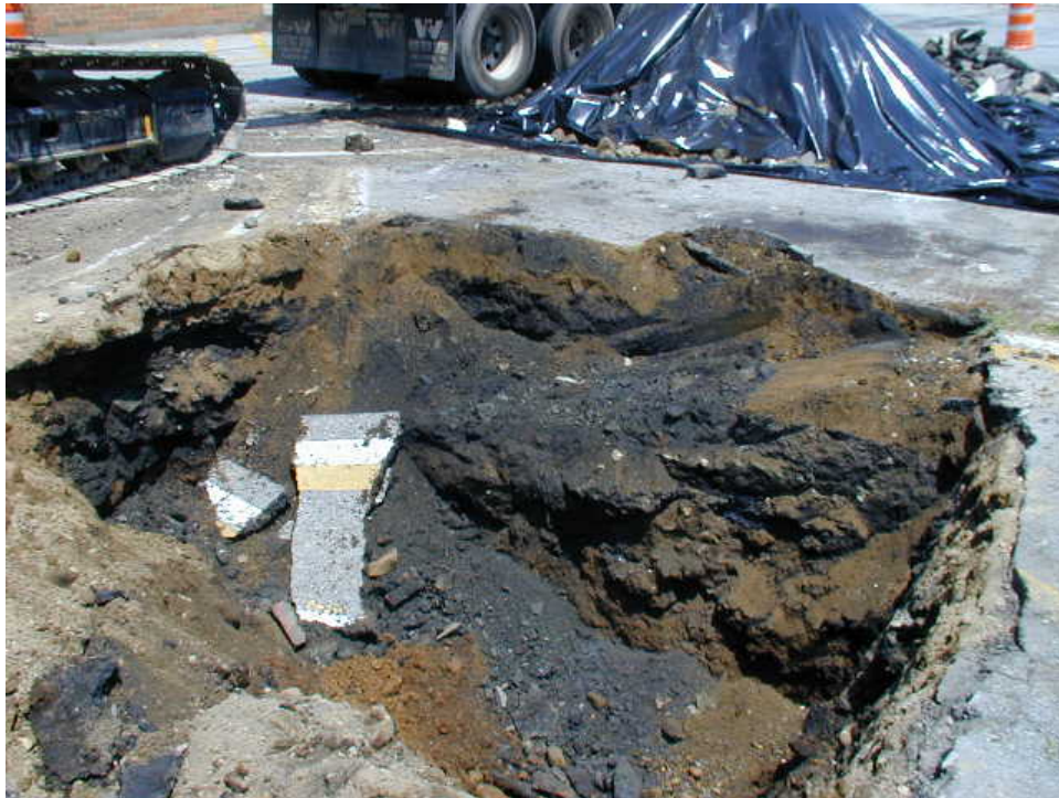
Photo 4 - View of the east wall of the excavation at SB-6 on the first day of excavation, showing impacted soils in the sidewall.
