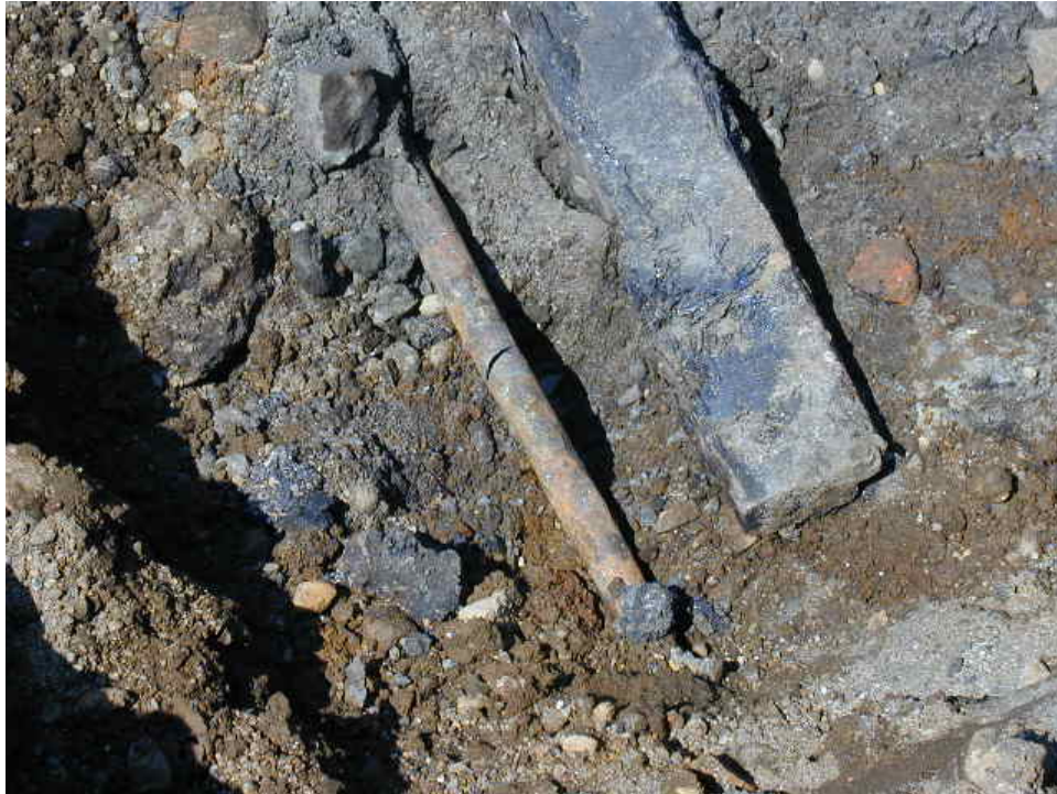
Photo 7 - A two-inch diameter iron pipe uncovered along west wall of excavation. Soils surrounding this pipe in the northwest portion of the excavation exhibited a petroleum-like odor.
