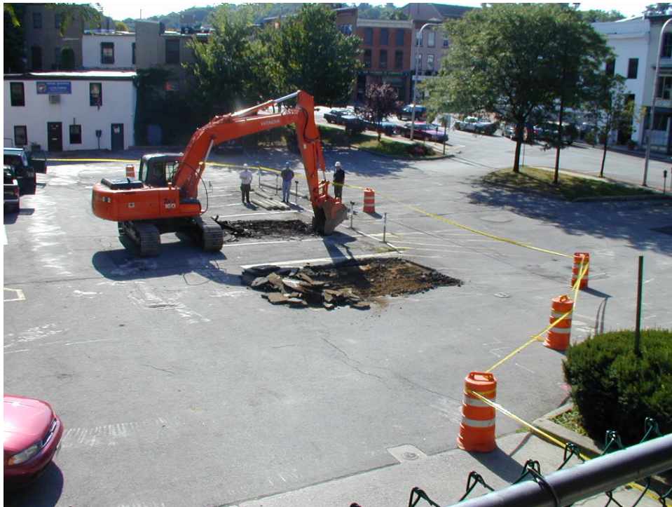
Photo 2 - View of excavation area looking southeast. The asphalt has been removed from the two excavation areas. The pedestrian walkway to the stairs into the garage can be seen on the right side of the photo.
