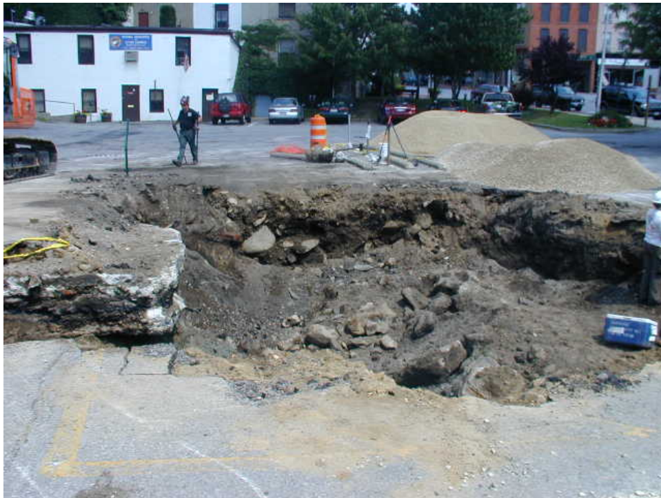
Photo 12 - View to east showing the maximum extent of excavation. Note the concrete slab at the left side of the photo.
