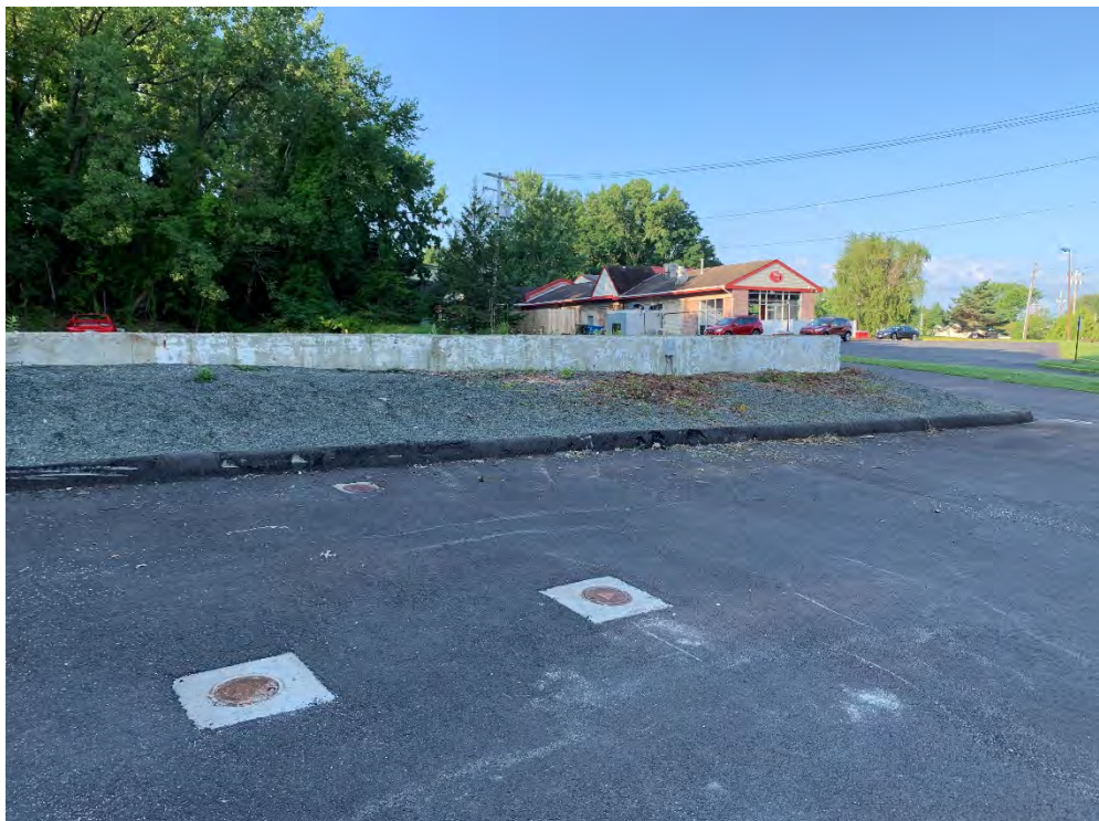
Photo 10: Asphalt cap condition (facing south).
