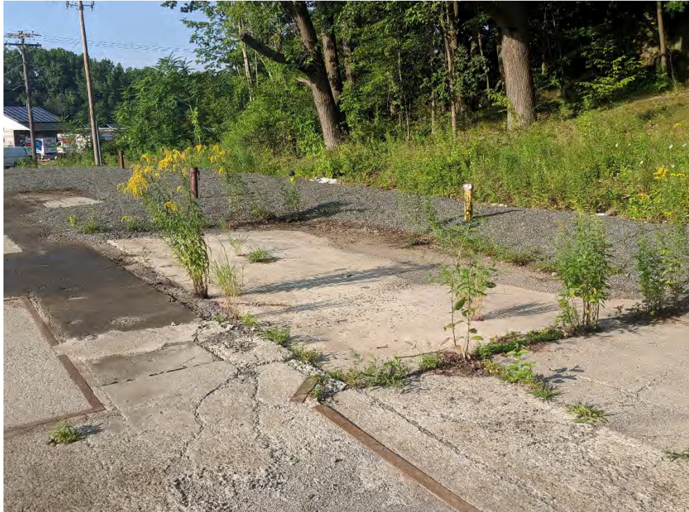
Photo 3: Concrete and stone cap before vegetation removal (facing north).
