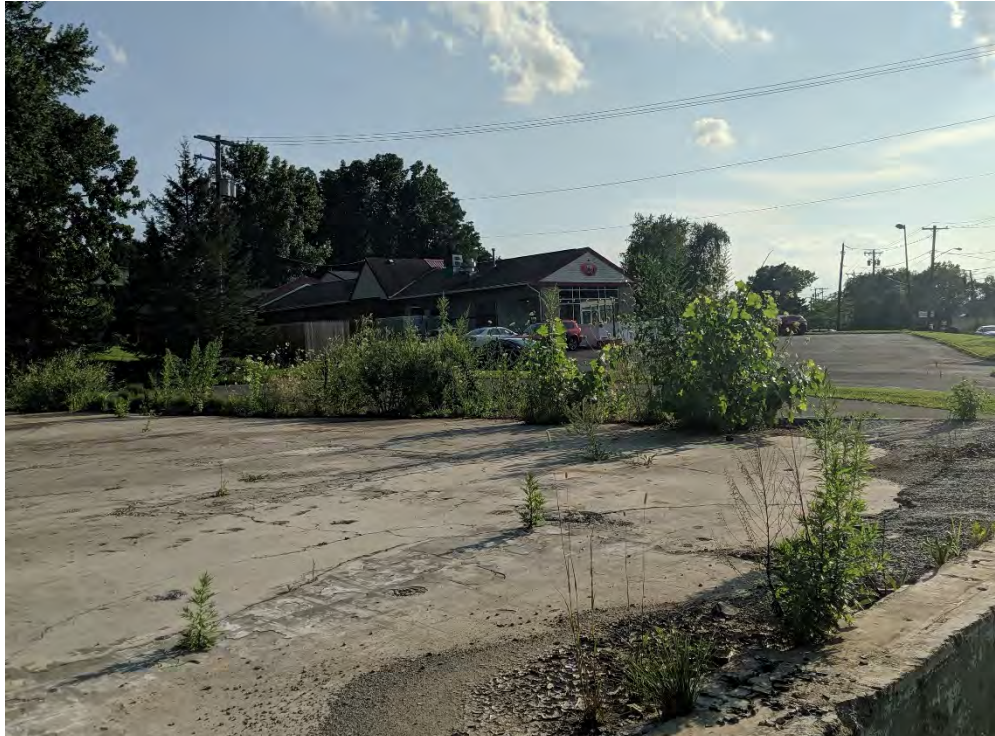
Photo 1: Concrete cap condition before vegetation removal (facing southwest).
