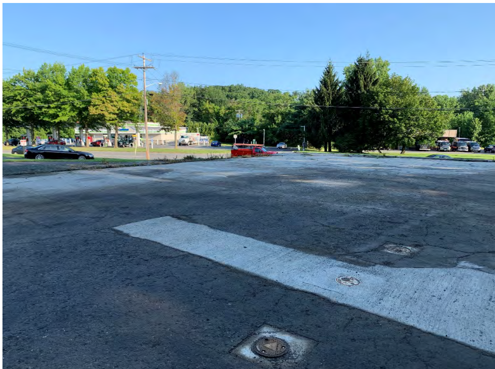
Photo 2: Concrete cap condition after vegetation removal (facing northwest).
