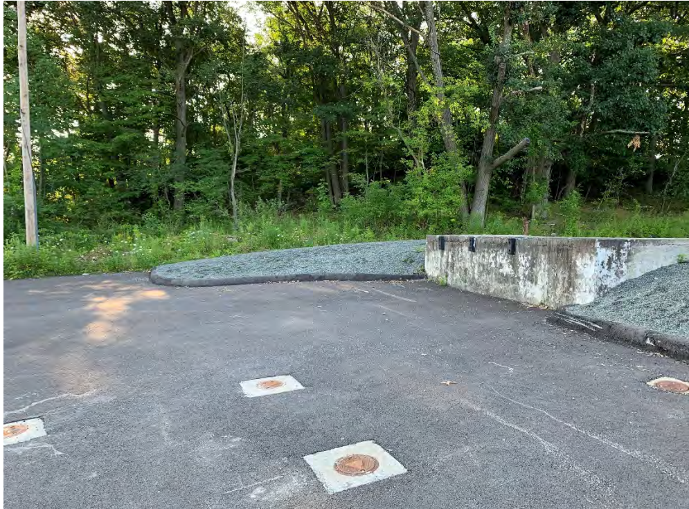
Photo 9: Asphalt cap condition (facing east).
