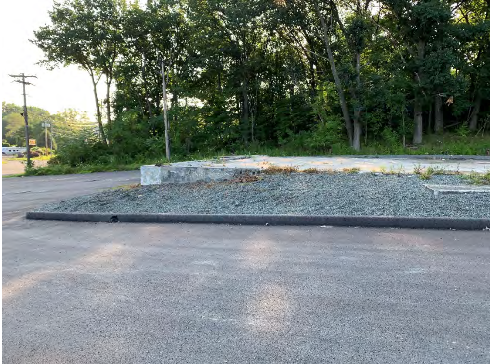
Photo 11: Asphalt cap condition (facing east).
