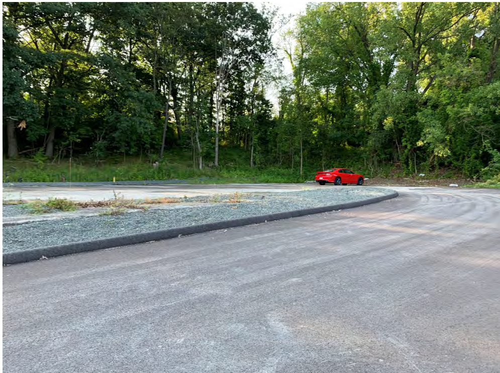
Photo 12: Asphalt cap condition (facing southeast).
