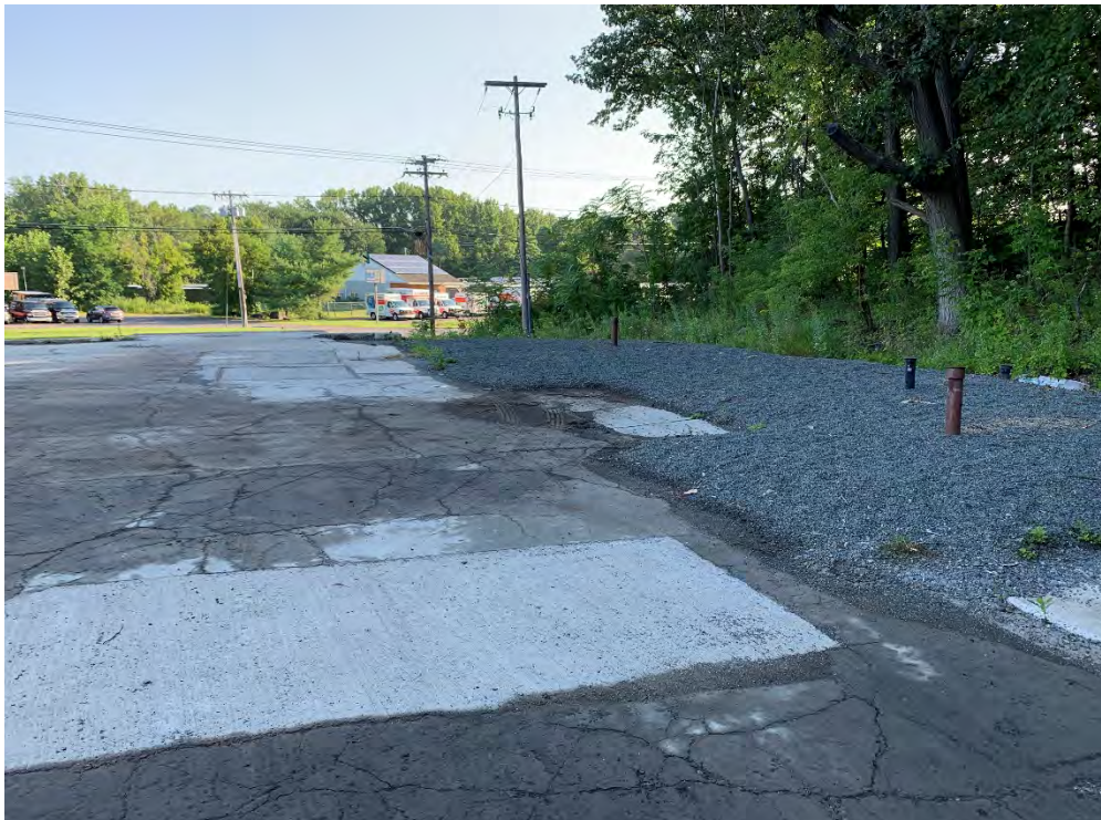
Photo 4: Concrete and stone cap after vegetation removal (facing north).
