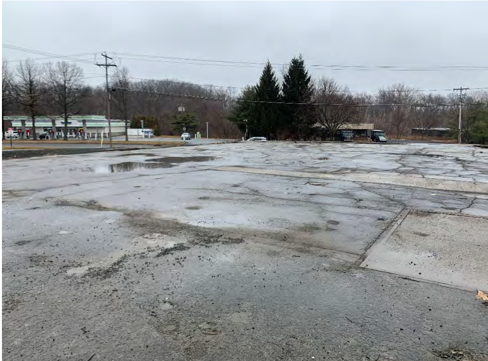
Photo 1: Concrete cap condition (facing northwest).
