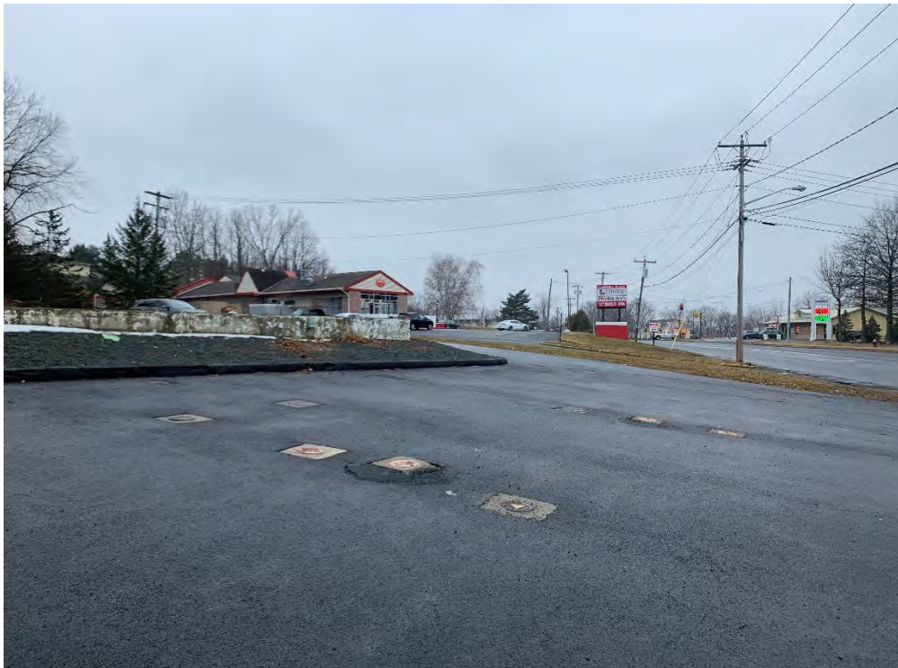
Photo 10: Asphalt cap condition (facing southwest).
