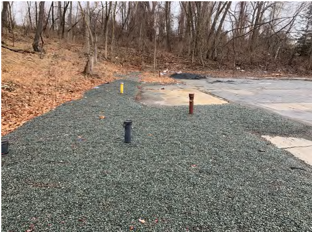
Photo 4: Concrete and stone cap condition (facing south).
