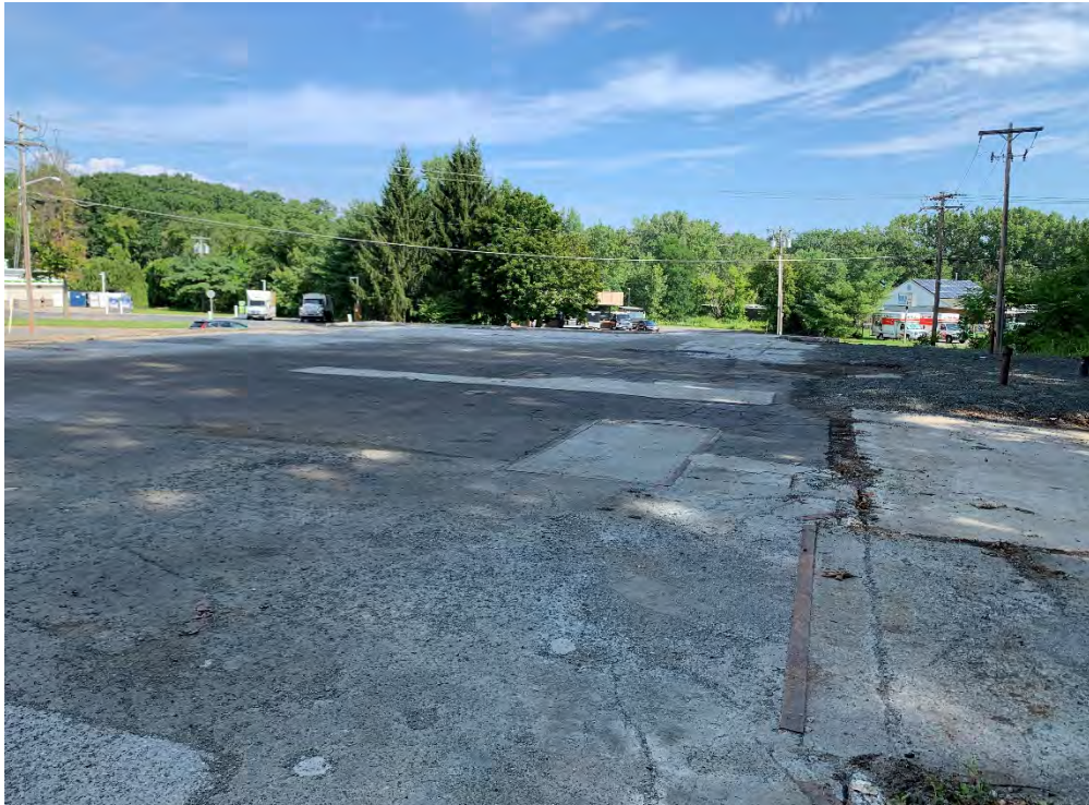
Photo 7: Concrete and stone cap condition (facing north).
