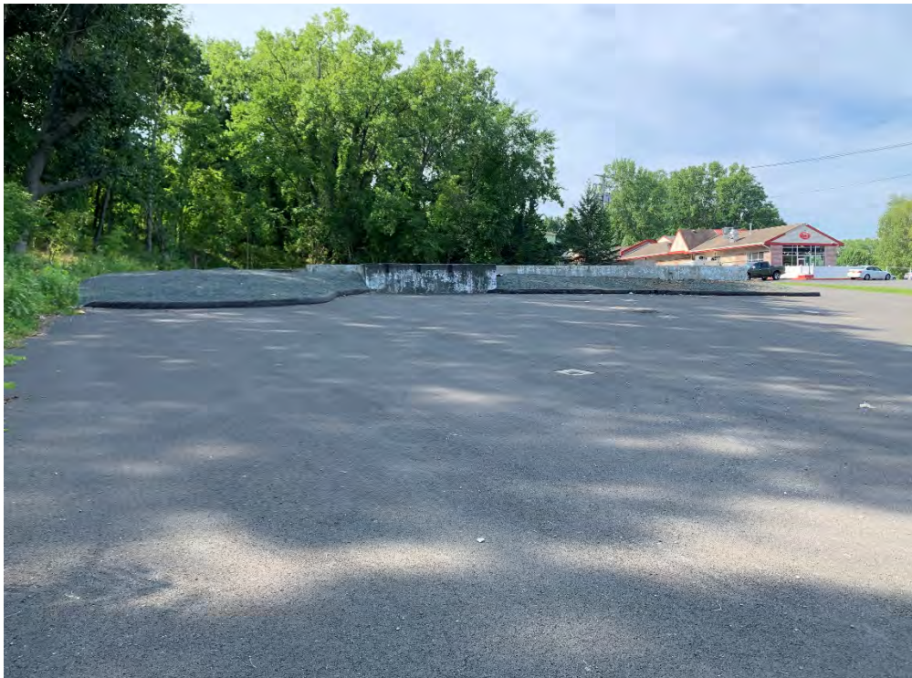
Photo 12: Former building foundation, stone, and asphalt cap condition (facing north).
