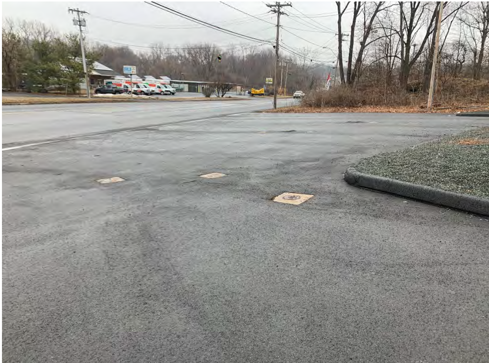
Photo 11: Asphalt cap condition (facing northeast).
