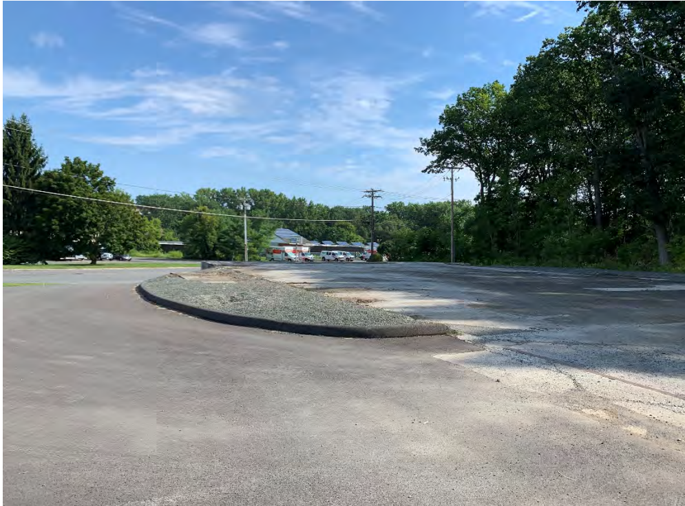
Photo 15: Concrete, stone, and asphalt cap condition (facing northeast).
