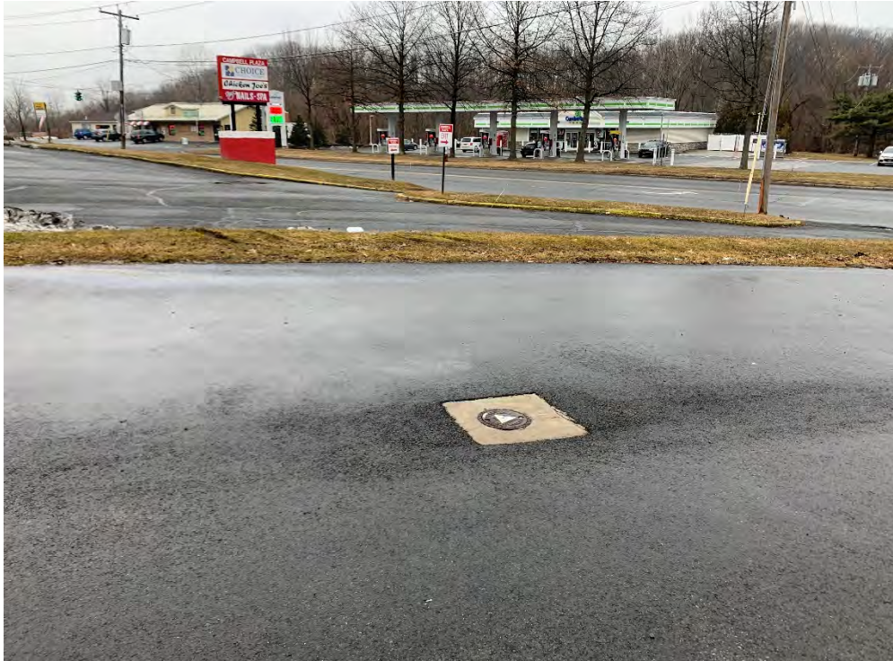
Photo 13: Asphalt cap condition (facing northwest).
