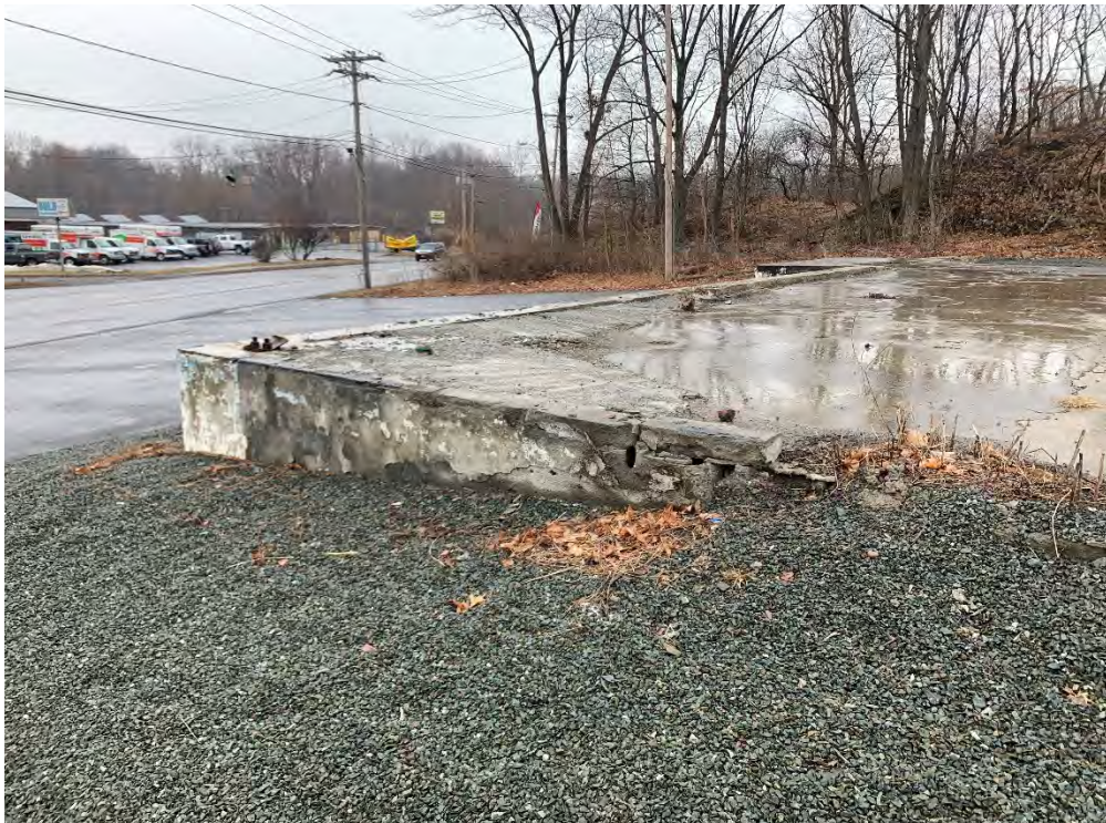
Photo 6: Concrete and stone cap condition (facing northeast).
