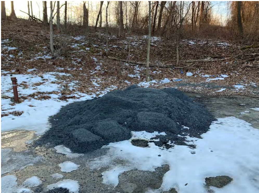
Photo 14: Pile of stone observed in southeastern corner of concrete cap (facing southeast).
