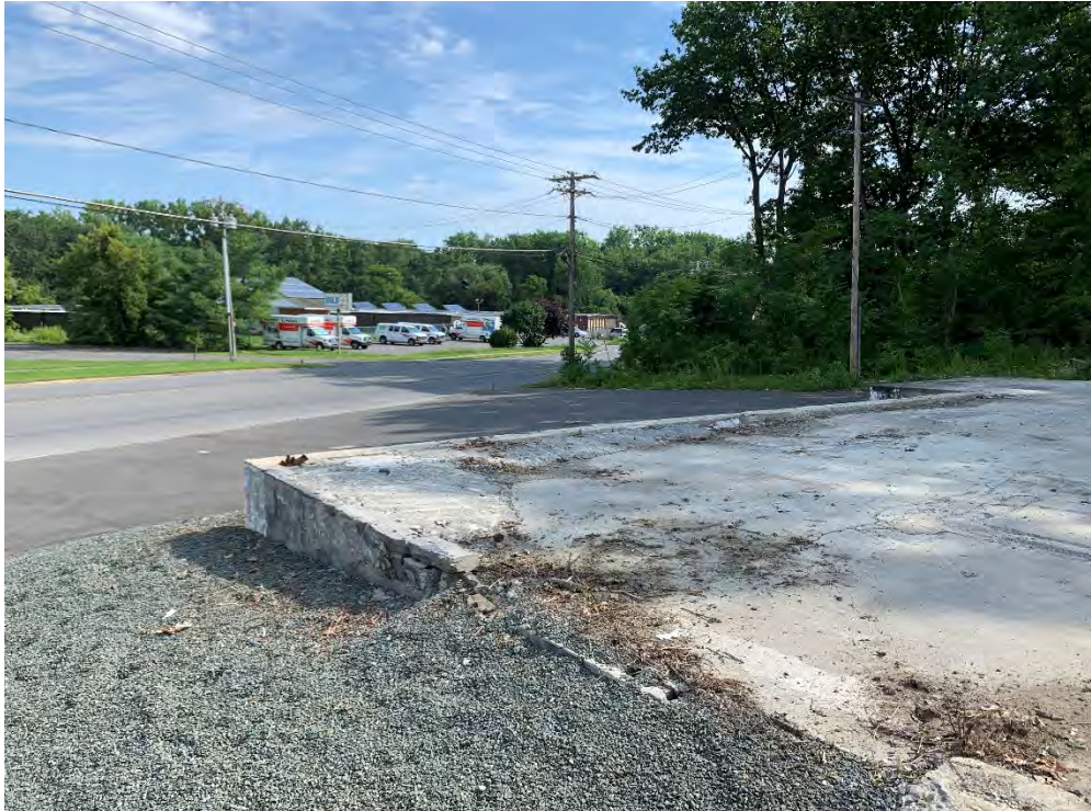
Photo 9: Former building foundation, stone, and concrete cap condition (facing northeast).
