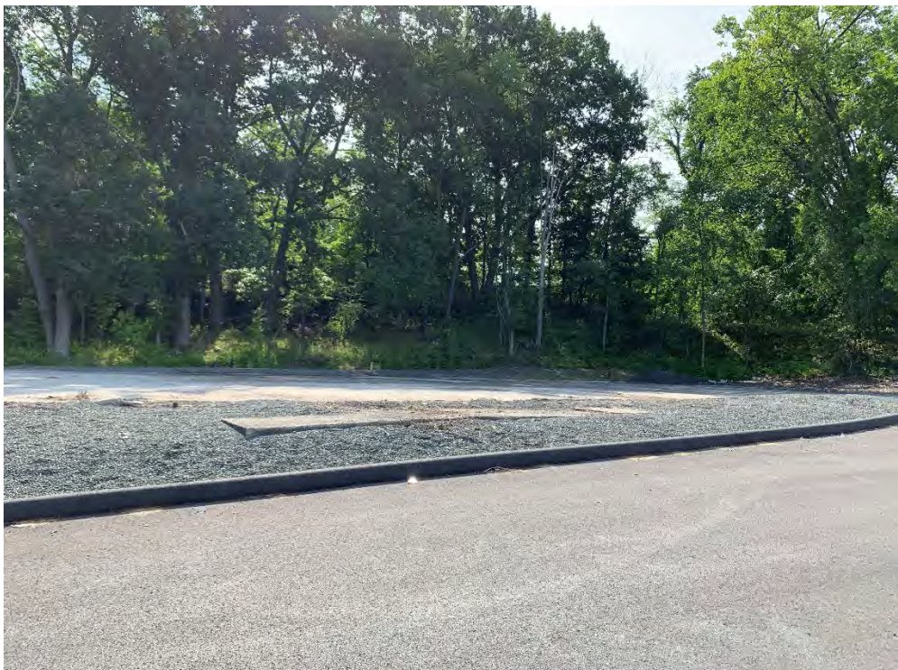
Photo 16: Asphalt, stone, and concrete cap condition (facing southeast).
