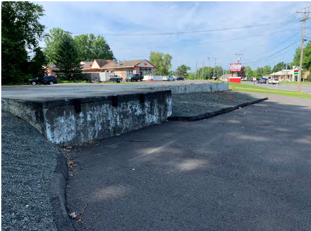
Photo 10: Former building foundation, stone, and asphalt cap condition (facing southwest).
