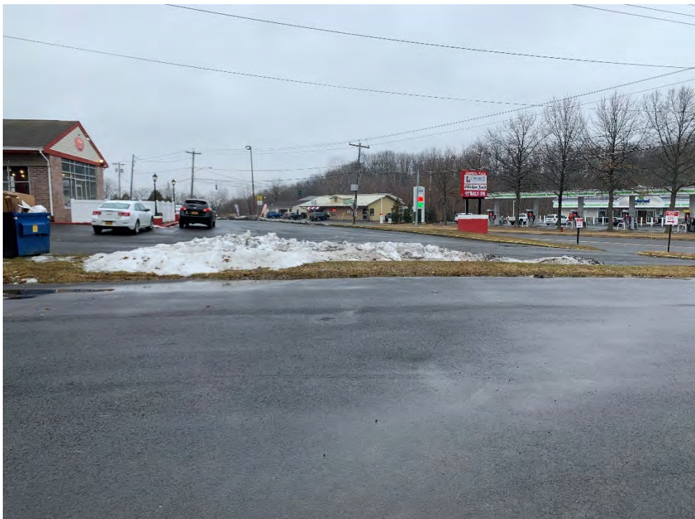
Photo 12: Asphalt cap condition (facing west).
