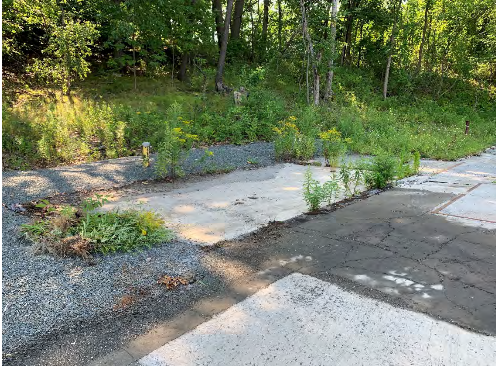
Photo 5: Concrete cap condition prior to vegetation removal (facing southeast).
