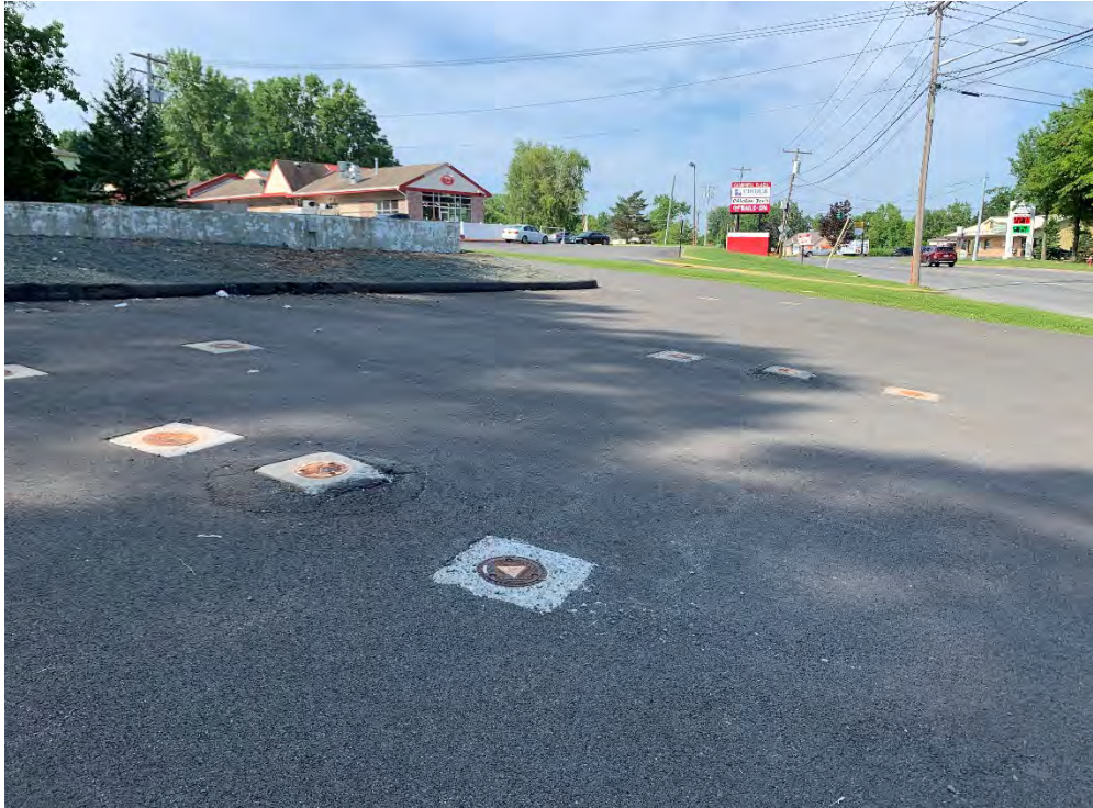
Photo 13: Asphalt cap condition (facing southwest).
