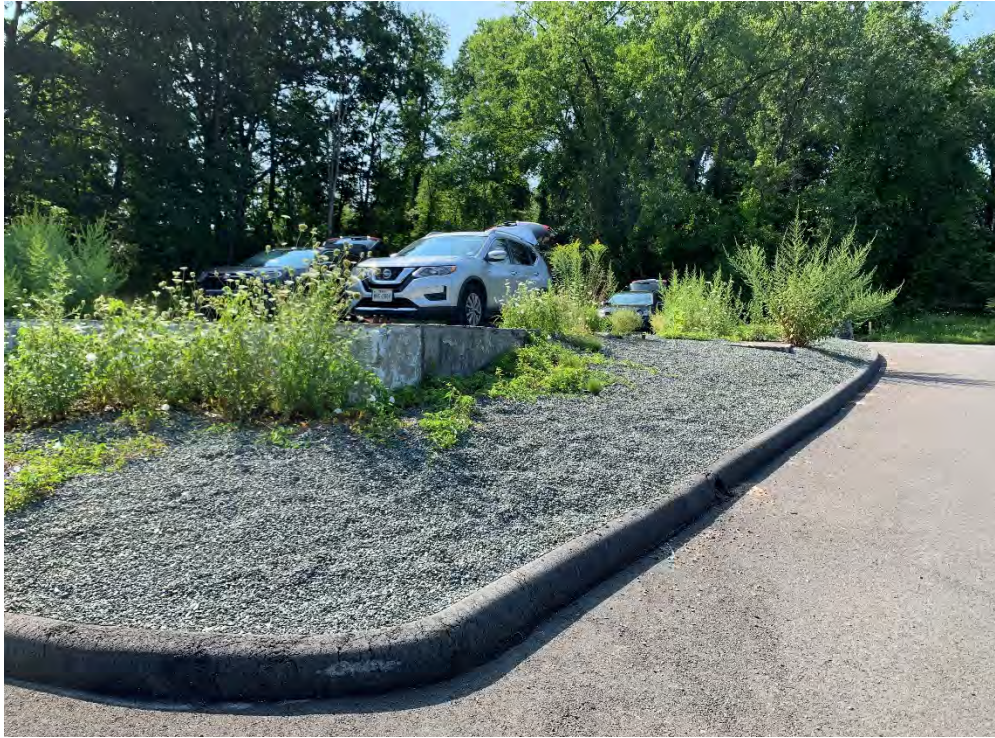
Photo 1: Concrete cap condition prior to vegetation removal (facing southeast).
