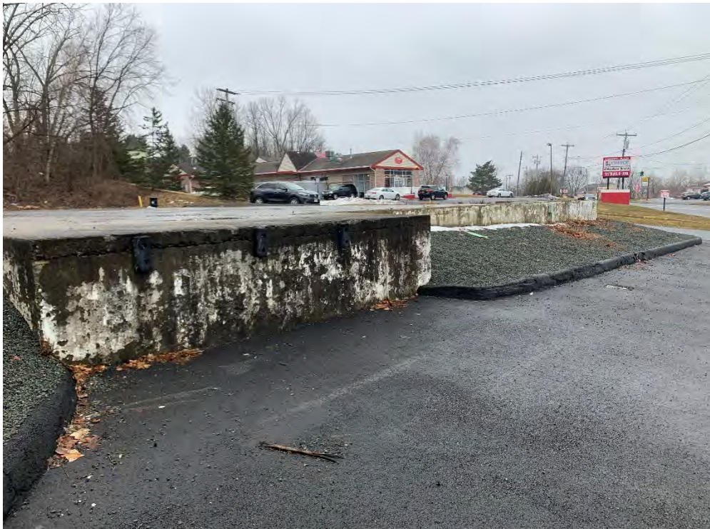
Photo 8: Former building foundation, stone, and asphalt cap condition (facing southwest).
