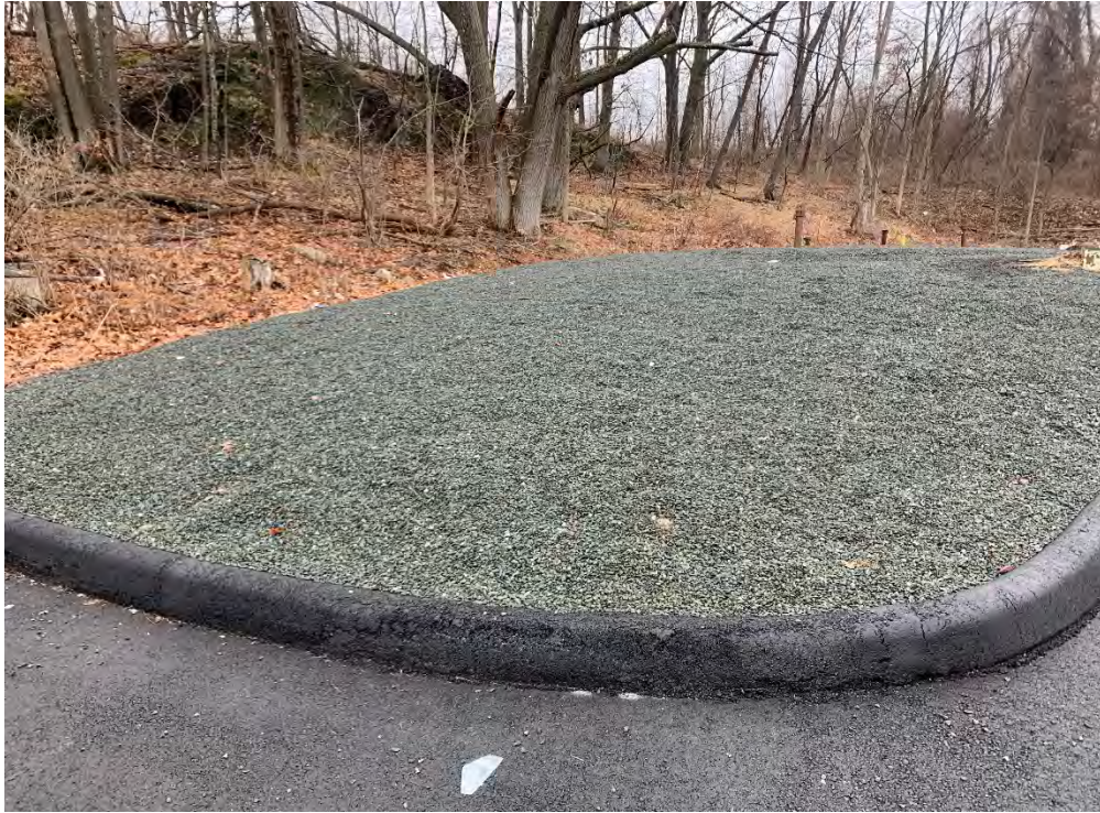
Photo 9: Stone cap condition (facing southeast).
