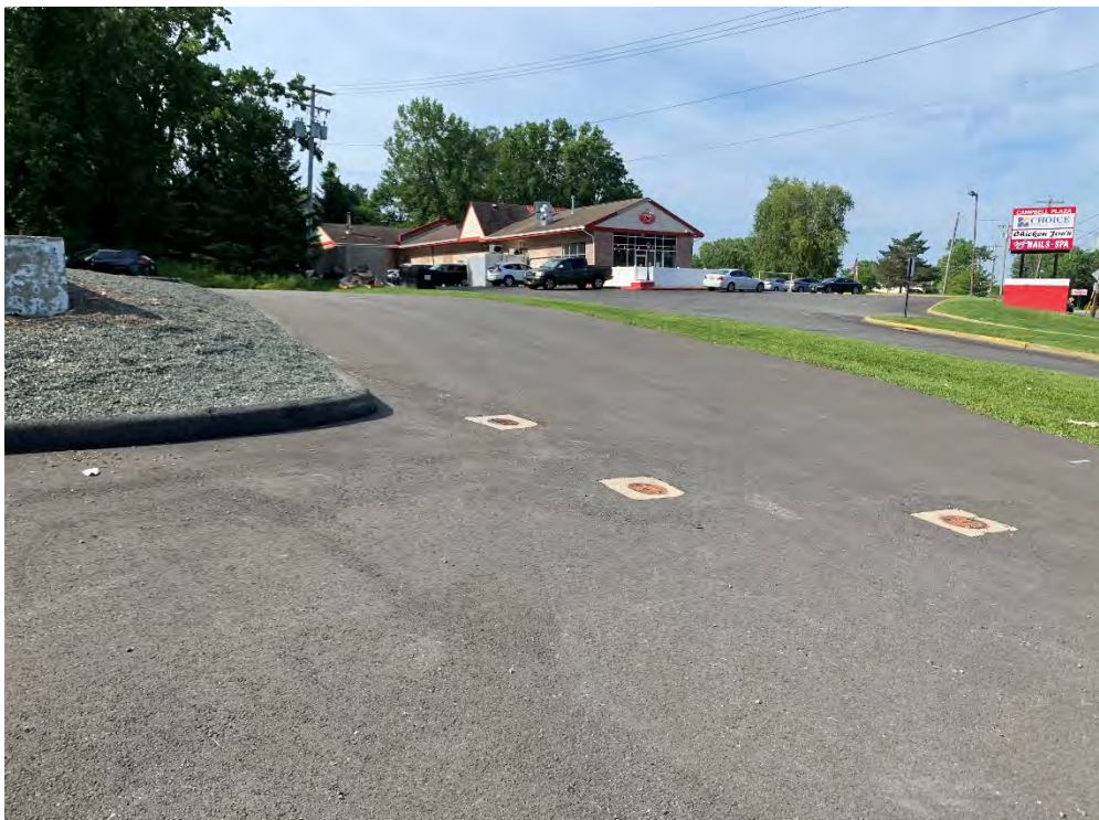
Photo 14: Asphalt cap condition (facing southwest).
