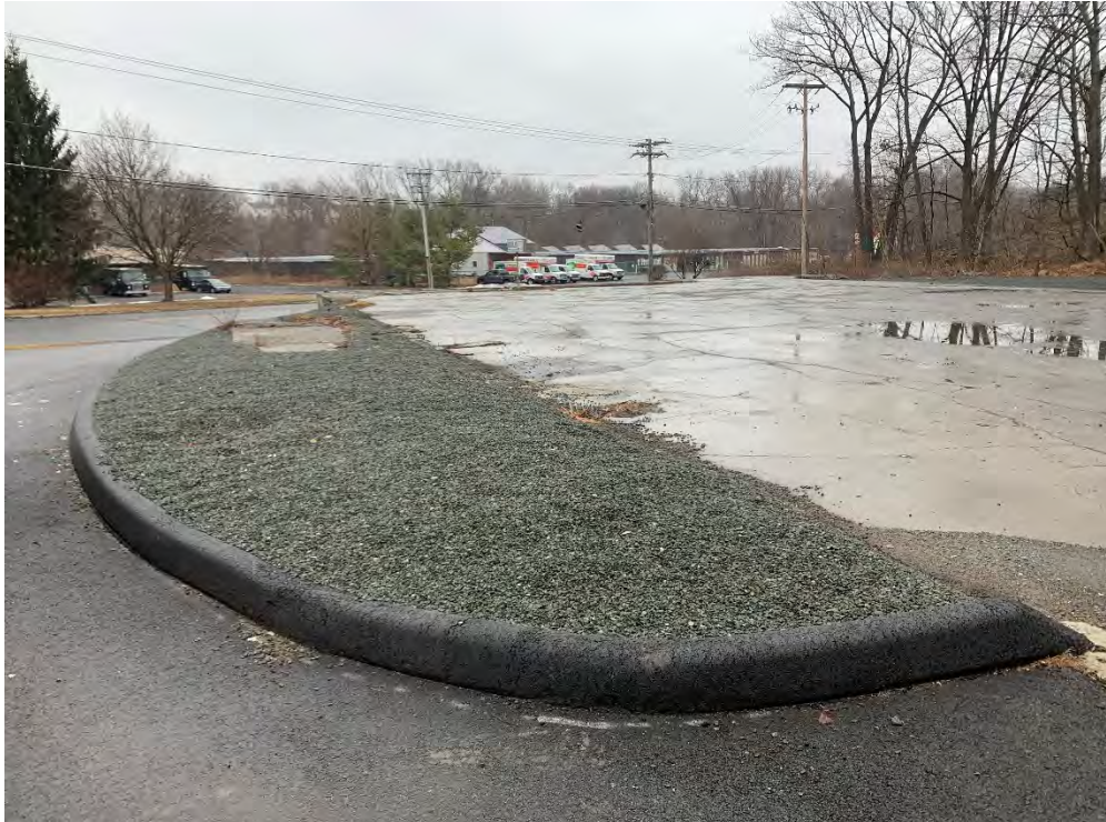
Photo 7: Concrete and stone cap condition (facing northeast).
