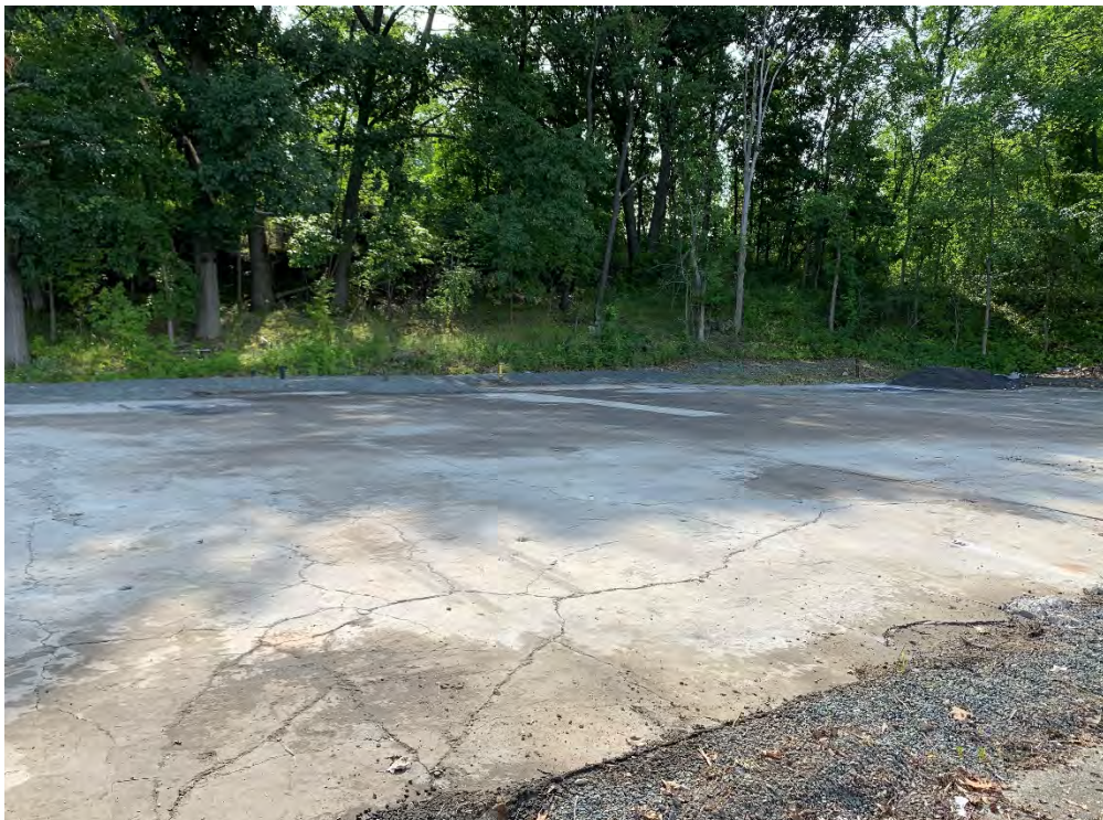
Photo 8: Concrete cap condition (facing southeast).
