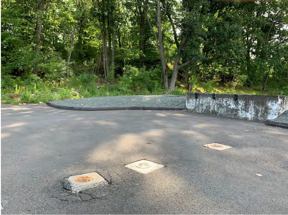
Photo 11: Former building foundation, stone, and asphalt cap condition (facing southeast).
