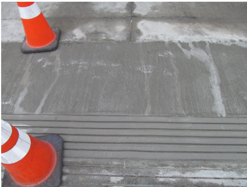
Photos of Concrete Apron Area – After Concrete Replacement
