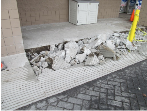
Photos of Concrete Apron Area – During Removal
