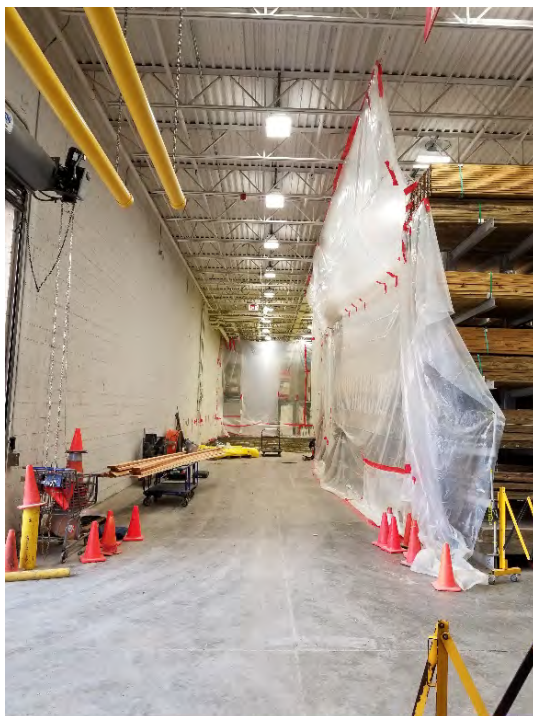
Photos of Isolated Work Areas Inside Building – During Slab Removal & Replacement
