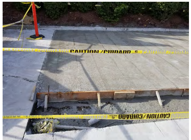
Photos of Concrete Slab Replacement
