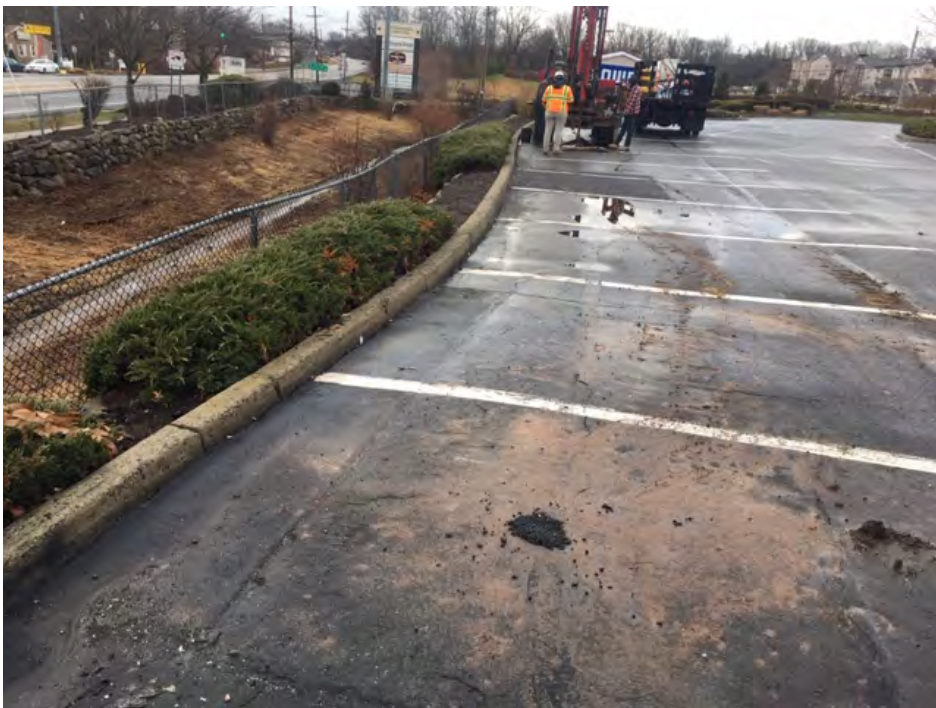
Geotechnical Borings in the Parking Lot Near the Retention Basin
