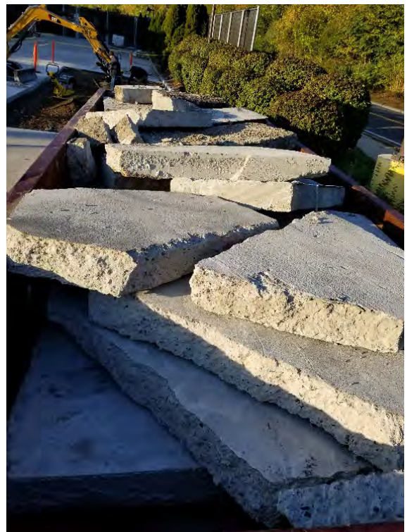
Photos of Concrete Slab Areas – During Removal
