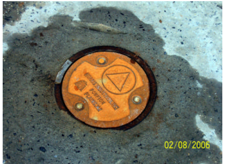
02/08/2006 - Sealed Monitoring Well
