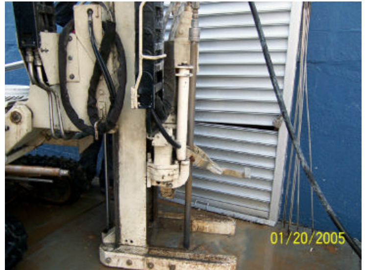
01/20/2006 - RegenOx Injection at Location # 8
