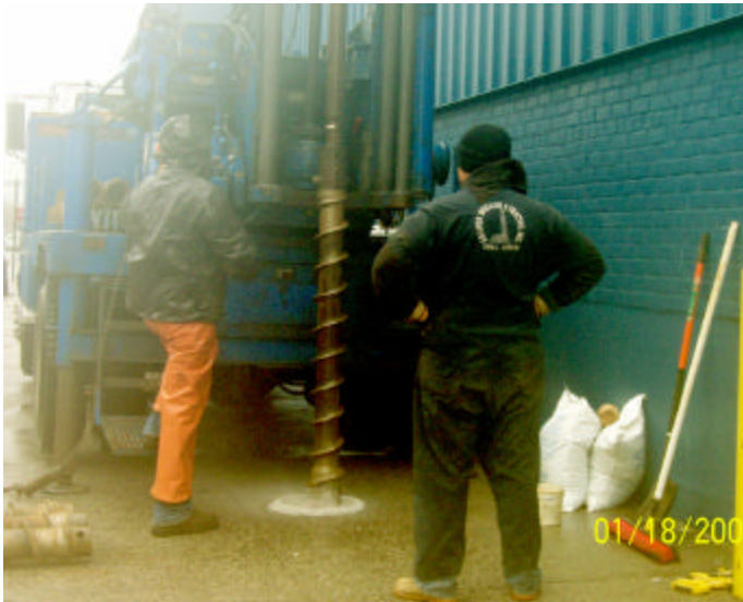
01/18/2006 - Permanent Down Gradient Monitoring Well Installation Boring
