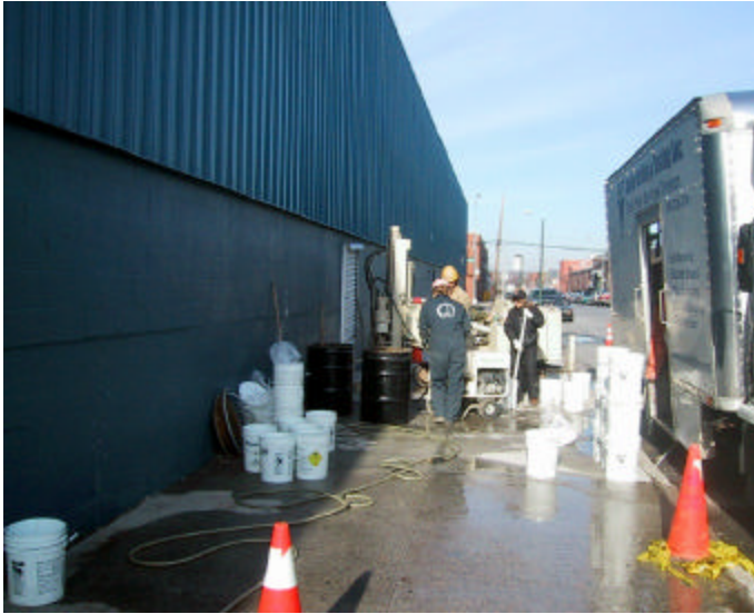
01/20/2006 - RegenOx Injection at Location # 3
