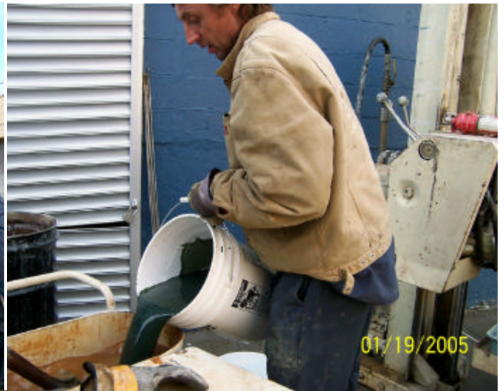
01/19/2006 - Adding Activator to the Mixture
