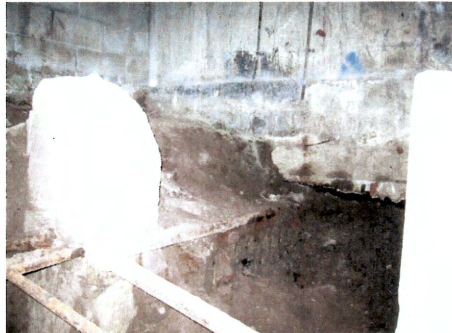
EXCAVATION BY LEAK SOURCE
