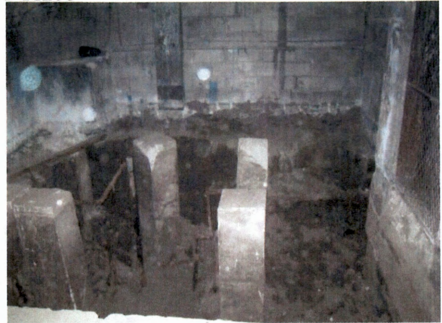
EXCAVATION TO TOP OF TANKS
