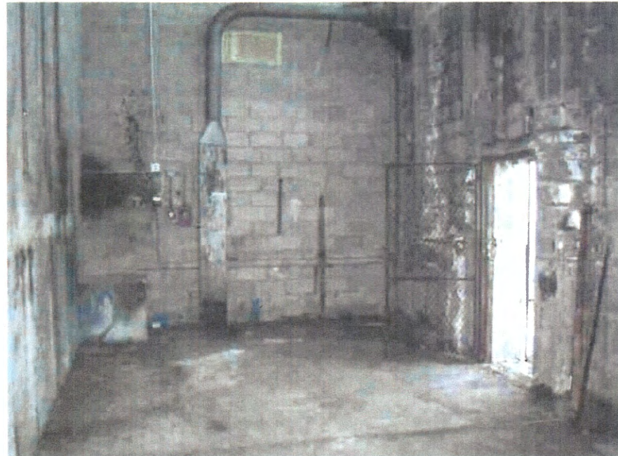
PAINT STORAGE ROOM
