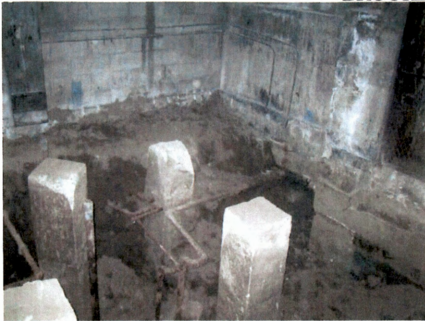
EXCAVATION REVEALING PIPES
