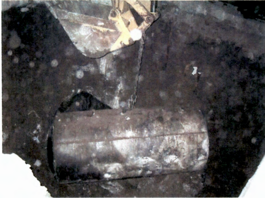
SOUTHERN TANK BEING REMOVED
