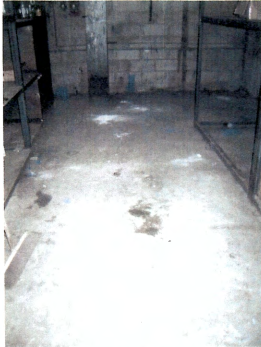
PAINT STORAGE ROOM
