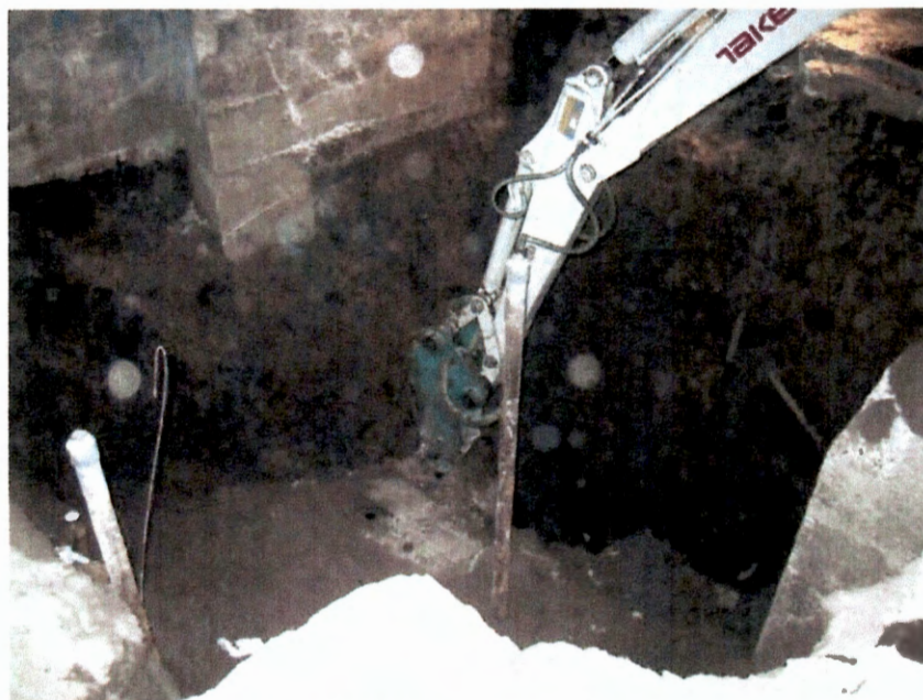
BREAKING CONCRETE AROUND TANK
