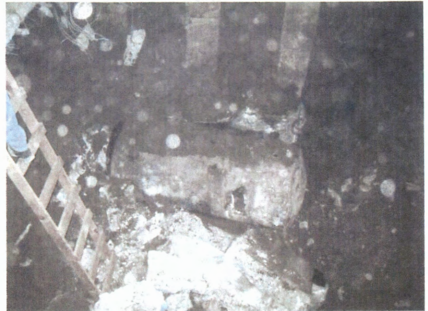
NORTHERN TANK EXPOSED
