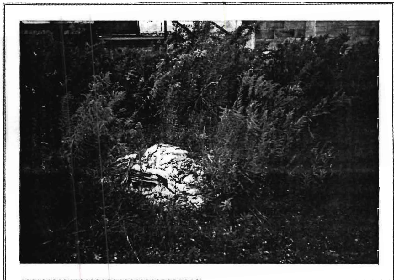
Photo #22: Pile of demolition debris potentially containing ACMs located near former scale house building.
