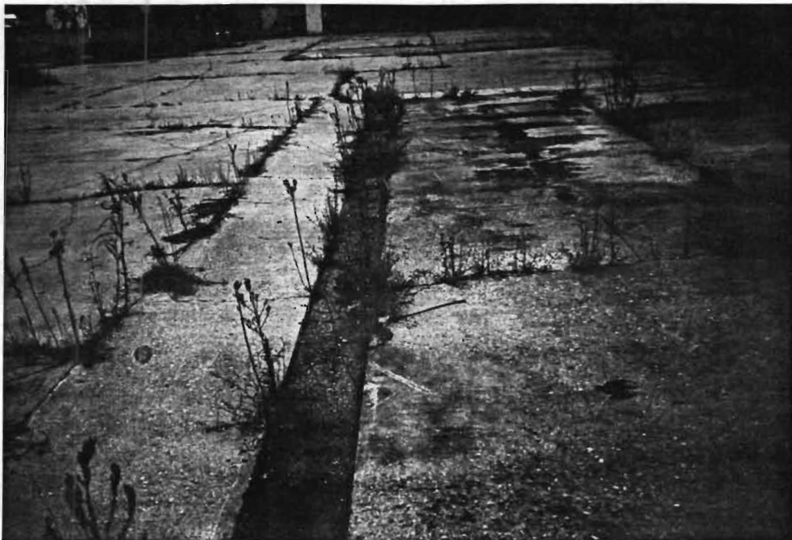
Photo #25: Trench drain filled with sediment observed in fenced yard located along south side of warehouse building.
