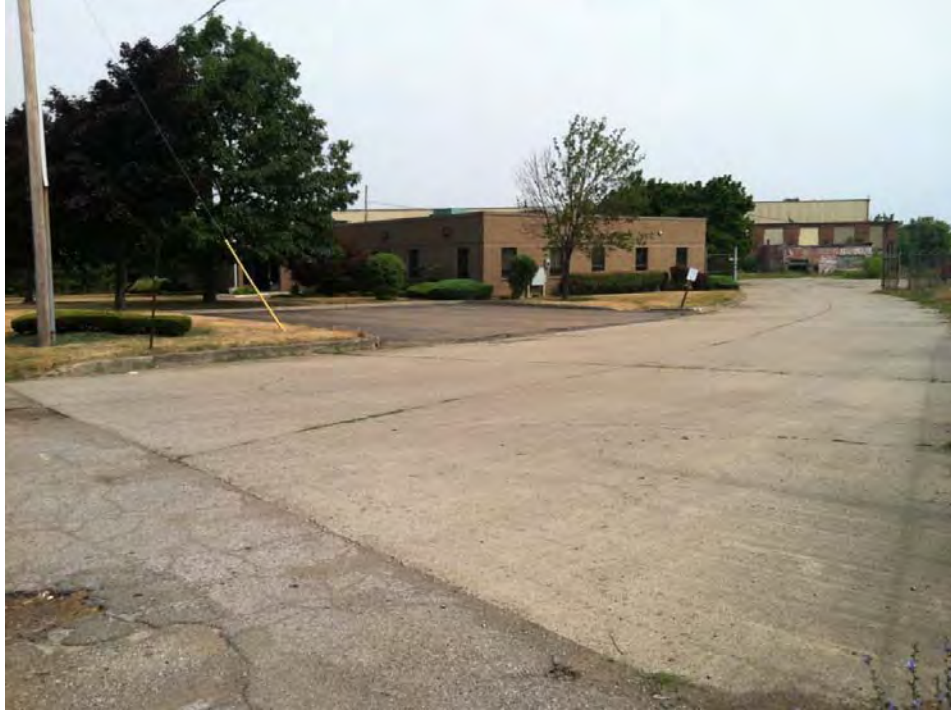
Photograph 5: 79.16-2-4 property facing northeast from South Roberts Road
