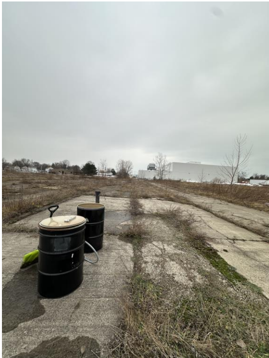
View of AL-1 and AL-2 facing West
