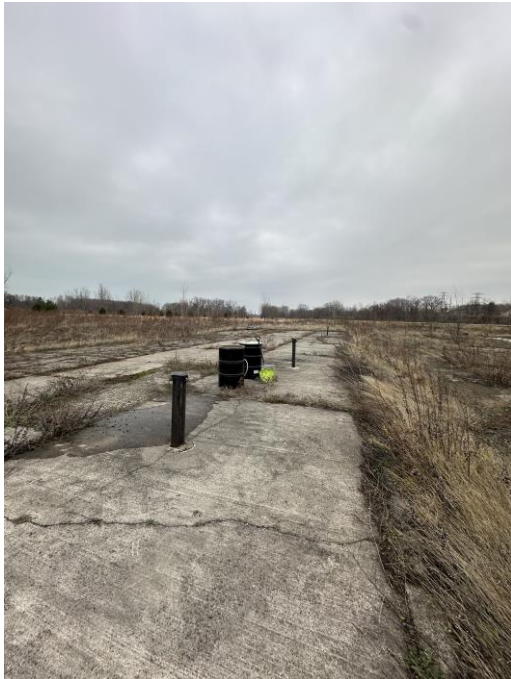
View of AL-1 and AL-2 facing East
