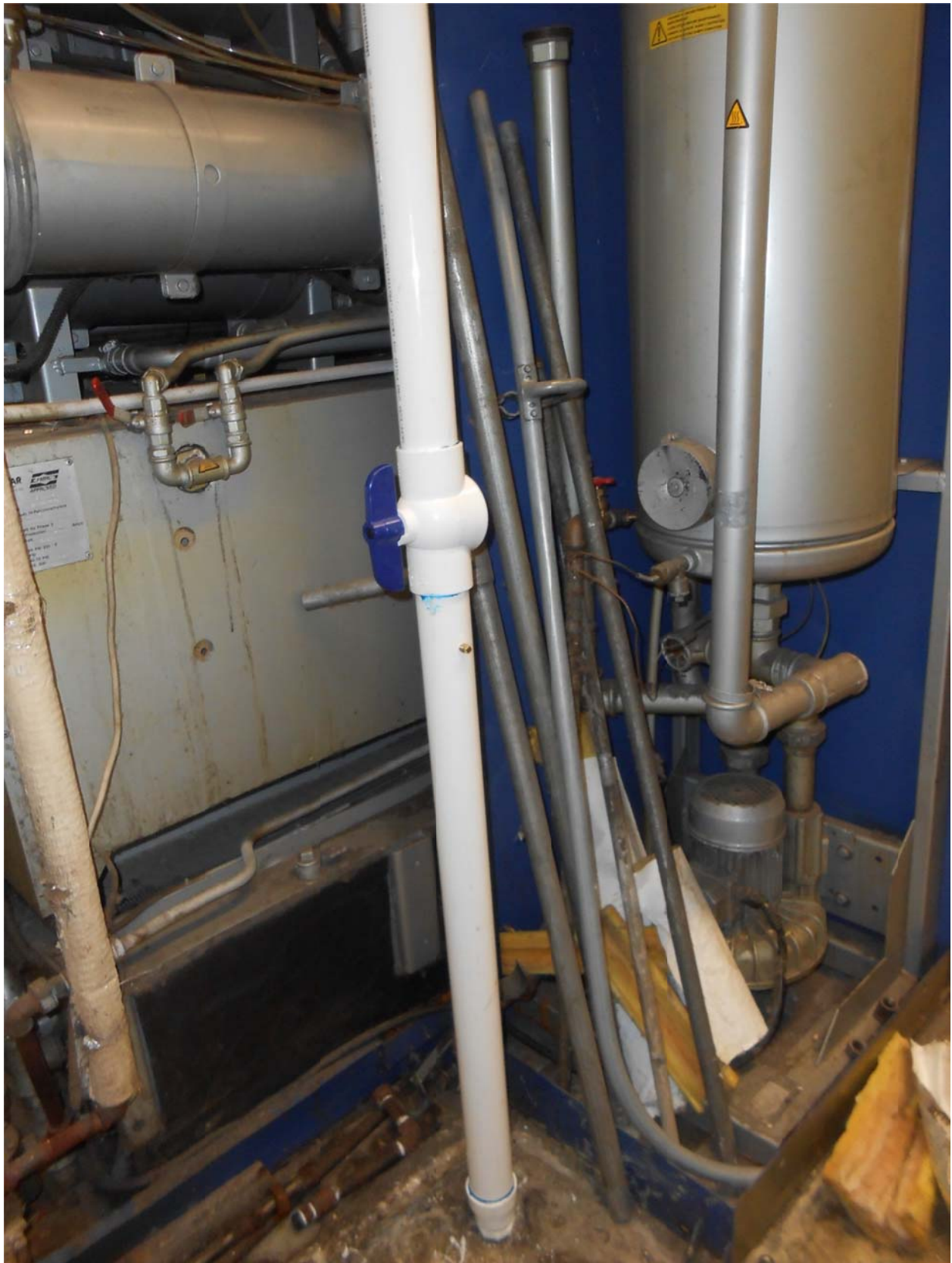
P18. Complete schedule 40 2-inch PVC vertical shaft at XP2 with valve showing adapter on base of PVC. 4/10/15
