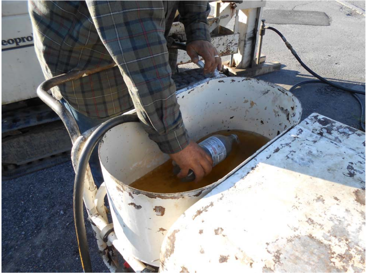
P43. Placing the measured 0.75 liter of inoculum into the 7.5 gallons of deoxygenated water in the hopper of the high pressure GS2000 pump. October 8, 2015
