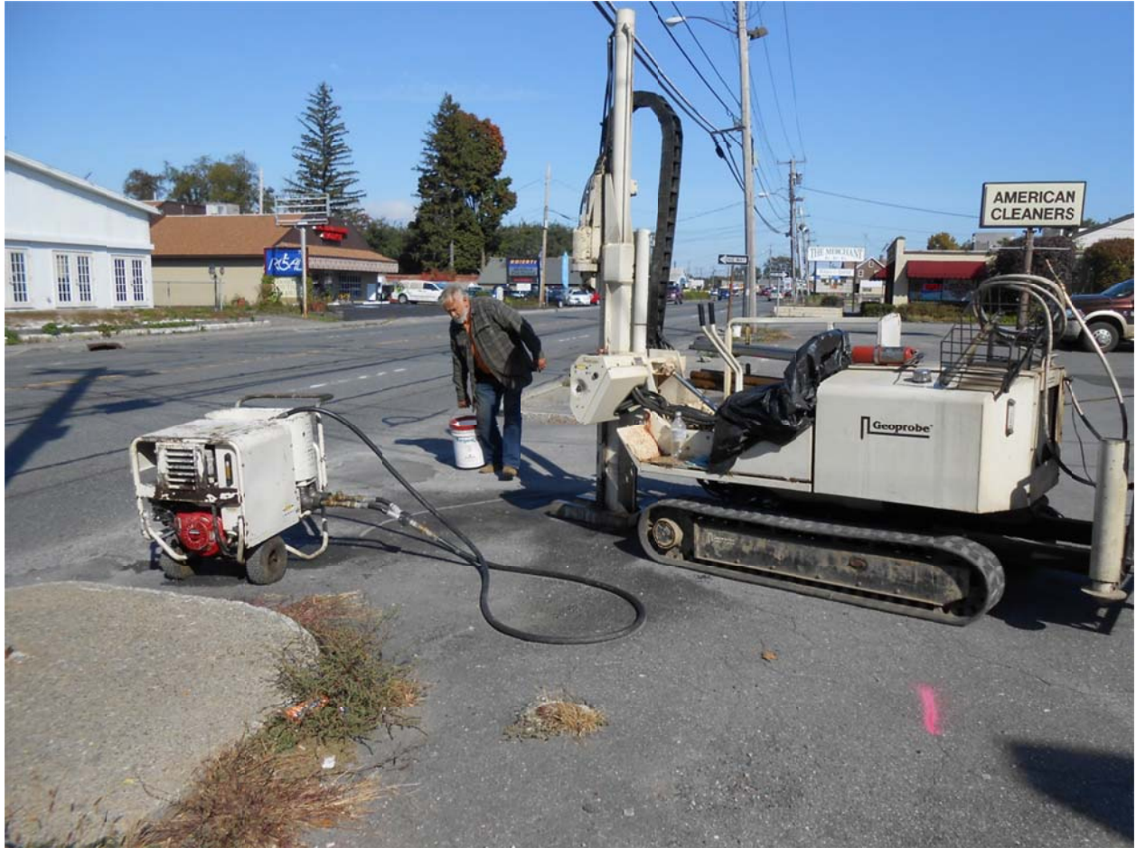
P46. Boring hole in the foreground is filled with sand and bentonite. October 8, 2015
