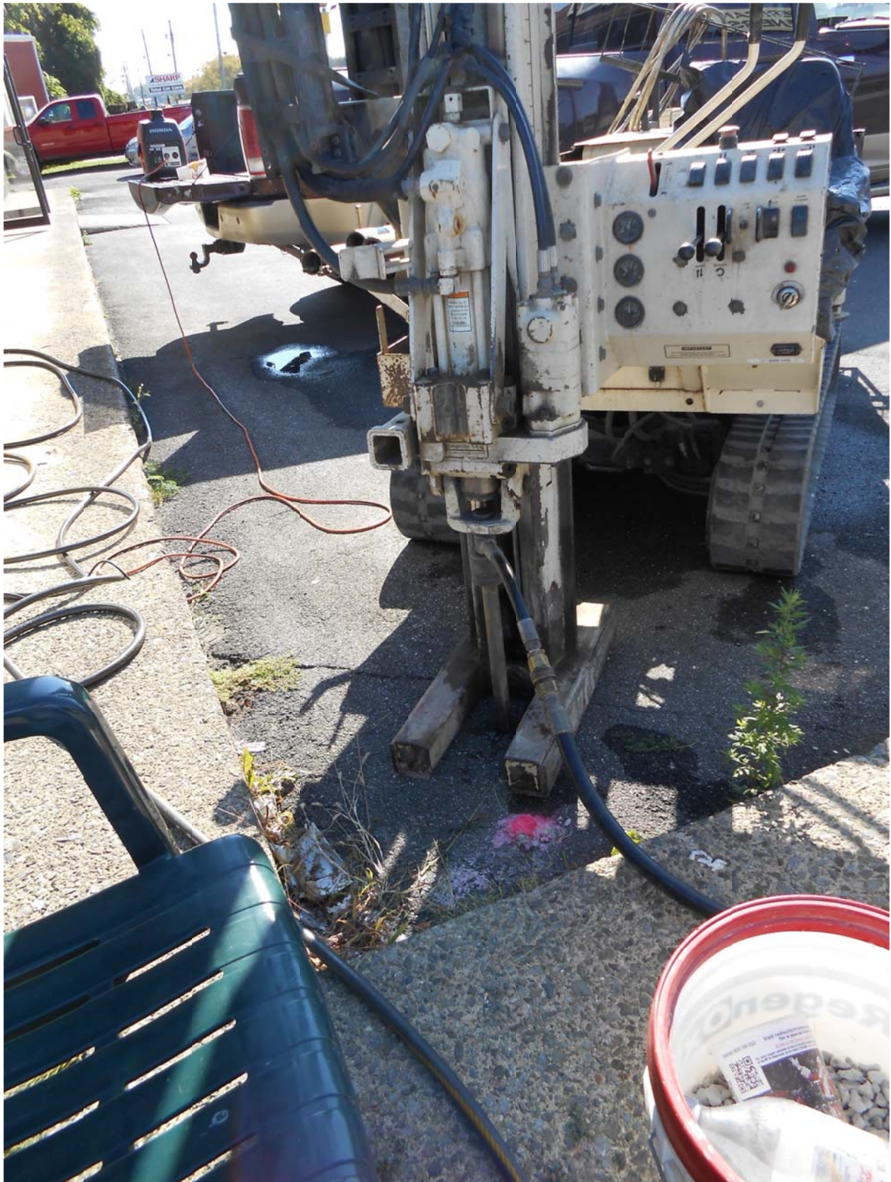
P44. Black hose from the GS2000 pump connects to the Geoprobe drill rods for injection. April 7, 2015
