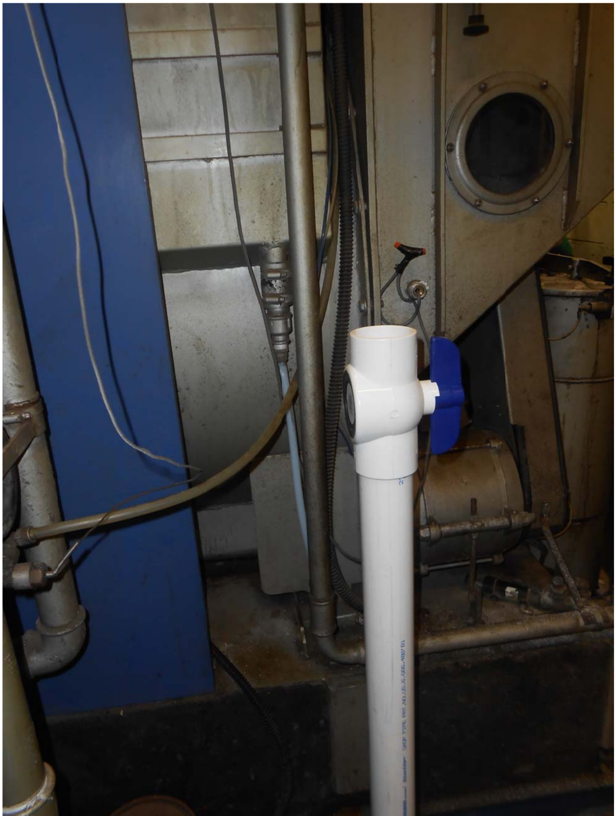
P17. 2-inch schedule 80 PVC vertical shaft installed at XP1 with blue-handled on/off valve to close shaft from atmosphere during vapor testing with Summa Canister or Photoionization Detector. 4/10/15
