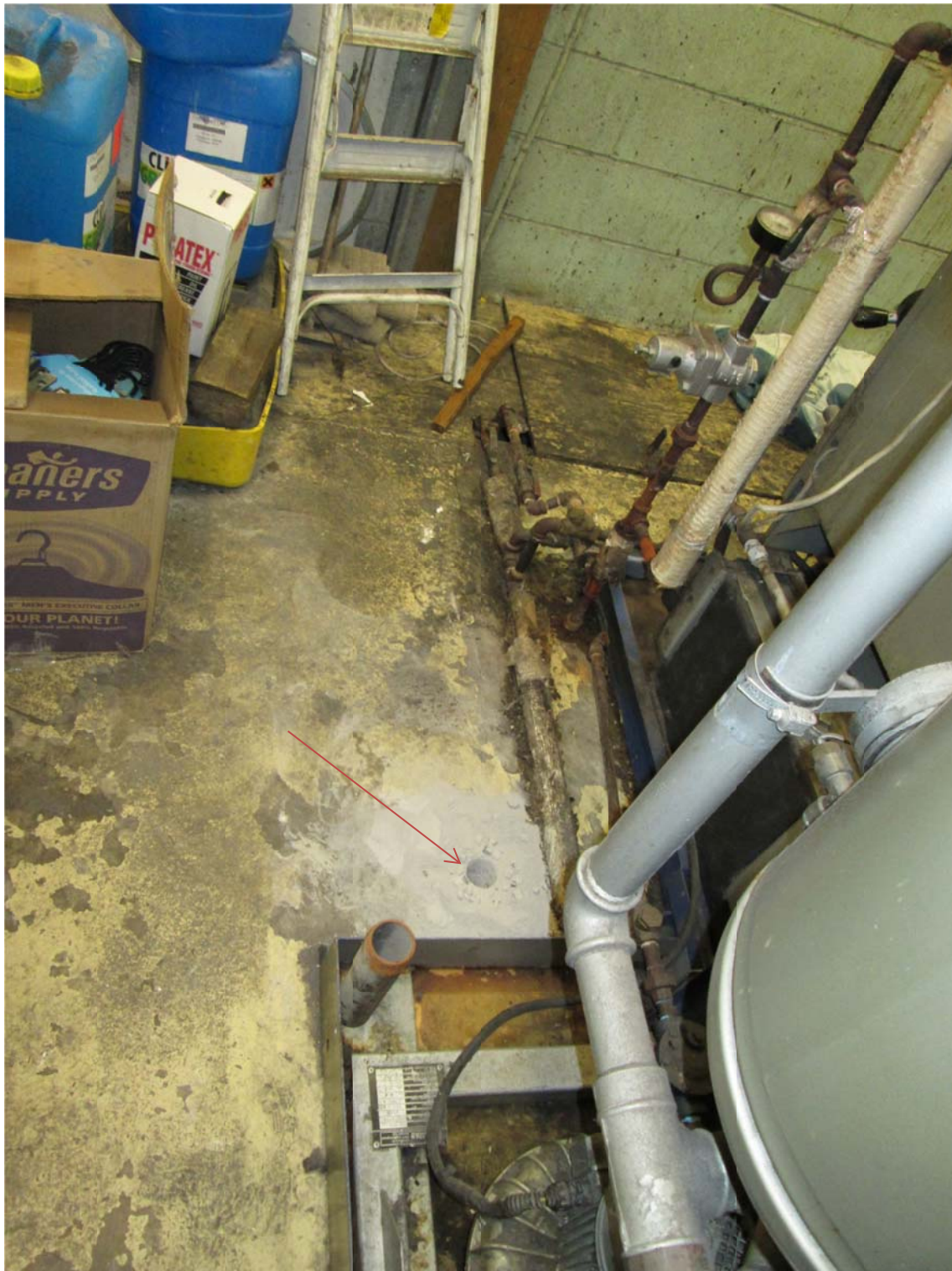
P8. Hole for XP1 through slab. 3/25/13
