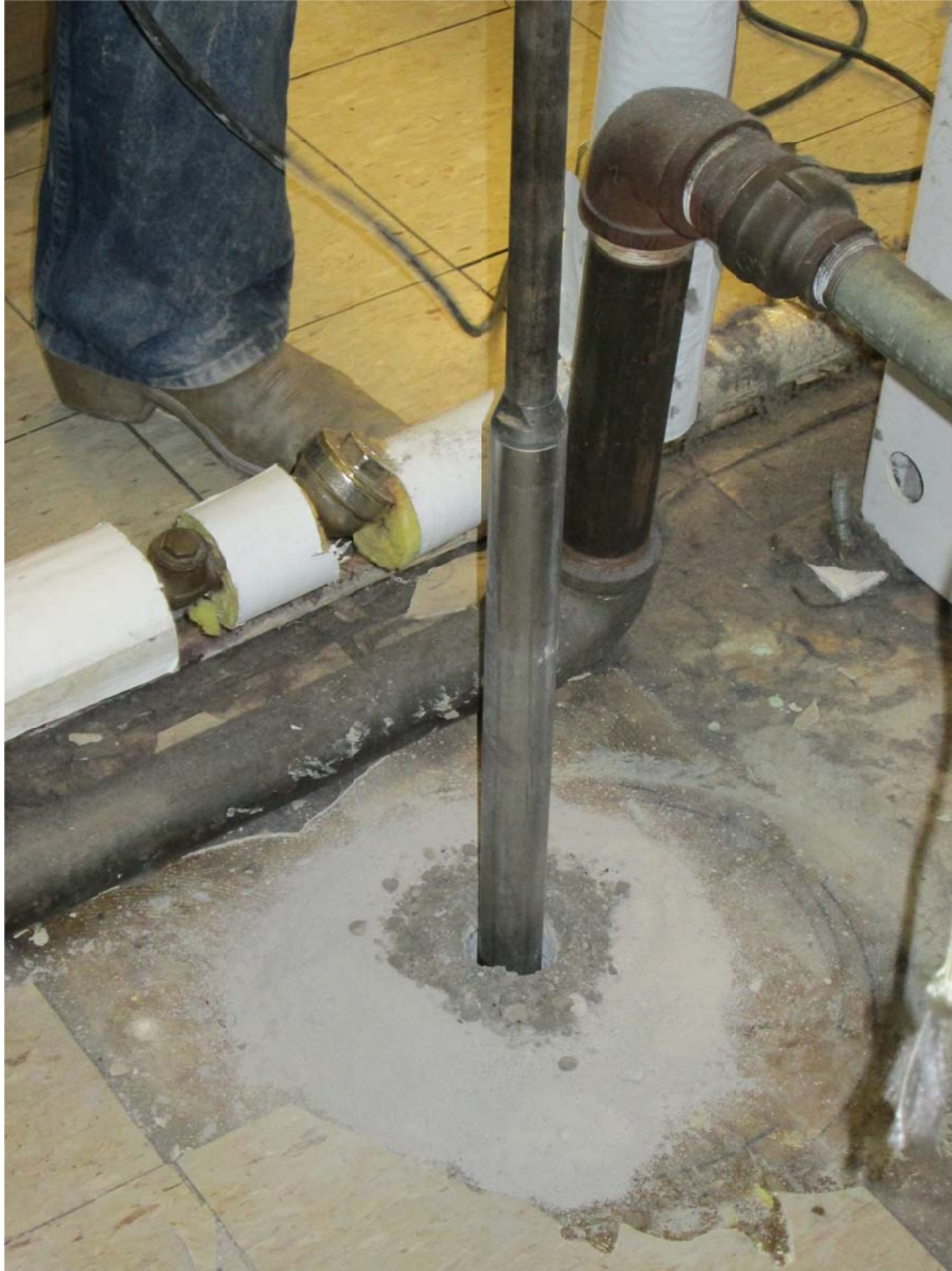
P2. Close-up of drill bit through the slab. 3/25/13
