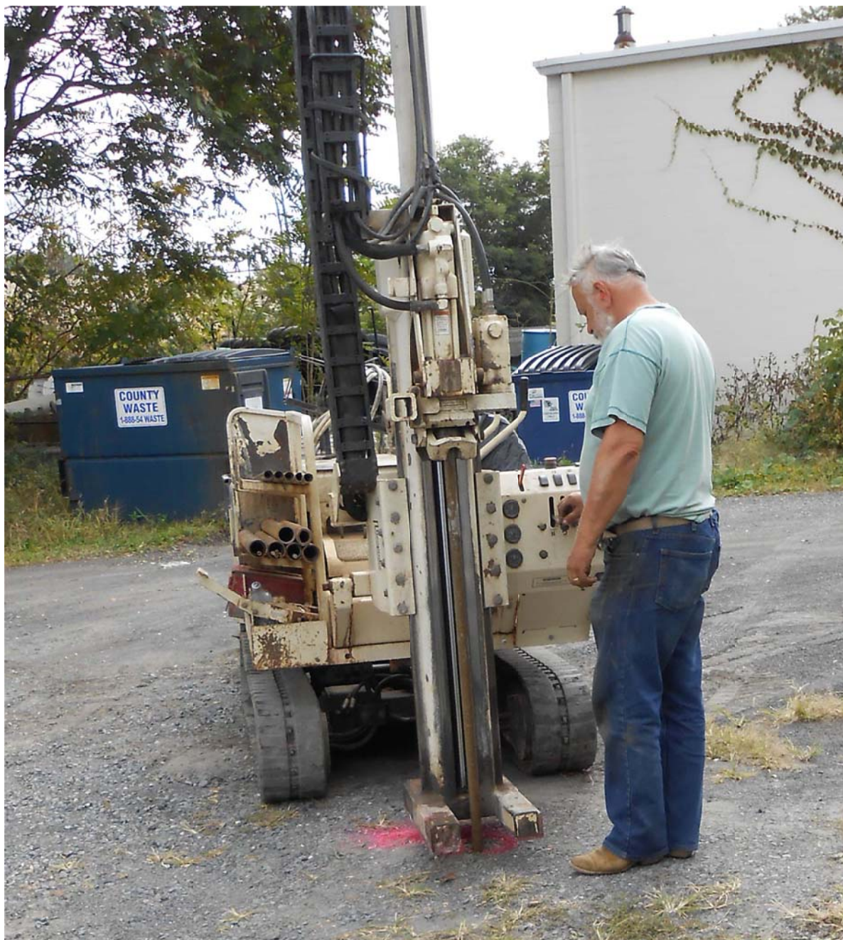
P36. Drilling the borehole for injection of inoculum into MIP3 with Geoprobe. October 7, 2015.
