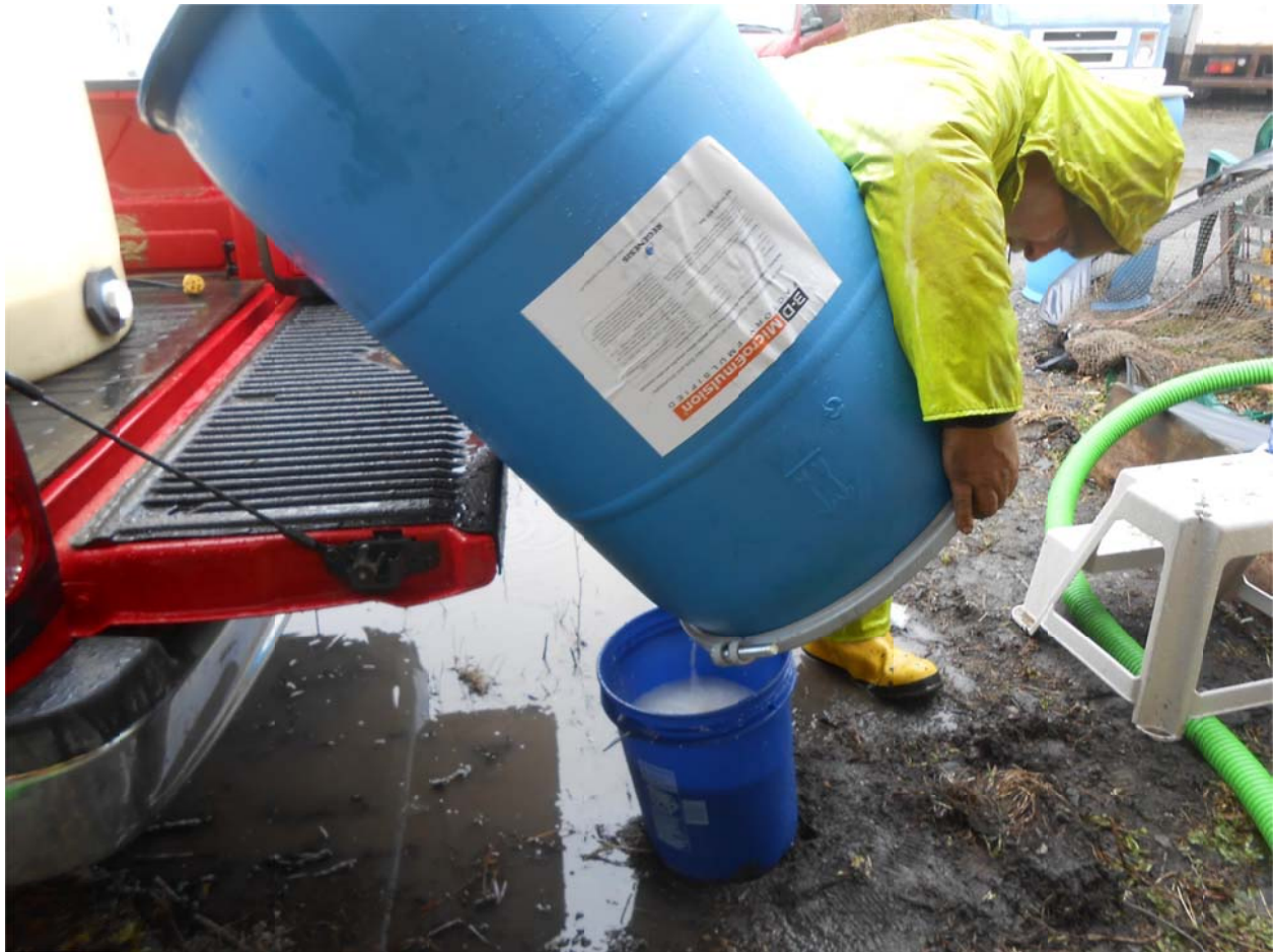
P34. The final drum of 3-D MicroEmulsion was emptied into a bucket and placed in the black mixing tank. 4/15
