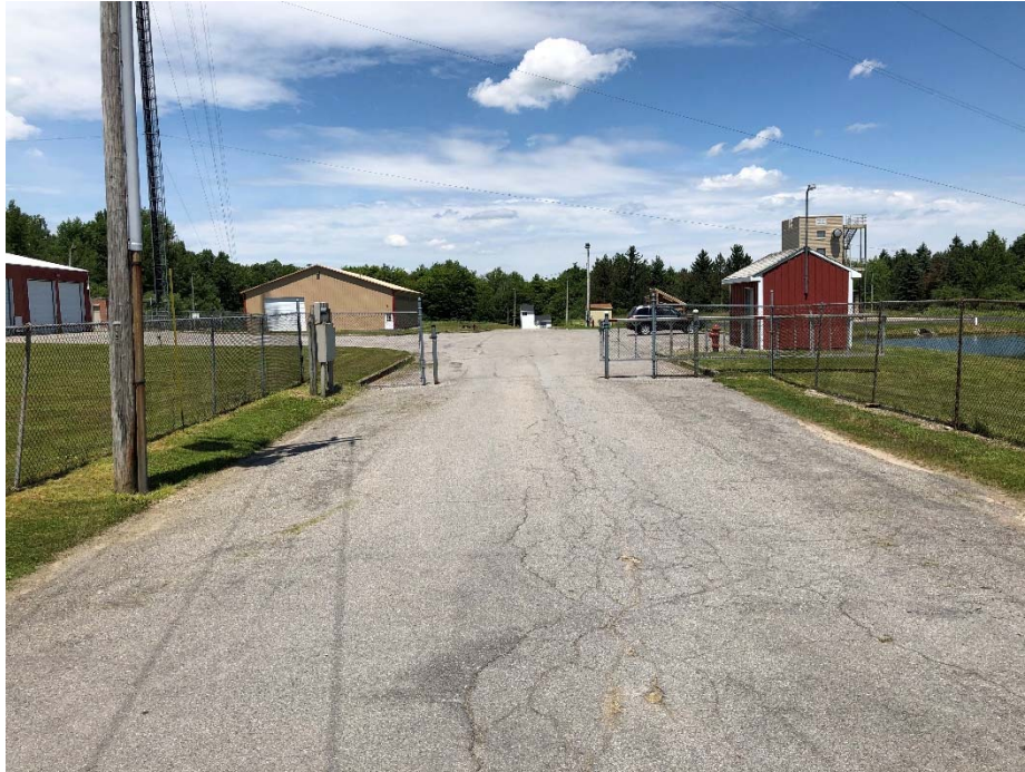
Photo 1: Main entrance to site (looking north).
