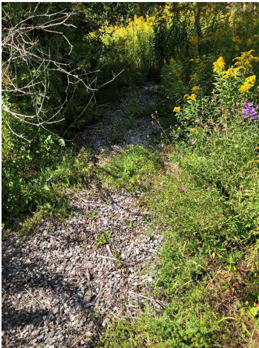
Photo 6: Gravel Drainage Area at East End of North Permeable Reactive Wall (looking north).
