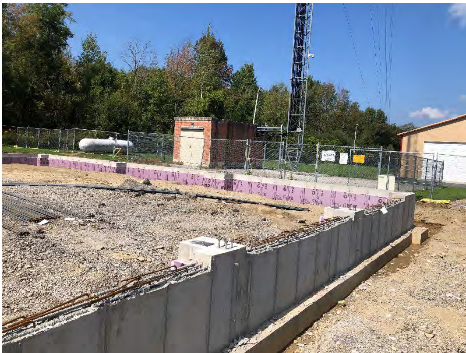
Photo 2: New building addition foundation construction (looking northwest).
