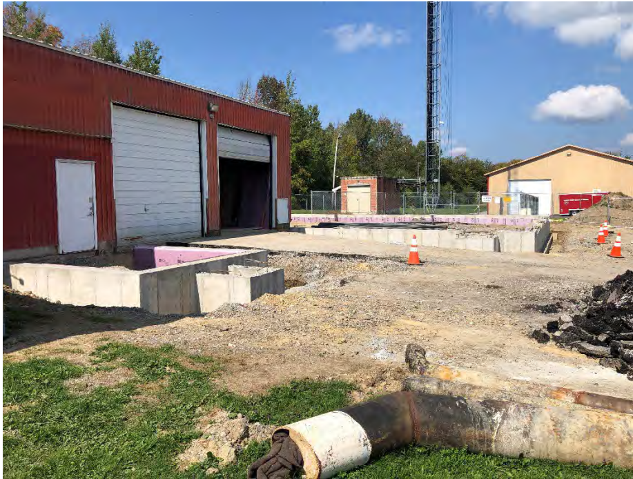
Photo 3: New vestibule and building addition construction (looking northwest).
