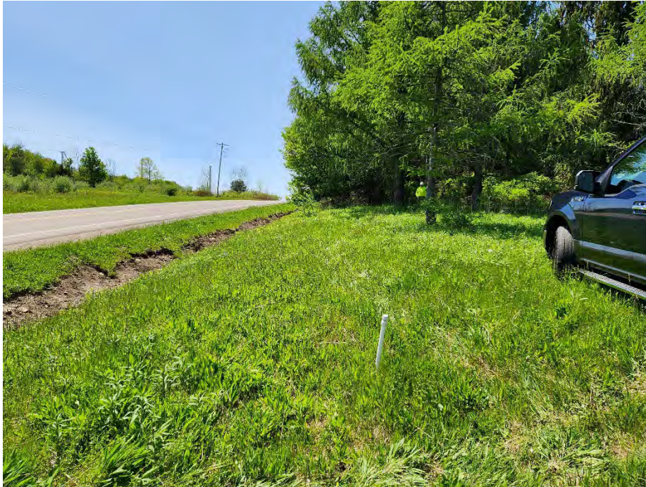
Photo 5: North Permeable Reactive Wall (looking west).
