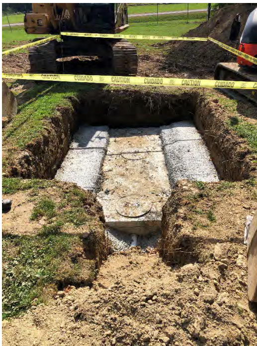
Photo 4: Newly installed septic tank (looking south).
