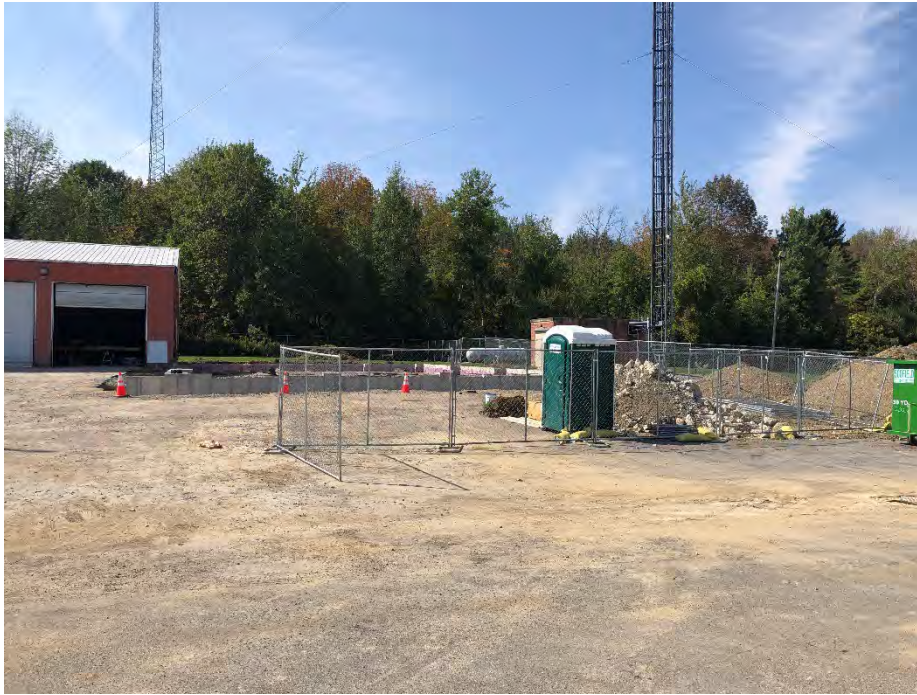
Photo 1: View of new building foundation construction area (looking west).
