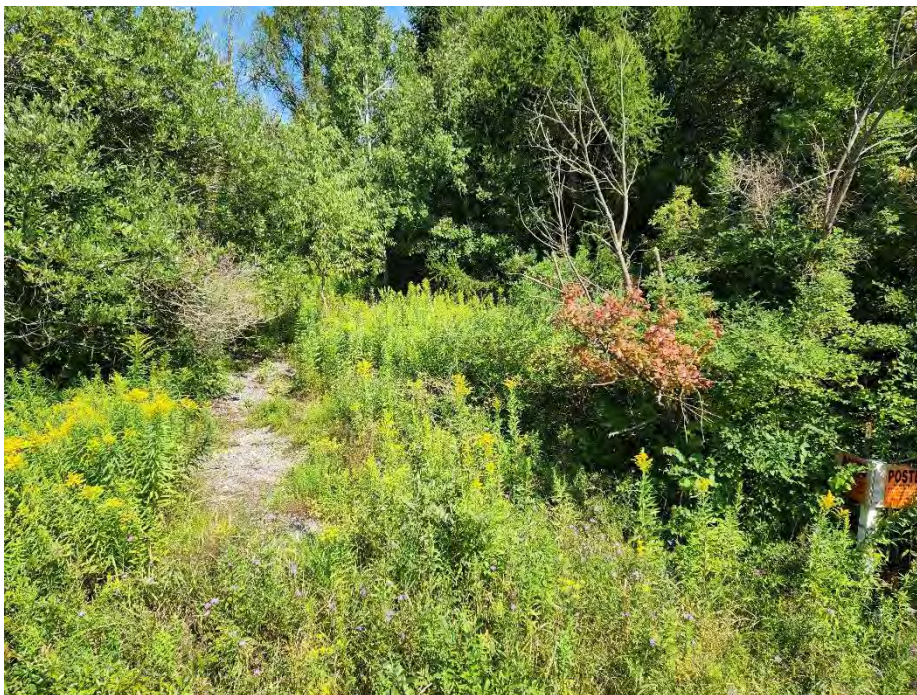
Photo 6: Gravel Drainage Area at East End of North Permeable Reactive Wall (looking north).
