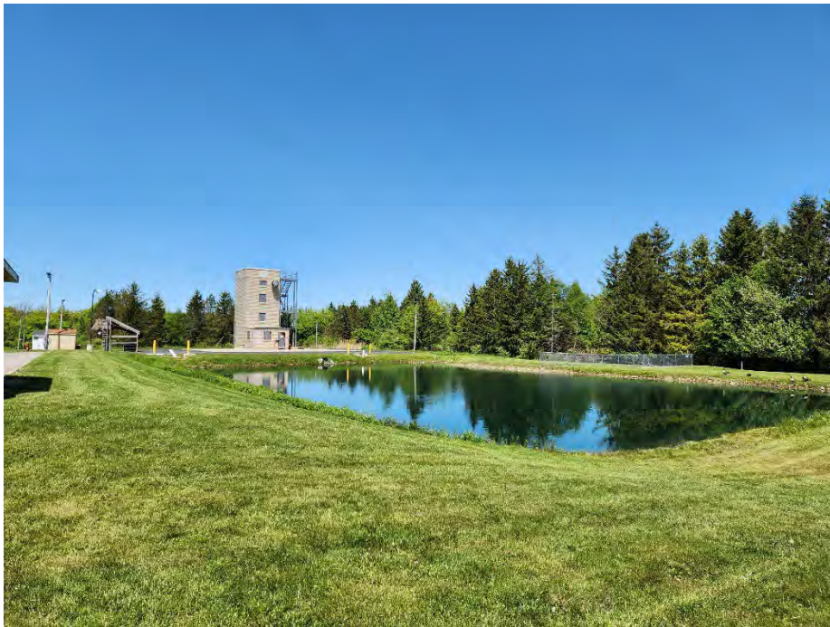
Photo 2: General view of Front Pond and current Fire Training Facility (looking northeast).
