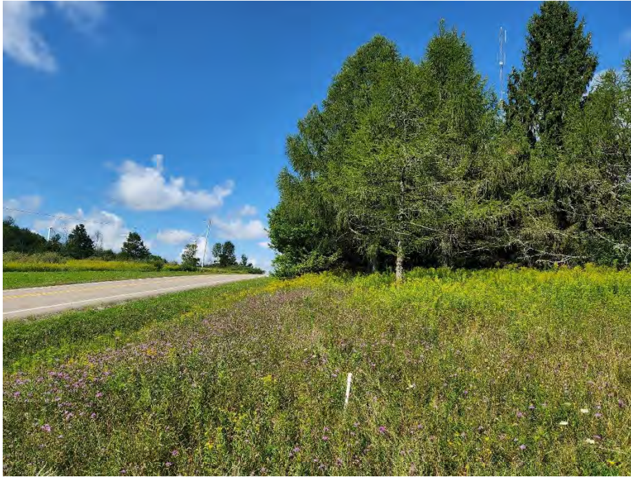
Photo 5: North Permeable Reactive Wall (looking west).
