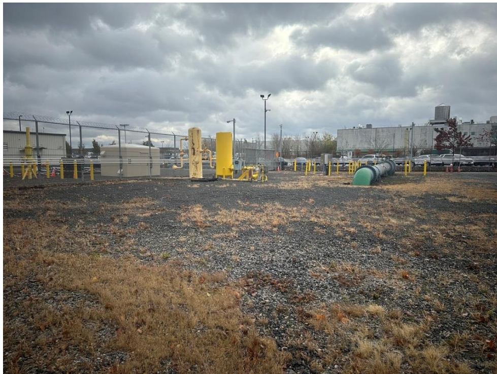
Photo 6: Gravel Cover on Con Edison Property (Facing Southeast)
