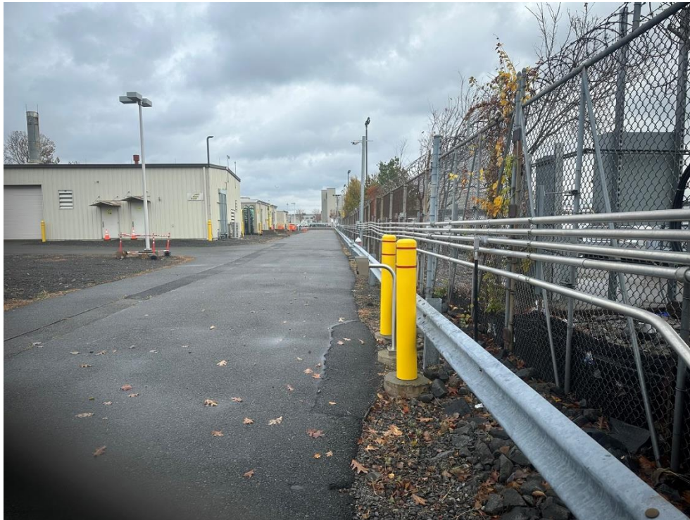
Photo 4: Iroquois Property Roadway (Facing East)
