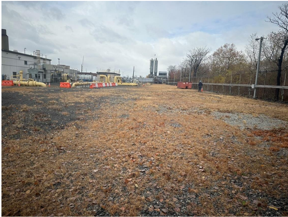
Photo 5: Gravel Cover on Con Edison Property (Facing Southwest)
