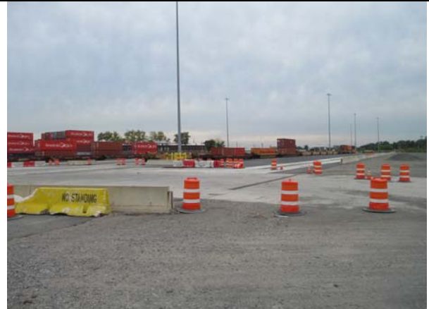
Photo 2: Concrete and crushed stone cover in Site 1 taken facing southeast.
