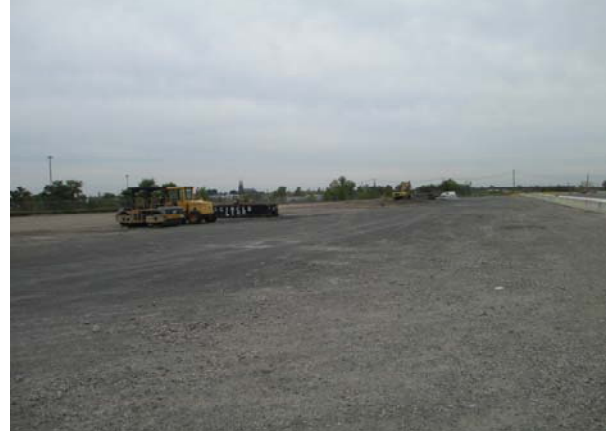
Photo 4: Crushed stone cover and container storage in Site 1 taken facing northwest.
