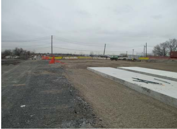
Photo 1: Railroad track excavation work in Site 1 taken facing northeast.
