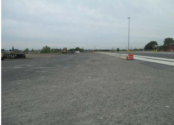
Photo 3: Crushed stone cover and newly installed railroad track taken facing north.
