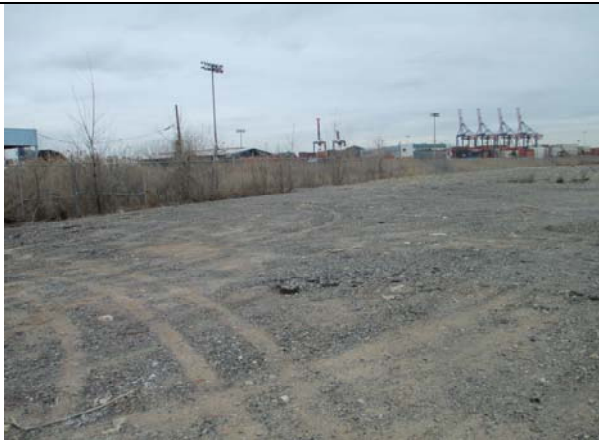
Photo 3: Crushed stone cover in Site 1 taken facing northwest.
