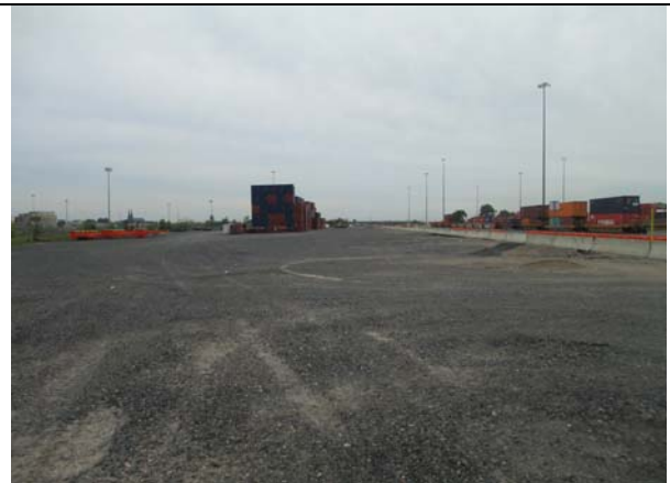
Photo 6: Crushed stone cover and container storage in Site 1 taken facing north.
