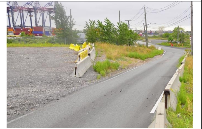
Photo 6: View of asphalt roadway in Site 1 taken facing west-northwest.
