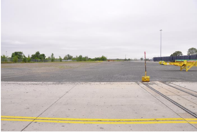
Photo 1: View of environmental cover (concrete and gravel) in Site 1 taken facing north.
