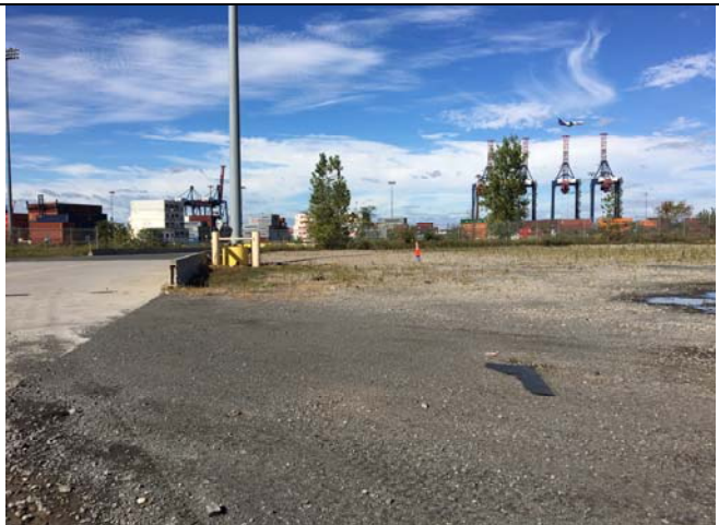
Photo 6: Environmental cover (gravel) in Site 1 taken facing west.
