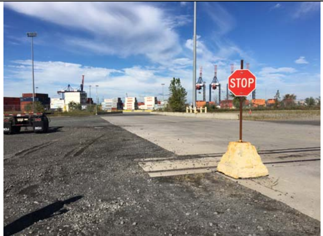
Photo 4: View of environmental cover (gravel and concrete) in Site 1 taken facing west.
