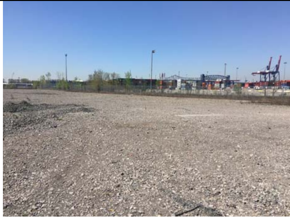
Photo 1: View of environmental cover (gravel) in Site 1 taken facing west.
