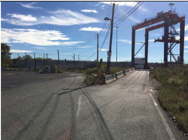
Photo 5: View of environmental cover (asphalt) in Site 1 taken facing southeast.
