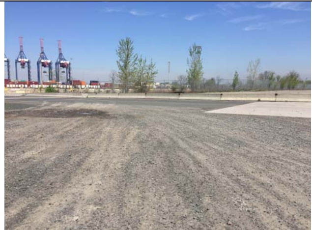
Photo 4: View of environmental cover (gravel/concrete/asphalt) in Site 1 taken facing northwest.
