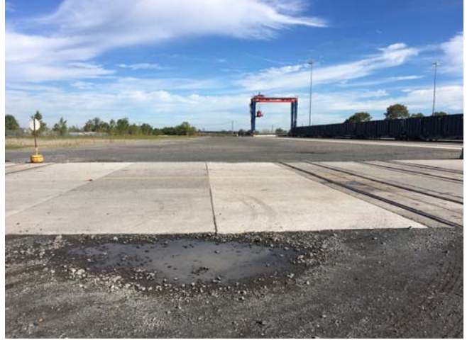
Photo 2: View of environmental cover (concrete and gravel) in Site 1 taken facing north.
