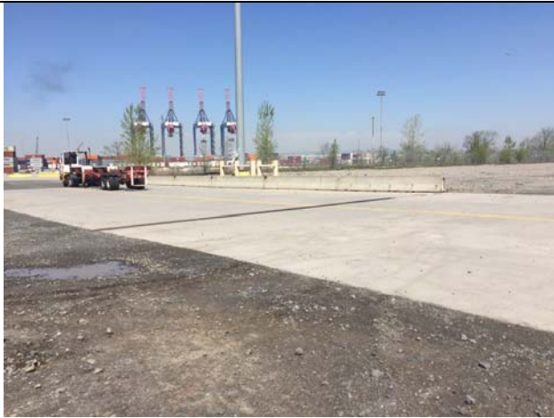
Photo 3: View of environmental cover (concrete) in Site 1 taken facing northwest.
