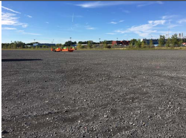
Photo 3: View of environmental cover (gravel) in Site 1 taken facing west.
