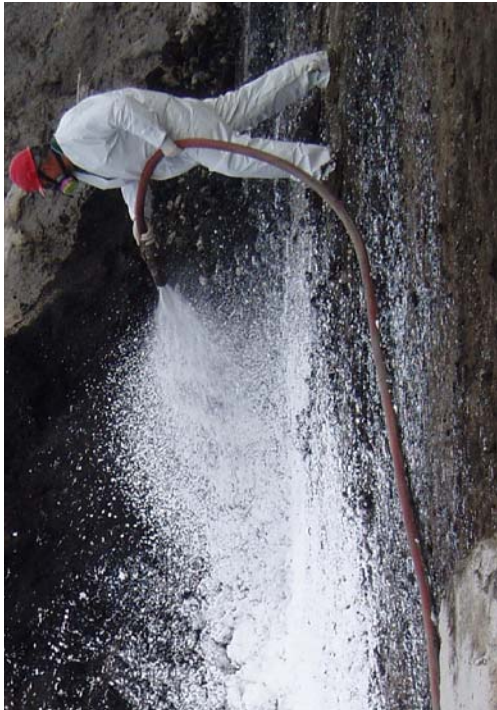
Figure 6 Odor Suppressant Foam Application
