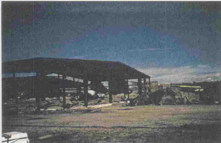
Hydroponics plant under construction on Truscon Site
