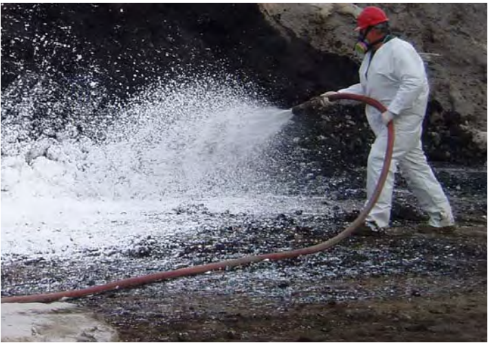
Figure 6 Odor Suppressant Foam Application
