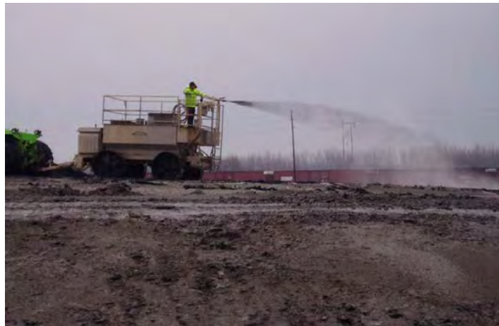
Figure 7 Odor Suppressant Posi-Shell® Application
