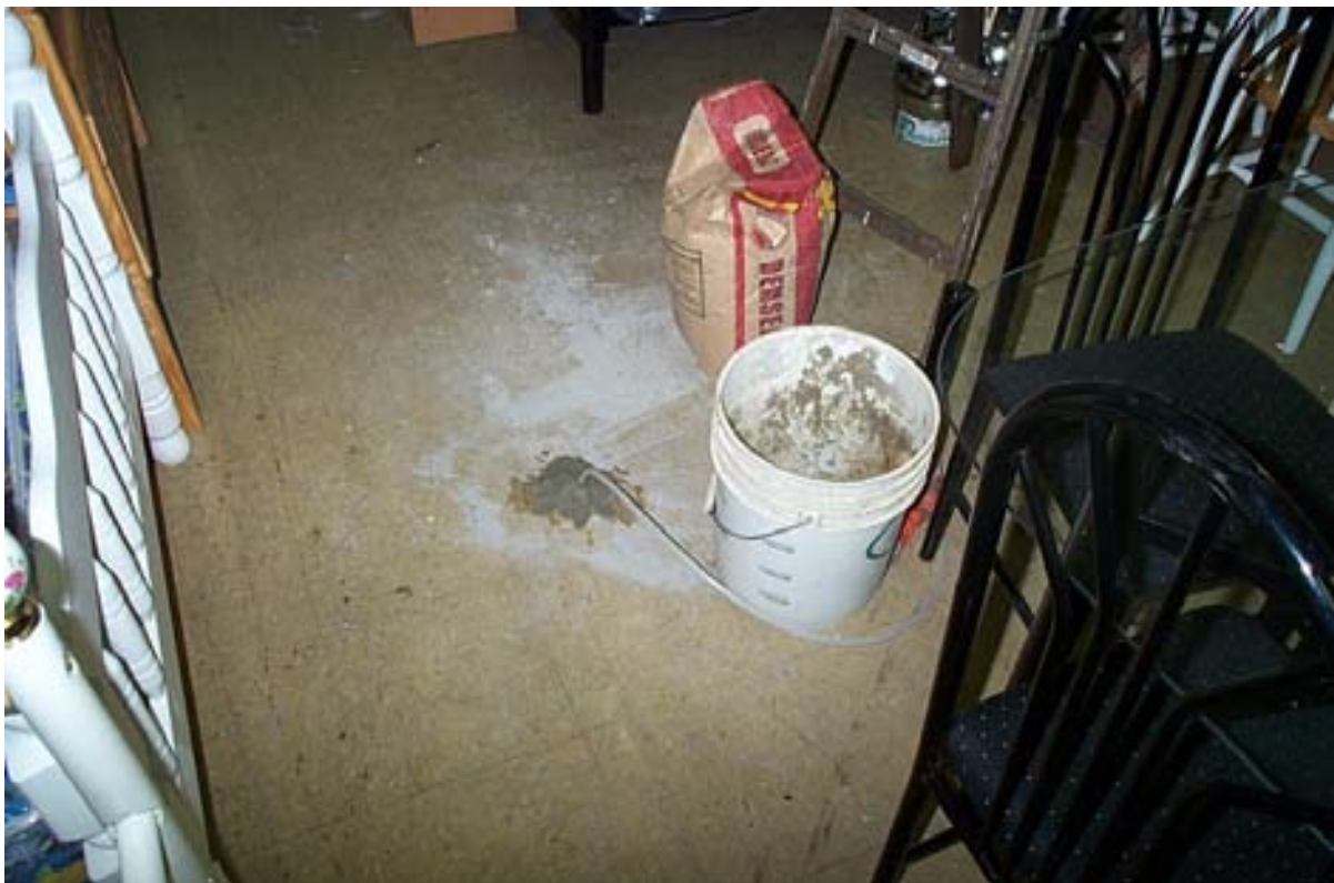
Example of monitoring point after installation.
