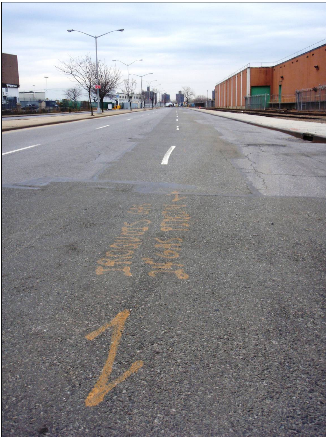
Photograph No. 3 – Southern Portion of Perimeter Site, Food Center Drive (looking northeast) (Note: Iroquois Gas Pipeline mark-out and saw-cut asphalt associated with pipeline installation)
