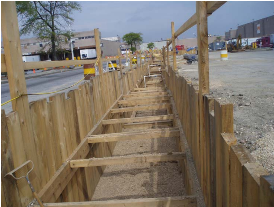
Photograph No. 2 – Excavation of trench with shoring and pipe bedding in place, looking north.
