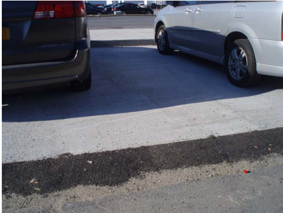
Photograph No. 5 – Asphalt patch along concrete installation.
