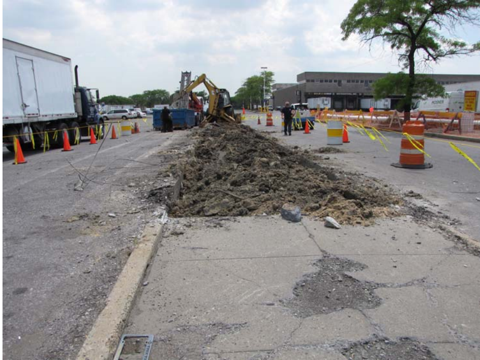
Photograph No. 1 – Removal of surface concrete from sidewalk/median, looking south.
