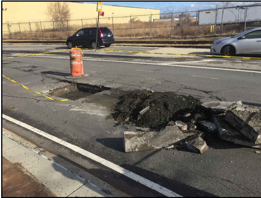
Photo 1: Facing northeast towards the southern portion of Krasdale Foods/former VCP Site F; test pit performed within Food Center Drive with excavated fill material and asphalt/concrete debris (January 2019). No MGP-related impacts noted and roadway was re-capped with asphalt.
