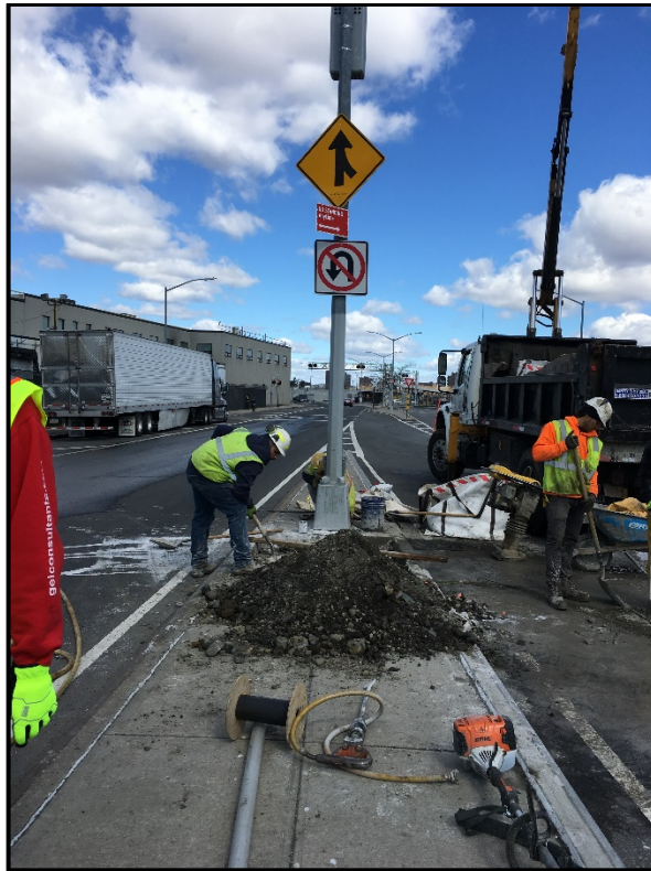
Photo 9: Facing north; excavated fill material within the median of Food Center Drive during telecommunication line installation. No evidence of MGP-related impacts were noted and the excavated fill was used as backfill in the same excavation.
