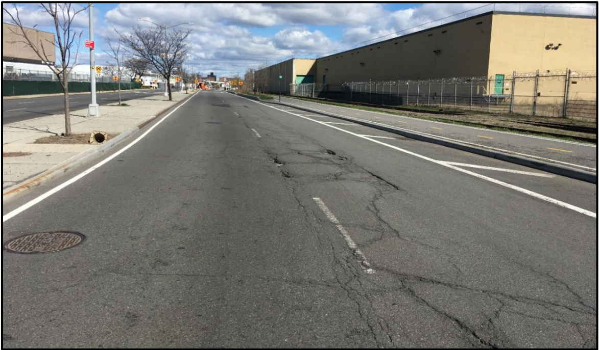
Photo 6: Facing north; FCD drive between Krasdale Foods (BCP Site 400 FCD) and the Meat Market (BCP Site 355 FCD). Minor cracking within the asphalt pavement.
