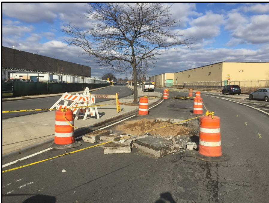
Photo 2: Facing north towards Krasdale Foods; two excavated test pits performed within Food Center Drive, backfilled with subbase material (January 2019). No MGP-related impacts were noted and the roadway was re-capped with asphalt.
