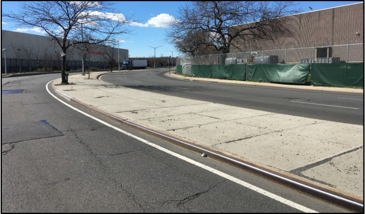
Photo 7: Facing southeast; Food Center Drive between Anheuser Busch (former VCP Site C and the Meat Market (BCP Site 355 FCD). Median in good condition. Minor cracking and evidence of asphalt patching in the roadway (from January 2019 test pits).
