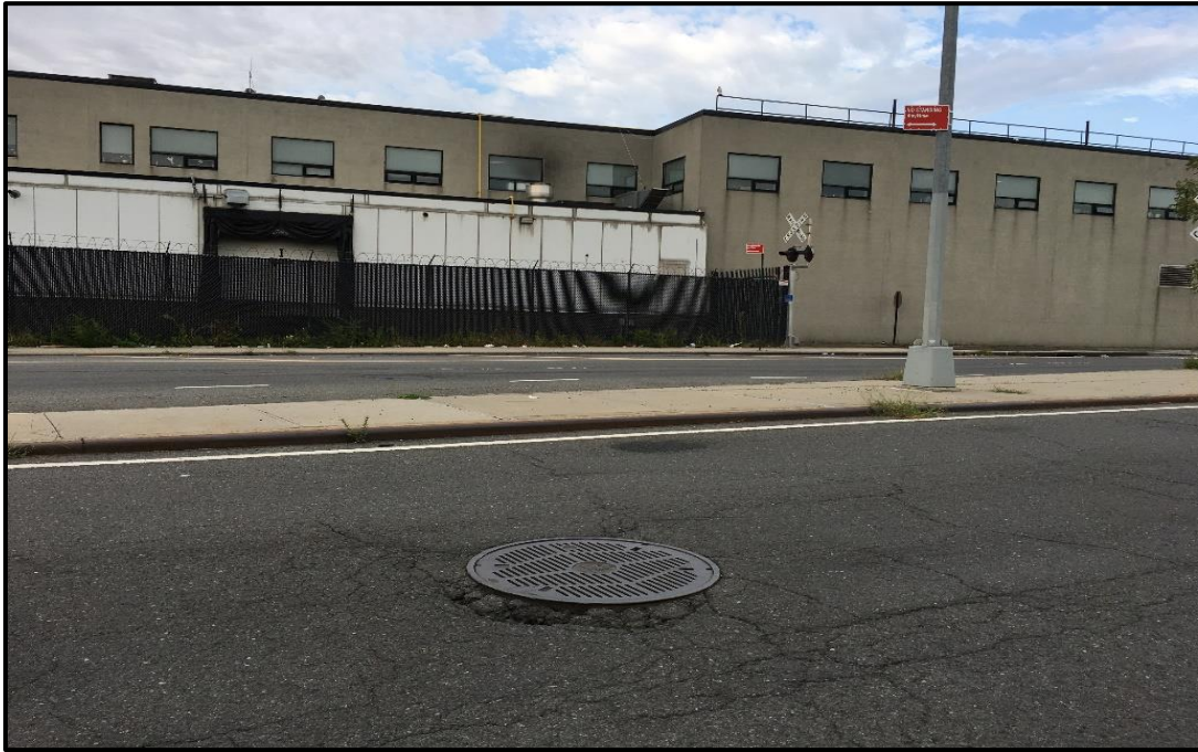
Photo 9: Facing west towards Baldor Foods (BCP Site 155 FCD). Minor cracking in asphalt around Con Edison manhole.
