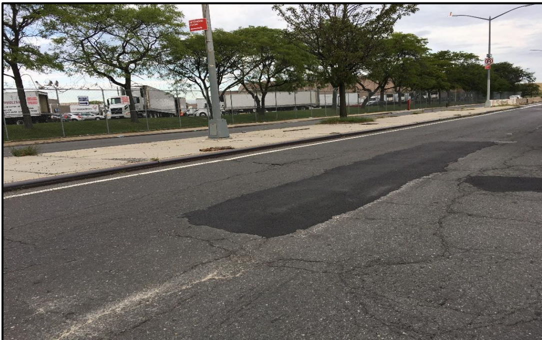
Photo 2: Facing north towards the Meat Market (BCP Site 355 FCD); adjacent to former VCP Site C; roadway generally in good condition. Evidence of minor asphalt patching.
