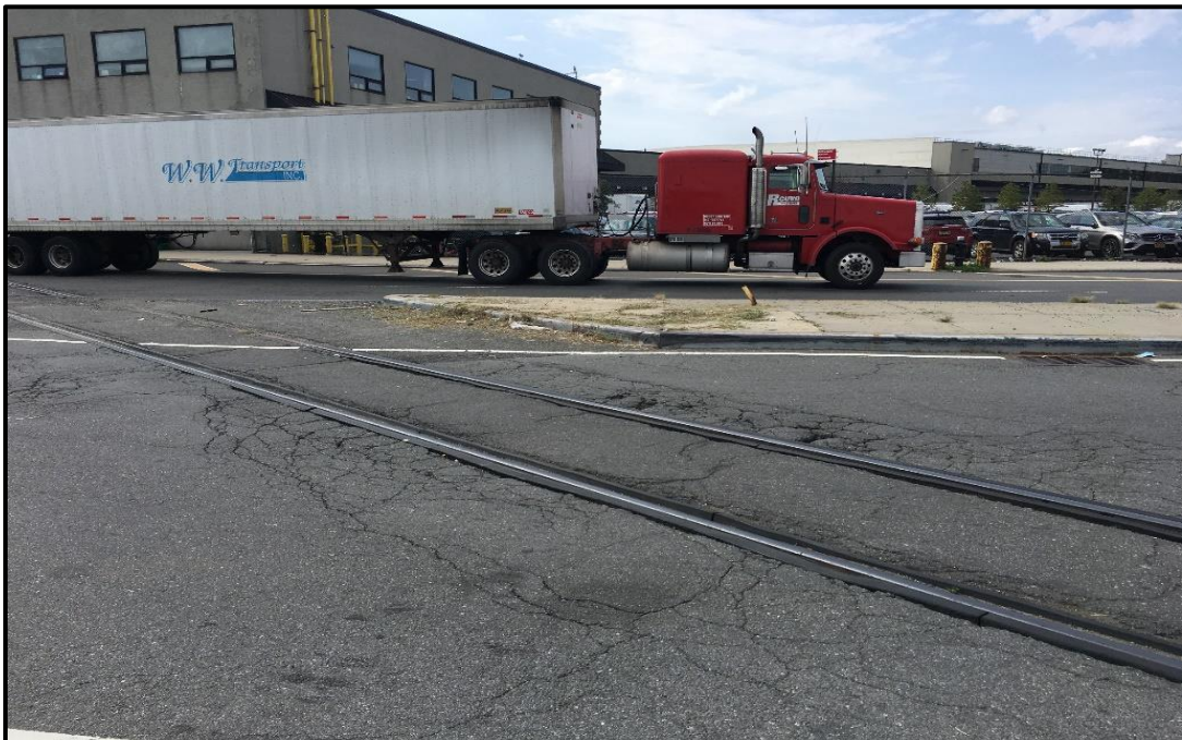
Photo 8: Facing west towards Baldor Foods (BCP Site 155 FCD). Minor cracking in asphalt around former railway lines.
