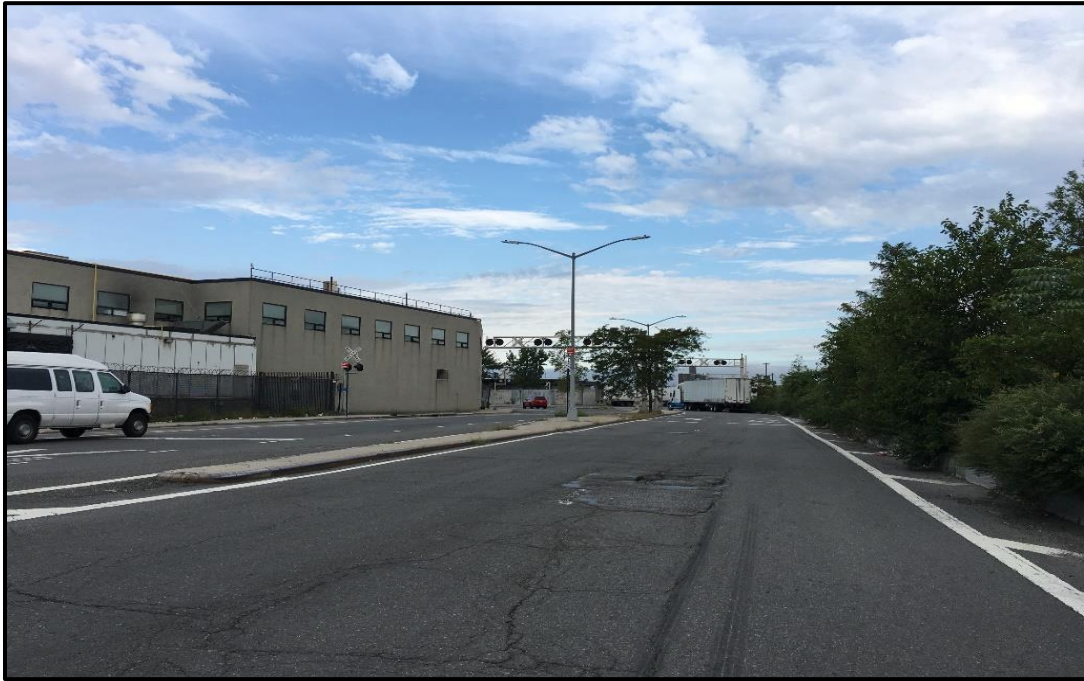
Photo 5: Facing east; Food Center Drive between Baldor Foods (BCP Site 155 FCD); and BCP Site D. Minor cracking and potholes within the asphalt pavement.
