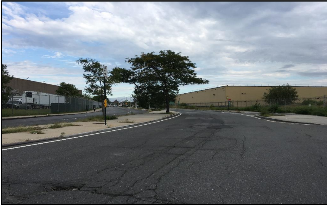
Photo 3: Facing north; FCD between Krasdale Foods (BCP Site 400 FCD) and the Meat Market (BCP Site 355 FCD). Minor cracking within the asphalt pavement. Location of two test pits performed in January 2019 in the background with cap still in place.
