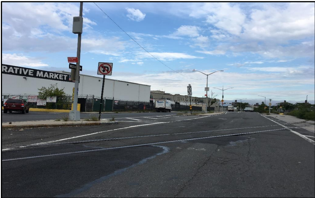
Photo 4: Facing northwest at the northeast portion of Food Center Drive, adjacent to the Meat Market (BCP Site 355 FCD) entrance; roadway generally in good condition. Evidence of asphalt patching.
