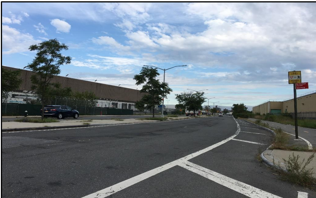
Photo 10: Facing northwest; Food Center Drive between Krasdale Foods (BCP Site 400 FCD) and the Meat Market (BCP Site 355 FCD). Roadway cap in place and in good condition with minor cracking and evidence of asphalt patching.
