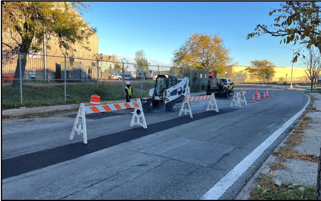
Photo 11: Facing northeast towards Krasdale Foods (BCP Site 400 FCD). Cowboy Contracting and All Pro performing asphalt milling for pothole repairs. Dust suppression performed with water tote and hose (November 2021).
