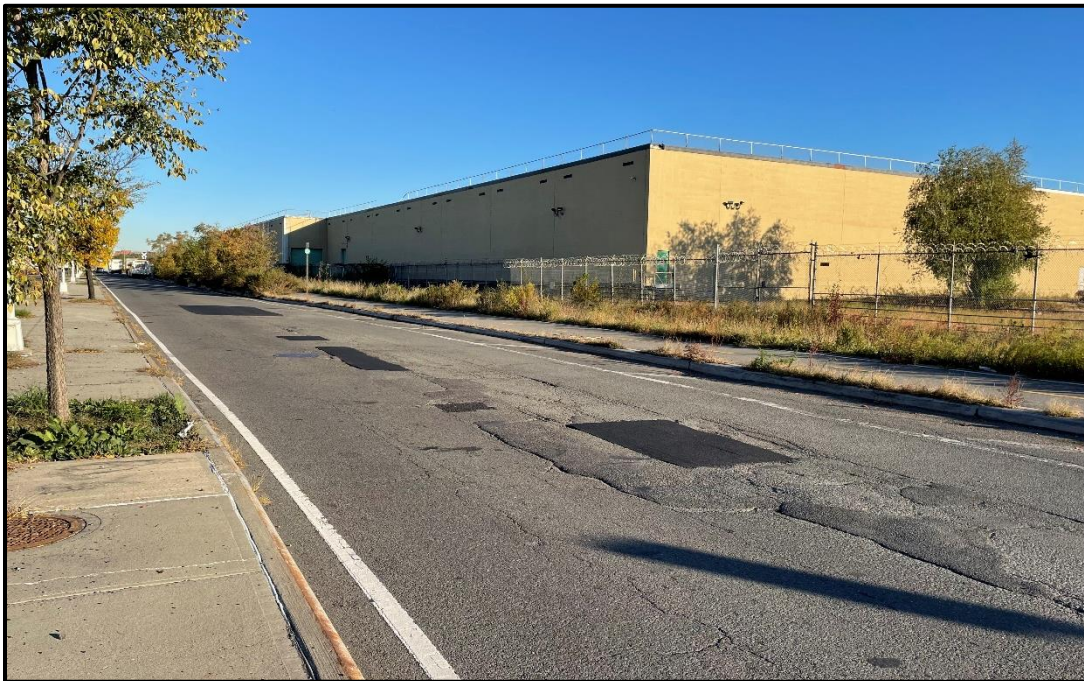
Photo 12: Facing northeast; Food Center Drive between Krasdale Foods (BCP Site 400 FCD) and the Meat Market (BCP Site 355 FCD). Pothole repairs/asphalt patching performed in the roadway by Cowboy Contracting and All Pro (November 2021).
