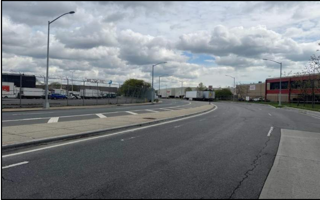
Photo 5: Facing northeast; Food Center Drive between Meat Market (BCP Site 355 FCD) and Sultana Distribution Services (BCP Site 600 FCD). Roadway generally in good condition with some minor cracking within the asphalt pavement.
