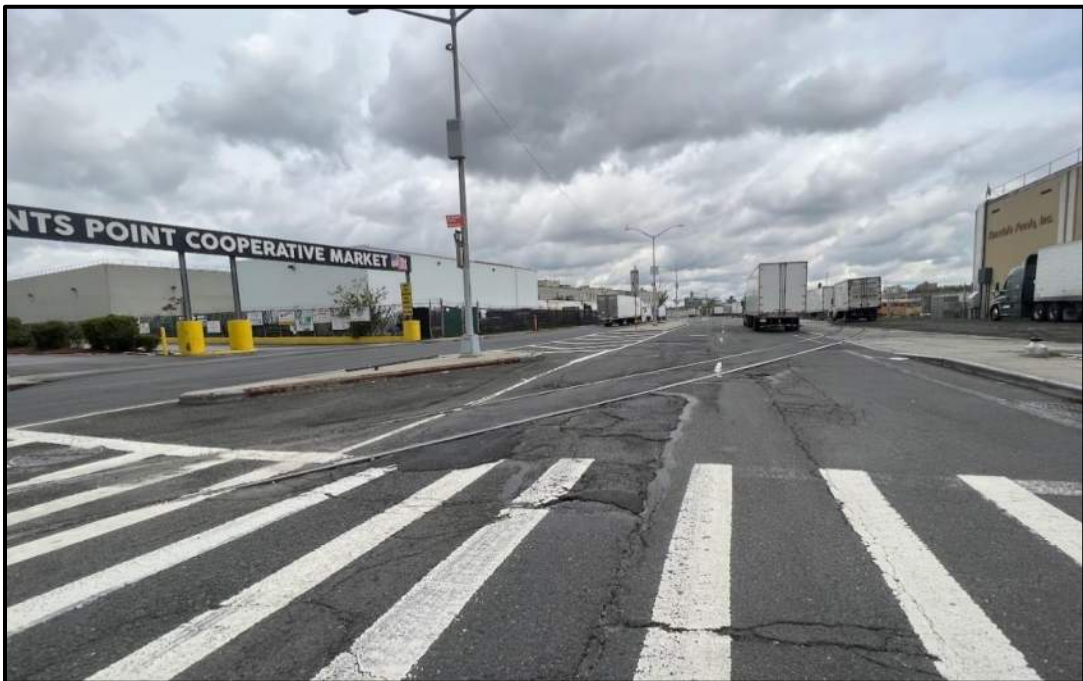
Photo 4: Facing northwest in the northeast portion of Food Center Drive, adjacent to the entrance of the Meat Market (BCP Site 355 FCD); roadway generally in good condition. Evidence of prior asphalt patching around the former railway lines.
