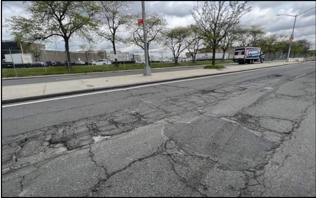
Photo 3: Facing northwest; FCD between Anheuser-Busch (VCP Site Parcel C) and the Meat Market (BCP Site 355 FCD). Minor cracking and potholes within the asphalt pavement.
