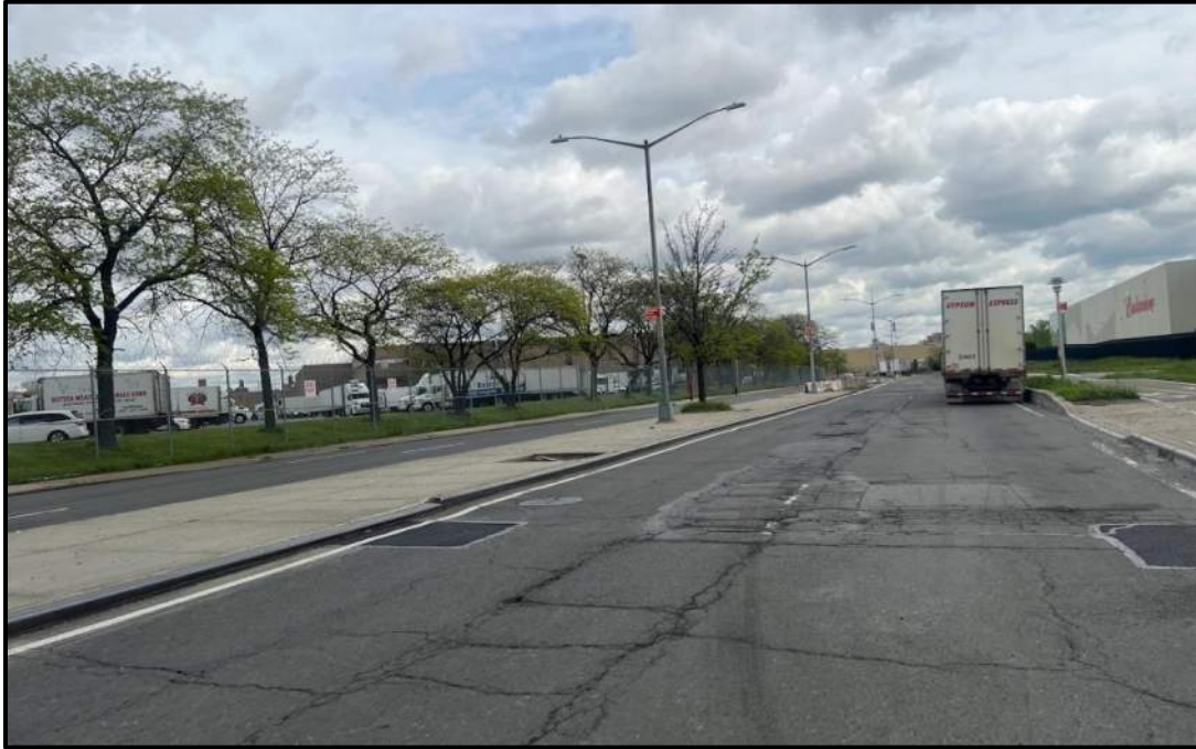
Photo 7: Facing west towards Meat Market (BCP Site 355 FCD), adjacent to Anheuser Busch (VCP Site Parcel C). Median in good condition. Minor cracking in the roadway, with recent asphalt patching present.
