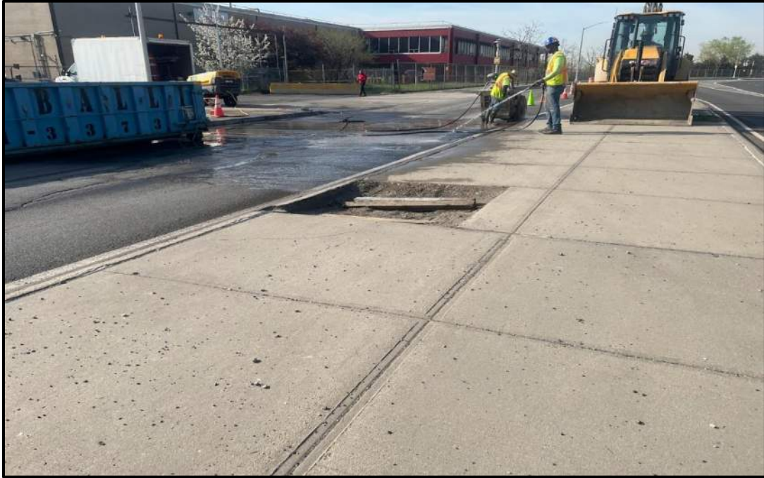
Photo 11: Facing south towards Sultana Distribution Services (BCP Site 600 FCD). Hylan performing saw cutting for fiber optic cable installation. Dust suppression performed with hydrant and hose (April 2023).
