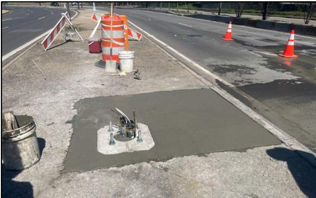
Photo 12: Facing northeast; Food Center Drive between Anheuser-Busch (VCP Site Parcel C) and the Meat Market (BCP Site 355 FCD). Concrete restoration around communications pole foundation in the roadway median by Hylan (April 2023).
