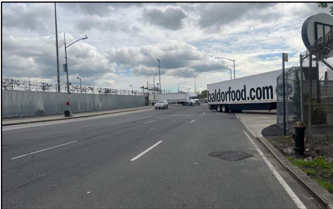
Photo 10: Facing east; Food Center Drive adjacent to the entrance for Baldor Foods (BCP Site 155 FCD). Roadway cap in place and in good condition with minor cracking and evidence of asphalt patching.
