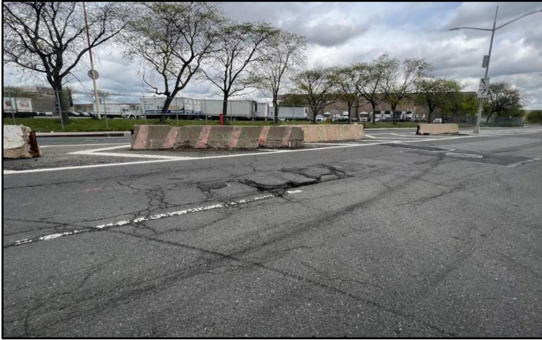
Photo 9: Facing north towards Meat Market (BCP Site 355 FCD). Minor cracking in asphalt, with recent asphalt patching around manhole.
