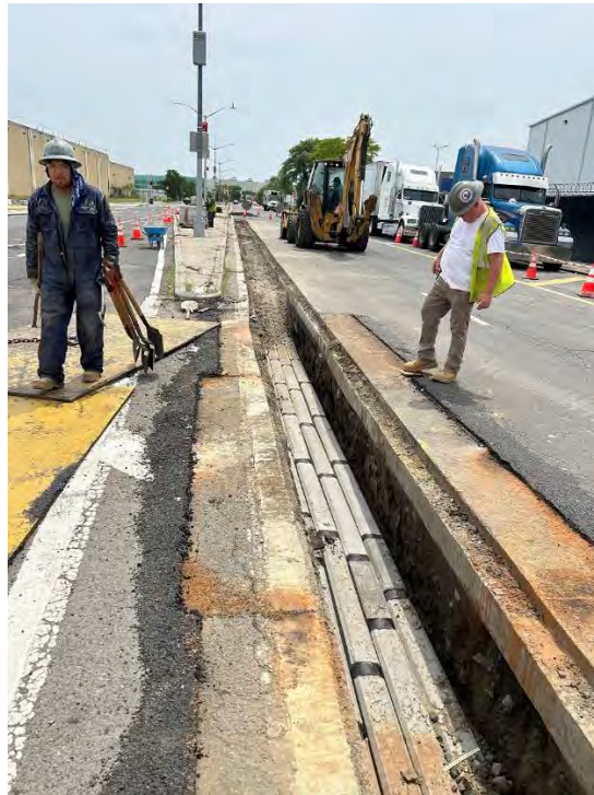
Photo 6: Backfilling trench 7-22-2024
