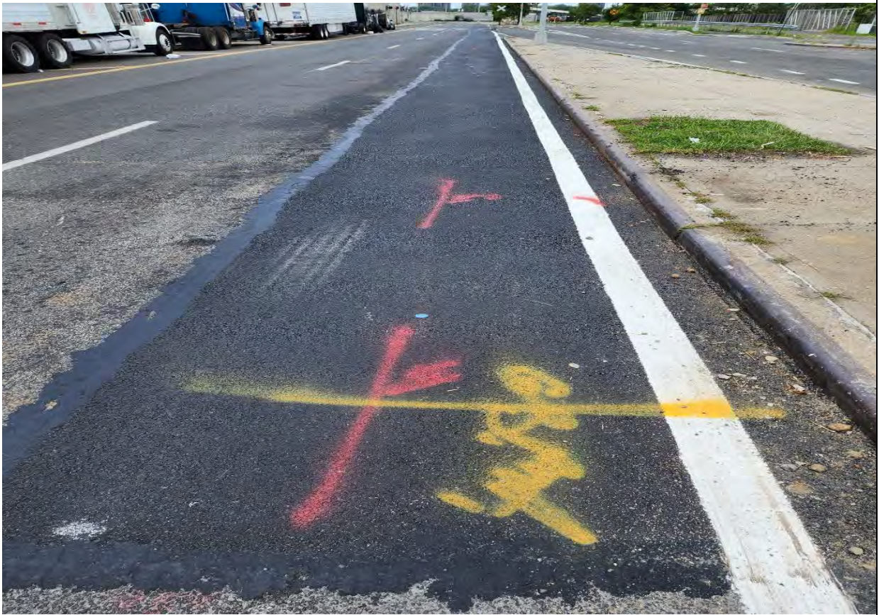
Photo 9: Completed trench paved over 7-31-2024
