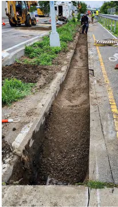
Photo 7: Trench backfilled 7-24-2024
