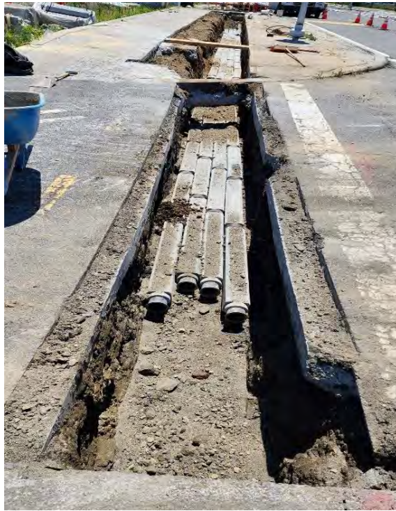
Photo 5: Excavation and duct installation progress 7-02-2024
