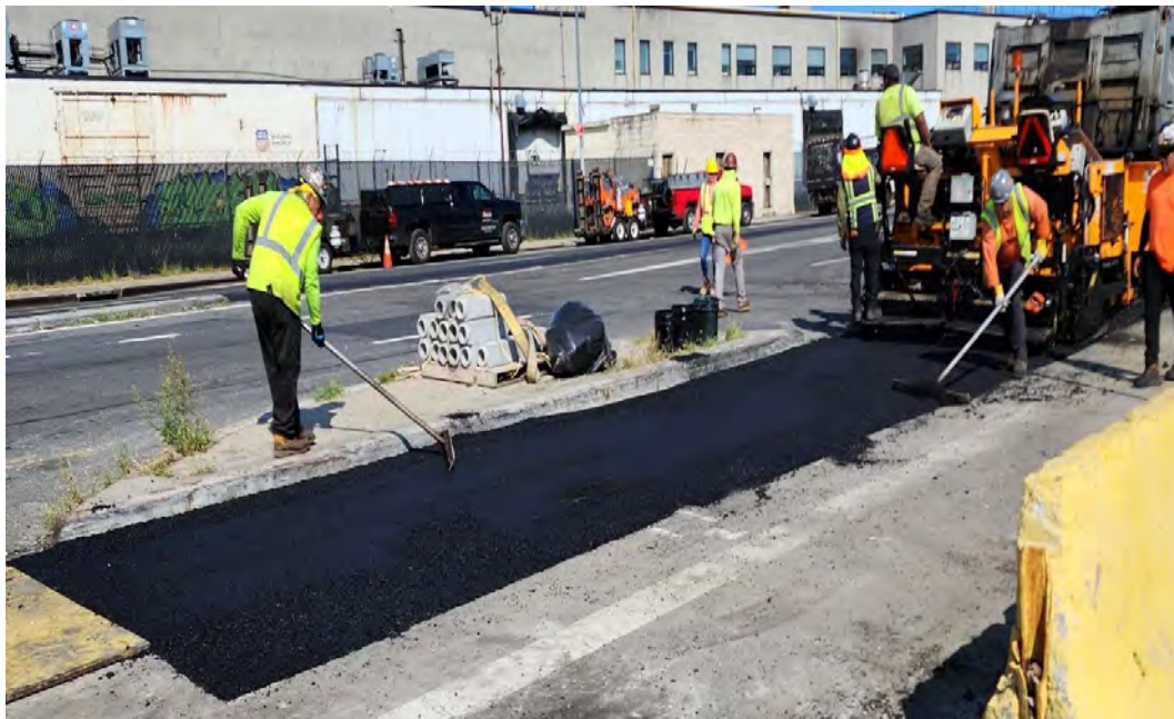
Photo 8: Blacktop paving over trench 7-26-2024
