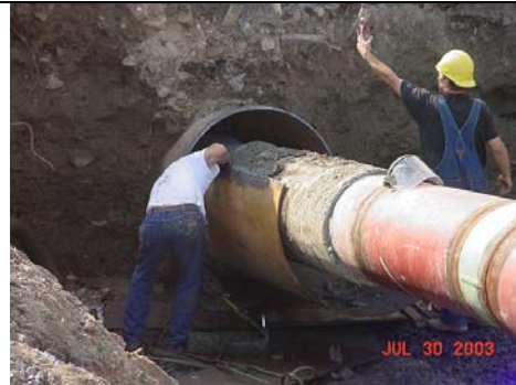
Photo 17. Cutting Casing
