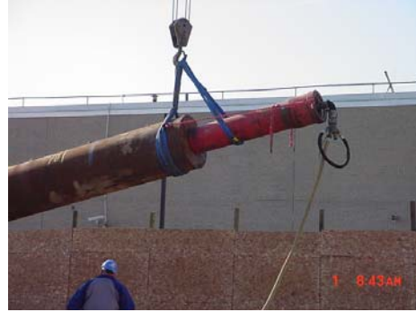
Photo 4. Piston Hammer
