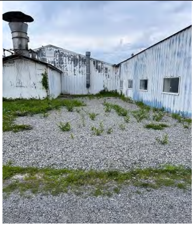
Cover System on east side of Building. Poinkers, Inc will install a No Parking sign.
