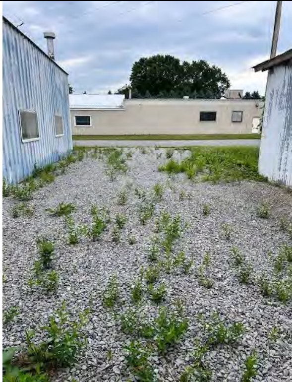
Cover system looking east toward CY Plastics facility.
