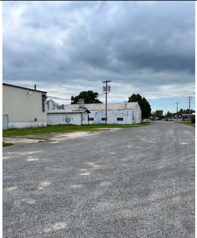
Facility driveway looking north.
