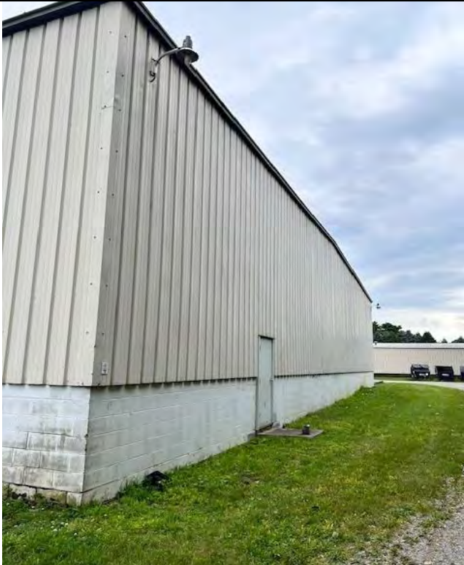
South side of building looking east.
