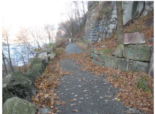
After – Looking North at Upper Retaining Wall
