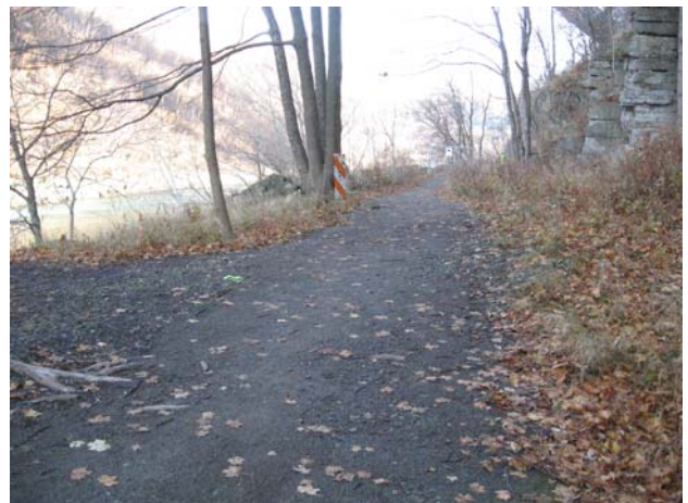
After – South end of Excavation Zone near Old Bridge Supports
