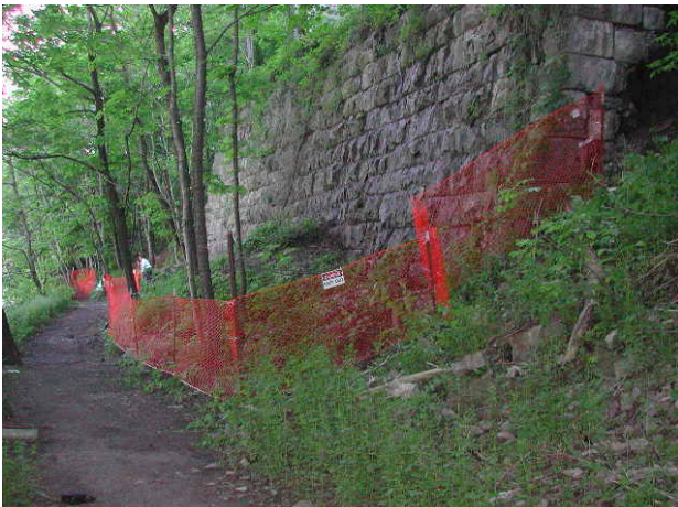
Before – Looking North at Upper Retaining Wall
