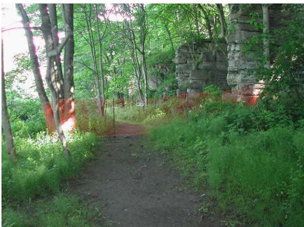
Before – South end of Excavation Zone near Old Bridge Supports
