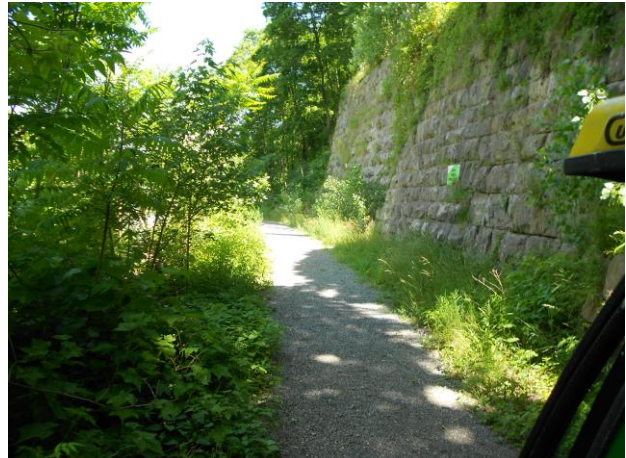
After – Looking North at Upper Retaining Wall
