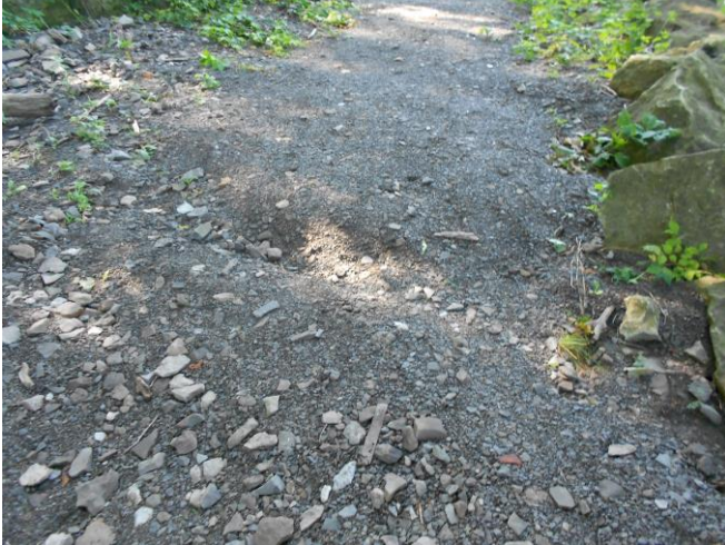
Ruts are forming across the Improved Trail as storm water and landslide debris flows across it near SW-2.
