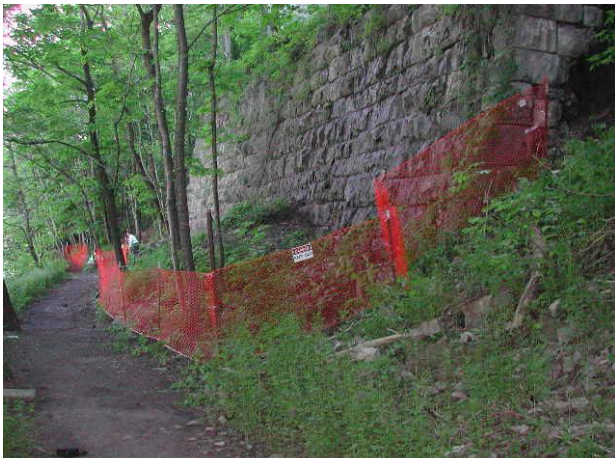
Before – Looking North at Upper Retaining Wall
