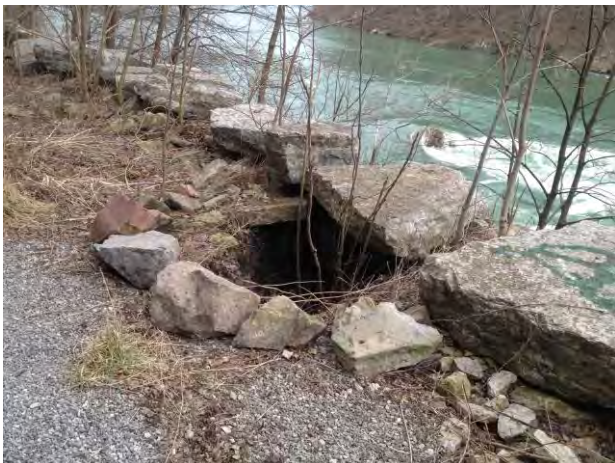
Before – Sink hole above the Lower Retaining Wall adjacent to the Improved Trail
