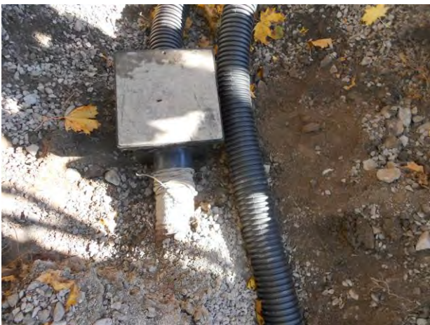
The Erosion Control drain pipe and SW-2 drain pipe run parallel under the Improved Trail
