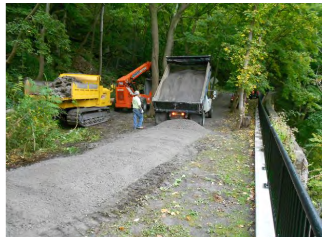
Crushed stone is brought in to protect the Improved Trail
