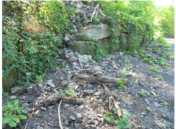
SW-2 and the improved trail are repeatedly covered with landslide debris after storm events. Landslide material easily washes over the existing stone block wall.
