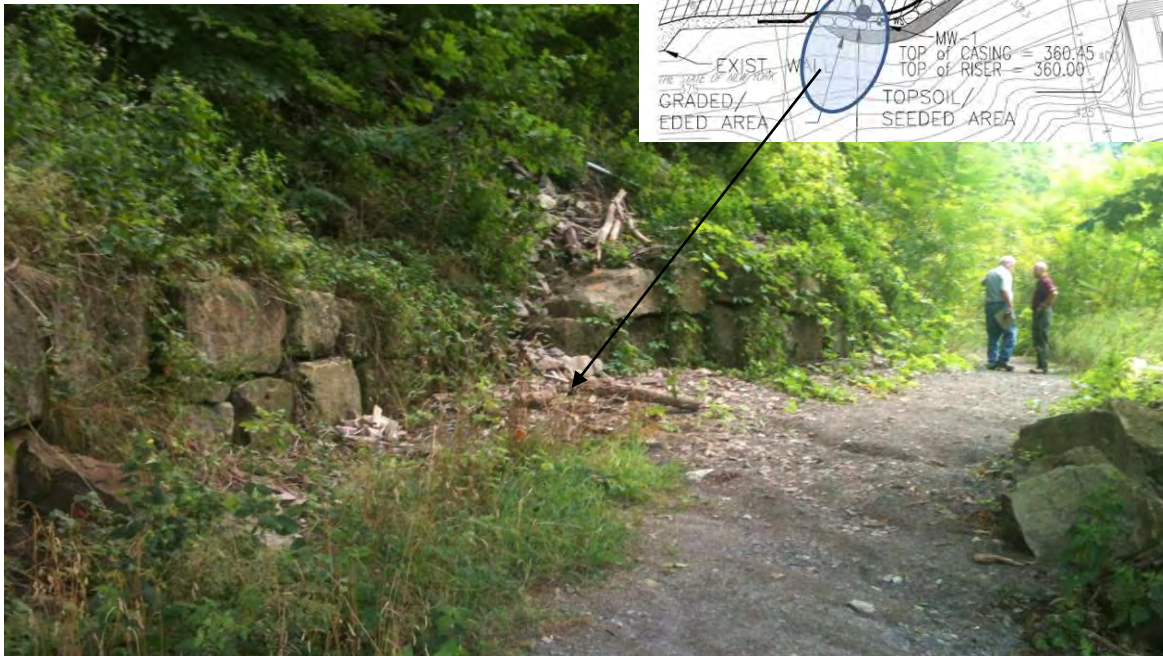
Overview showing the block wall to the north and south of the landslide area near SW-2. MW-1 is located a few yards north of SW-2 and has the same type of stone block wall protecting it. Movement of the slope is slowly pushing the adjacent stone over the monitoring well.
