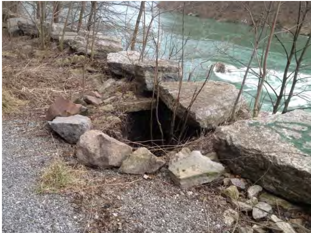
Sink hole by lower retaining wall; upper retaining wall is to the left (not visible)
