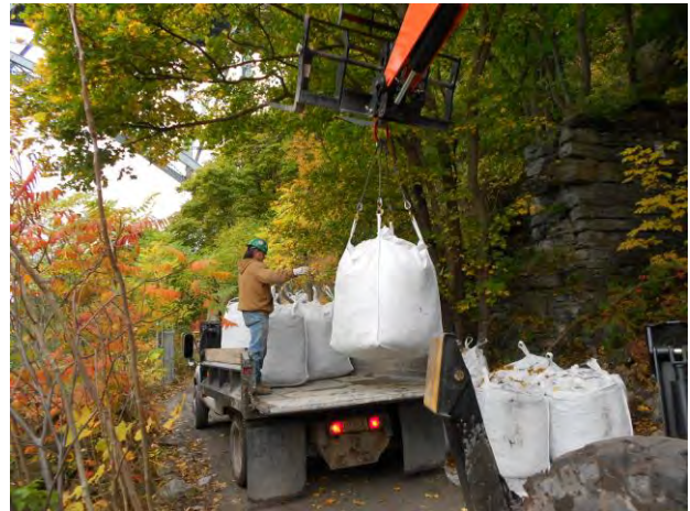
A truck is used to haul the soil bags up the trail to the Upper Staging Area
