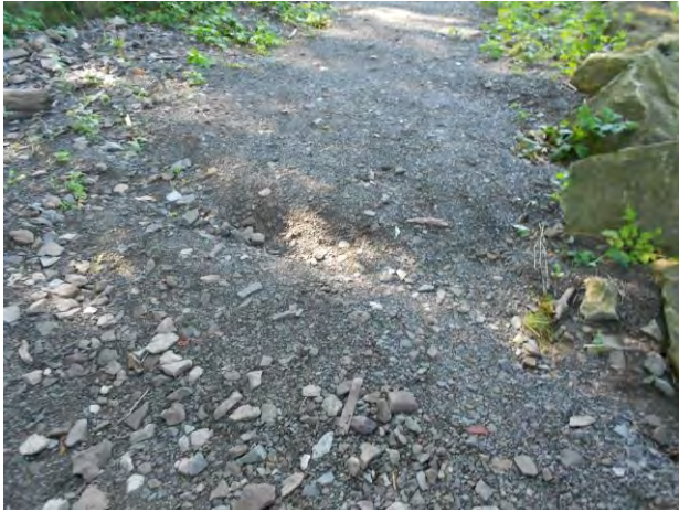
Before – Ruts are forming in the Improved Trail caused by storm water runoff near SW-2
