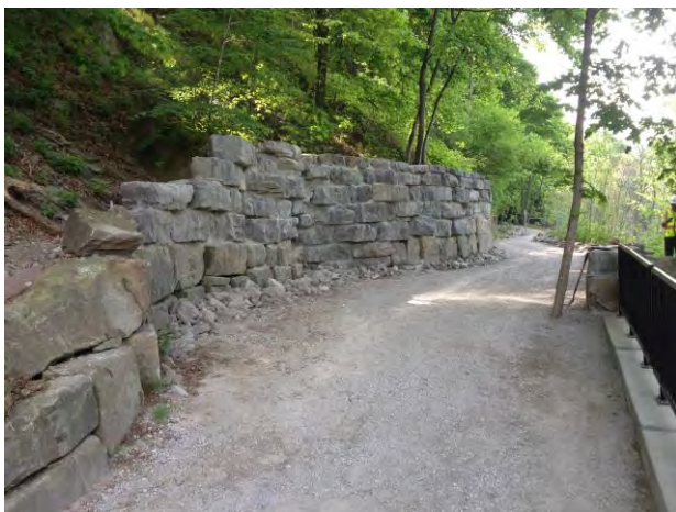
Looking south along the trail - a Final Inspection view of the front face of the Erosion Control Wall
