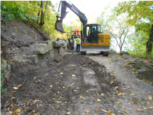
A Landslide material on the trail is excavated and disposed
