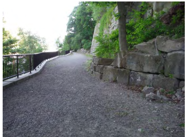
After – The sink hole is filled and a metal railing has been added above the Lower Retaining Wall
