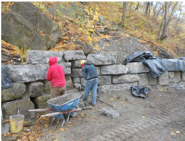
Grout is added to both the front and back of the wall after stones are placed
