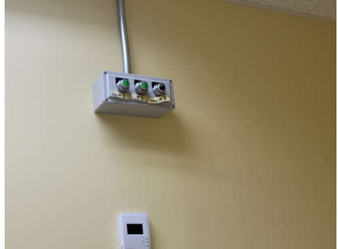
Photo 2: View of PMS associated with the SSDS fan units.
