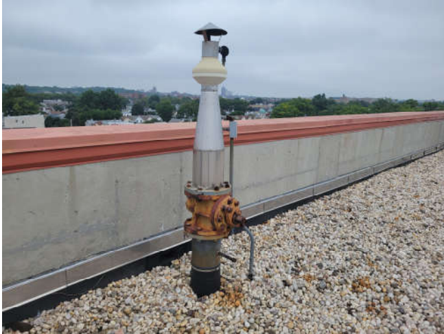
Photo 1: View of typical SSDS fan unit on the roof.
