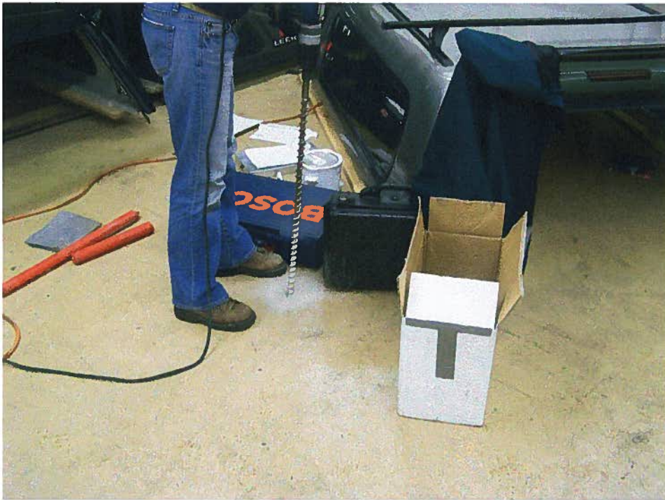
Photo No. 10. Installation of Sub-Slab Vapor Sample Point SVS-JCL-02 (April 2007)
