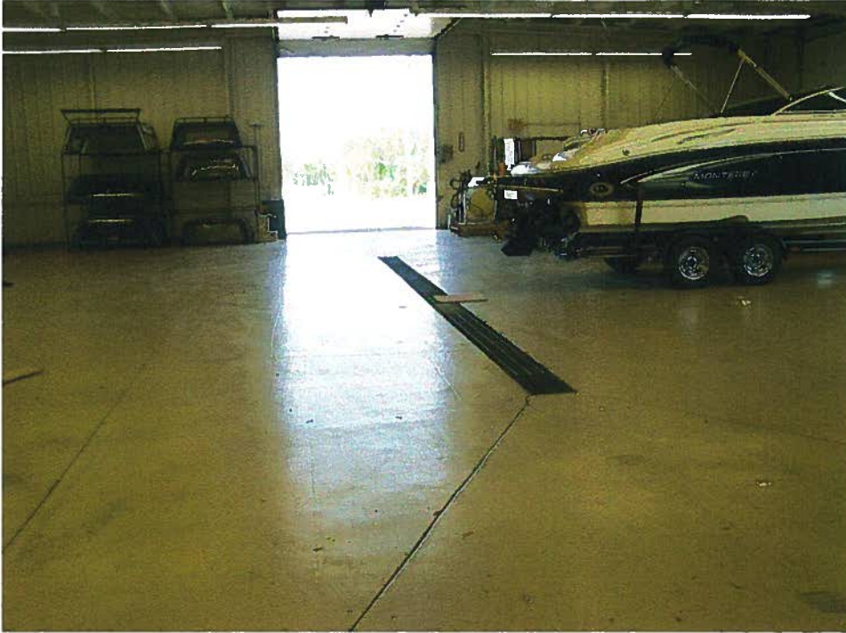
Photo No. 13. Trench Drain Located in Central Portion of Service Area (June 2007)
