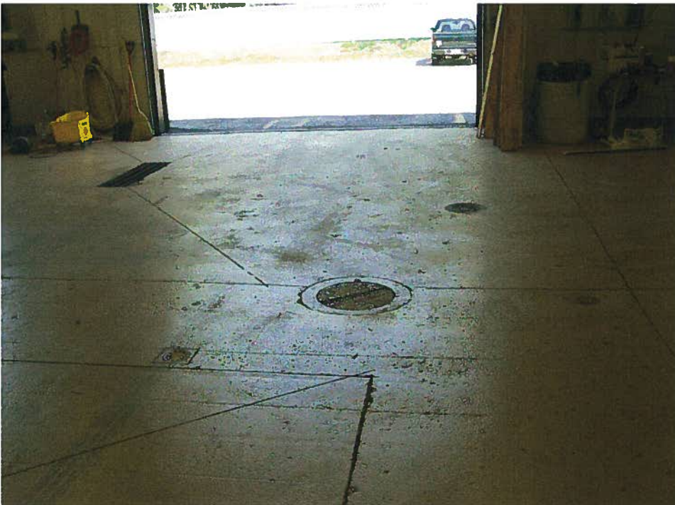
Photo No. 14. Oil/Water Separator Located Inside Service Area Portion of Building (June 2007).
