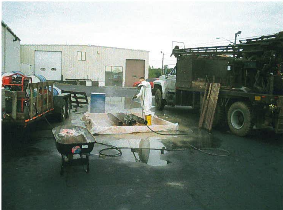
Photo No. 2. Decon of Drilling Equipment Between Well Locations (September 2006)
