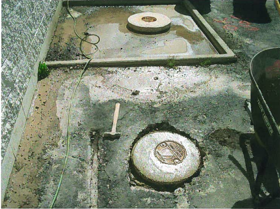
Photo No. 3. Completion of MW-JCL-02 in service Area (September 2006)
