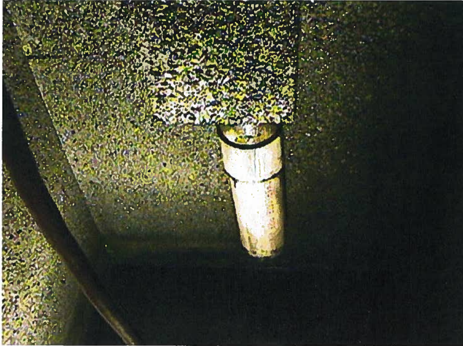
Photo No. 15. Interior of Oil/Water Separator. 4" PVC Outlet Pipe Visible on East Wall of Tank (February 2008).
