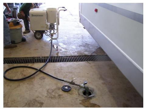
Photo No. 6. View of Geoprobe GS2000 injection pump hooked to injection well.
