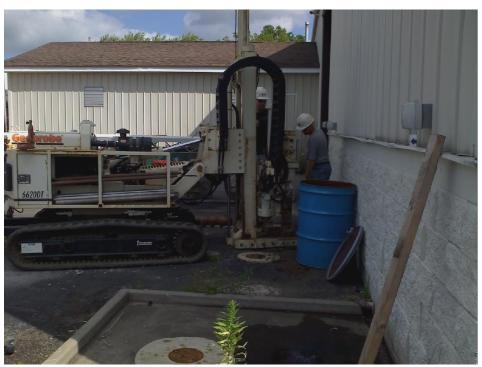
Photo No. 1. View looking north at installation of injection well in source area of site, along west wall of building.
