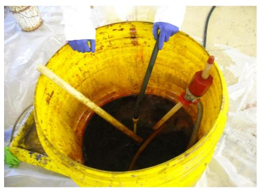
Photo No. 4. Adding water to permanganate solution in poly drum for appropriate mixture.
