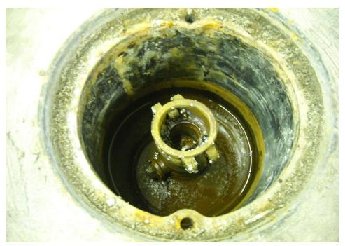
Photo No. 2. View of typical flush mount injection well completion with steel ball valve assembly.
