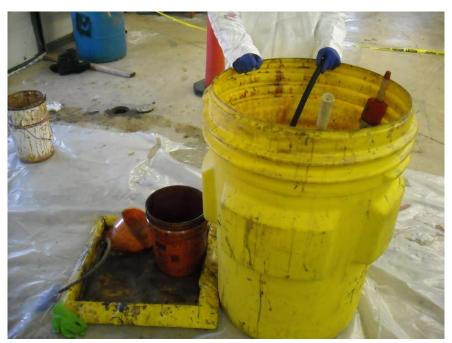
Photo No. 5. View of poly mixing drum and injection supplies.
