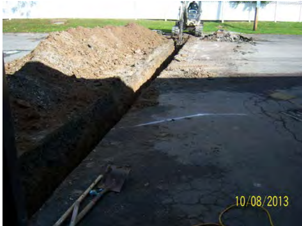
Photo 7. View of waterline trench excavation.
