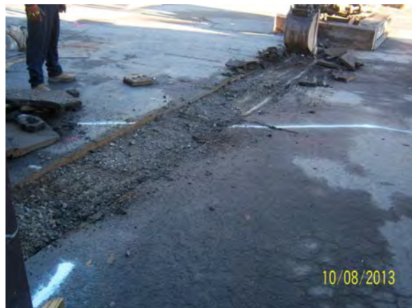
Photo 6. View of asphalt removal prior to trenching for waterline.
