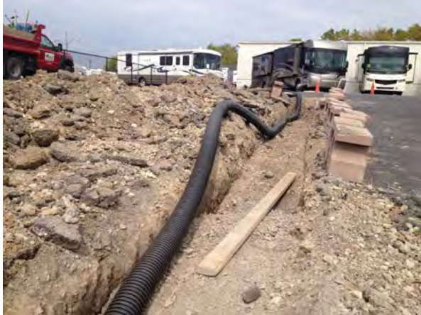
Photo 1. View to north, shallow retaining wall trench excavation.
