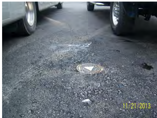
Photo 12. View of new pavement & box, MW-13.
