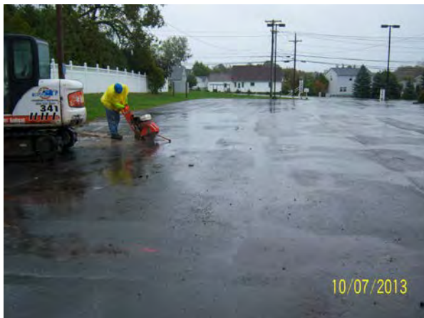
Photo 5. View to east, asphalt cutting for waterline installation.
