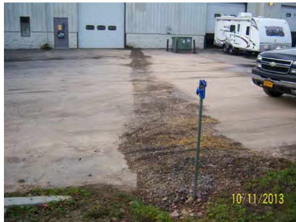
Photo 10. View to south, waterline installation complete with backfilling prior to repaving.
