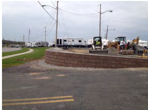
Photo 4. View to west, new retaining wall construction.
