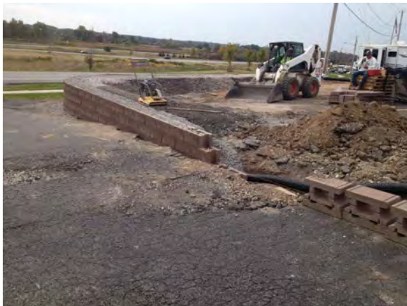
Photo 3. View to southwest, retaining wall construction at N. Sanford Rd. entrance.
