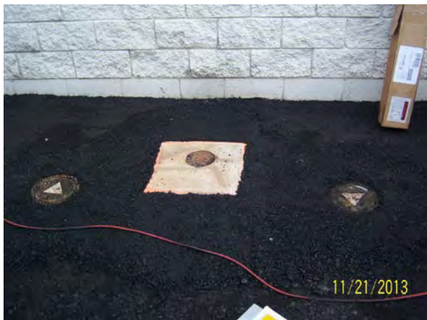
Photo 11. View of new protective curb boxes & new asphalt pavement at MW-3, MW-JCL-02.
