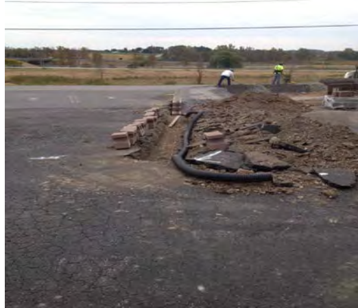
Photo 2. View to south, asphalt cut and shallow trench excavation.
