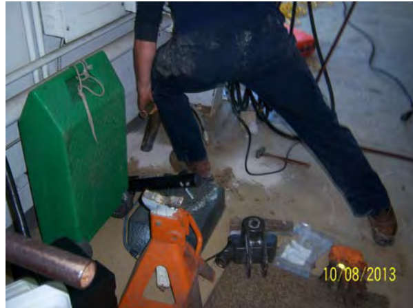
Photo 8. View of interior concrete coring for waterline access.
