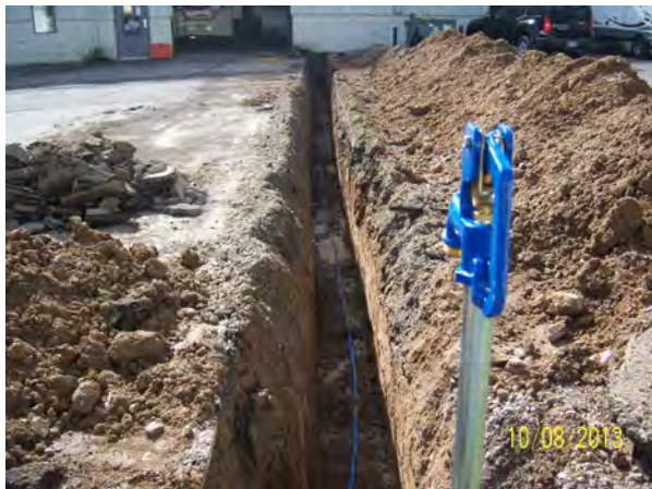
Photo 9. View to south, new waterline & spigot installed.
