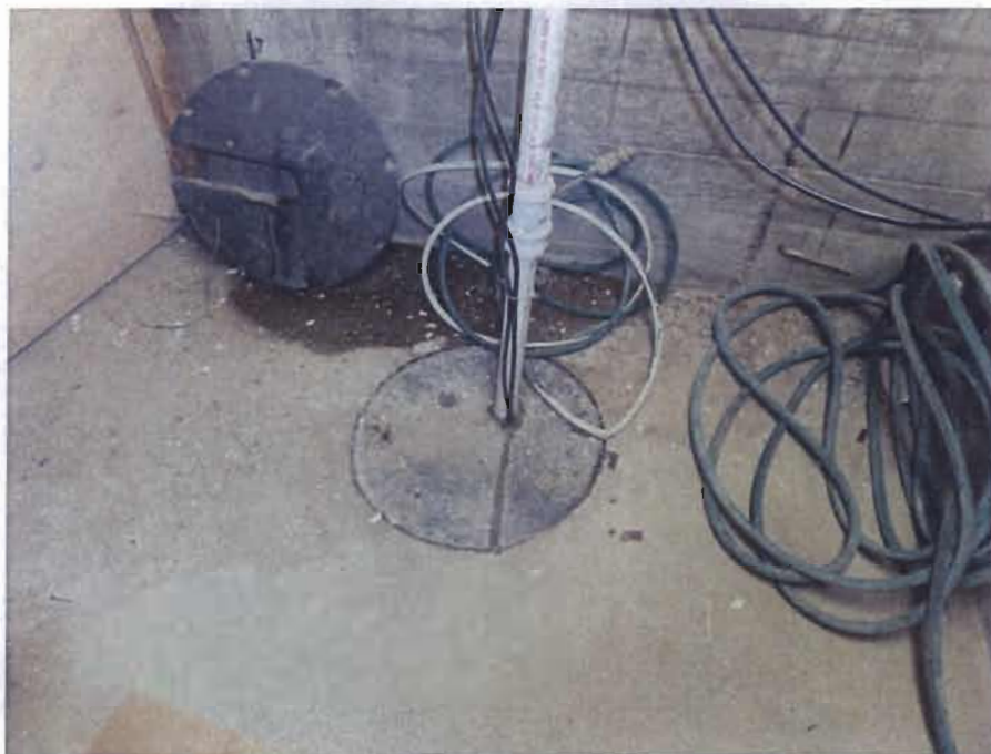
Photograph 5 – Sealed Sump in Building Basement
