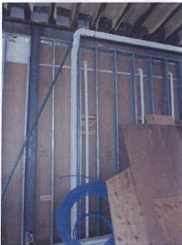
Photograph 6 – SSV Mitigation Piping – Southern Vent
