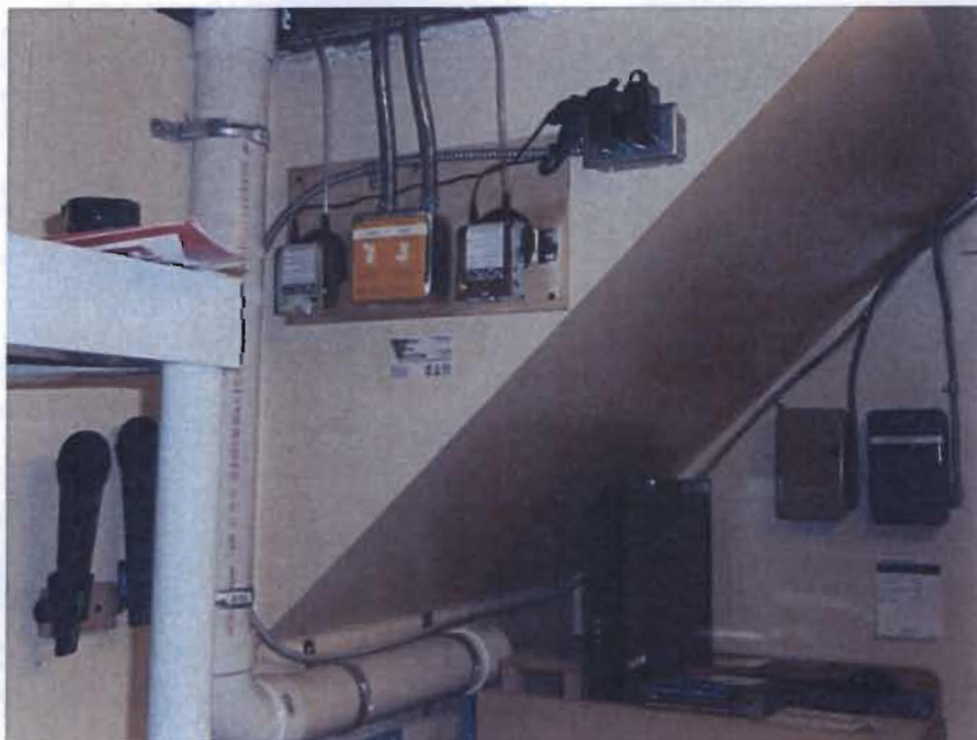
Photograph 4 – SSV Mitigation System Controls and Monitoring Equipment
