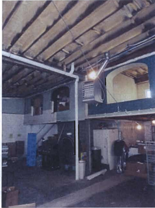
Photograph 7 – SSV Mitigation Piping – Southern Vent
