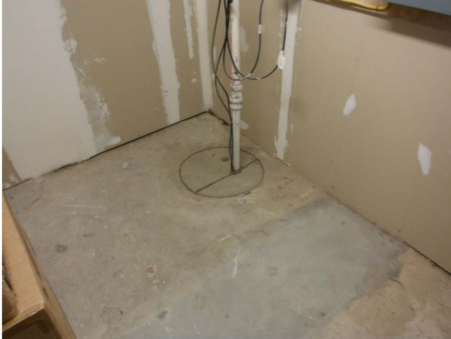
Photograph 5 – Sealed Sump in Building Basement
