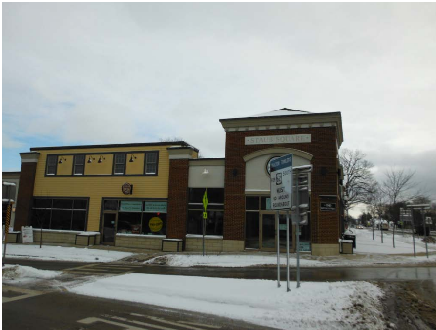
Photograph 12 – Front or Building Exterior (South Side)
