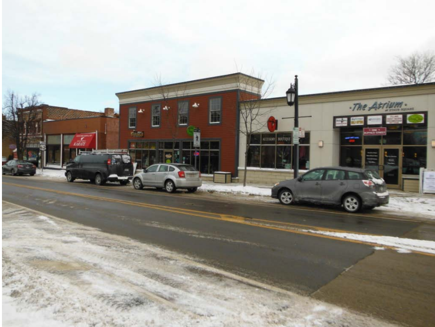
Photograph 13 – Front or Building Exterior (North Side)
