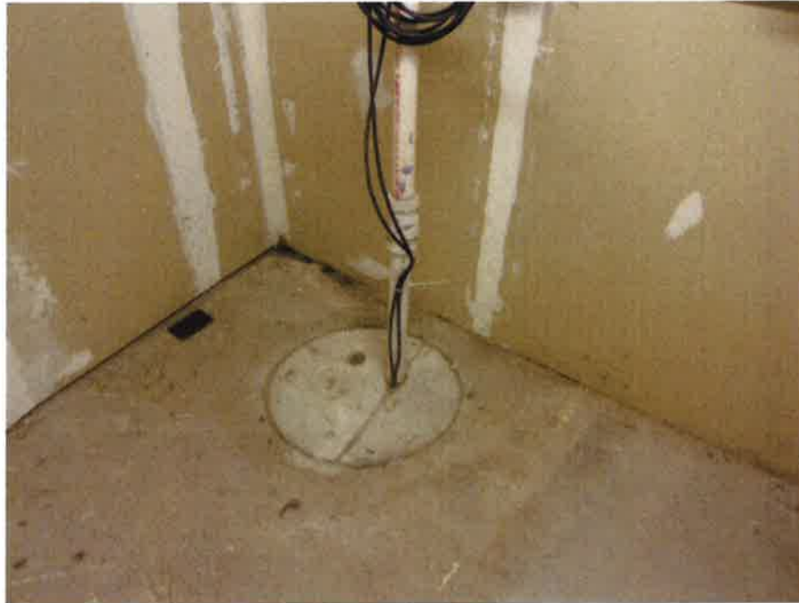
Photograph 5 – Sealed Sump in Building Basement
