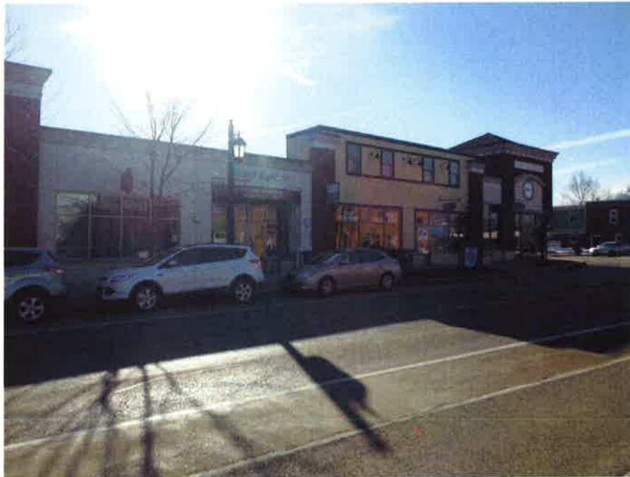
Photograph 10 – Front of Building Exterior from Buffalo Street
