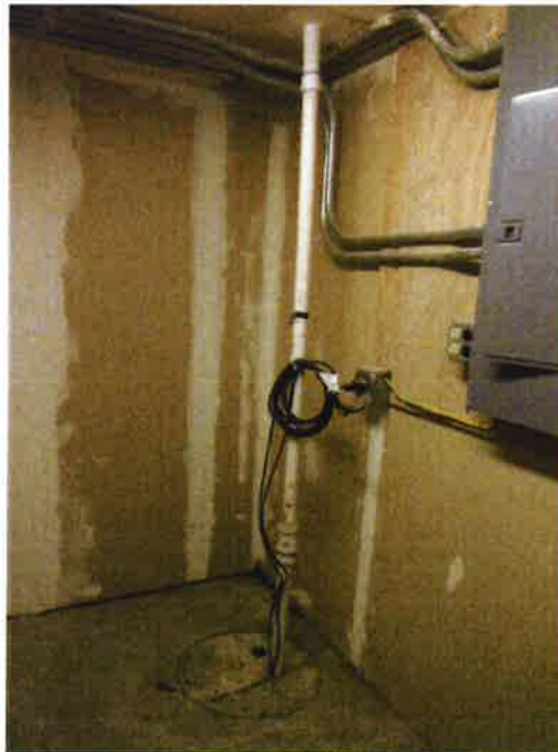
Photograph 10 – Sealed Sump in Building Basement
