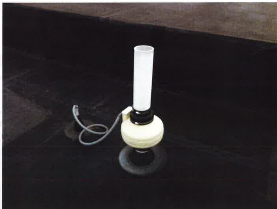
Photograph 2 – Southern SSV Mitigation Roof Fan
