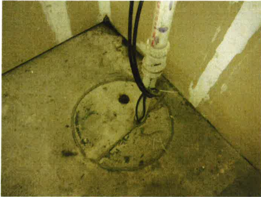
Photograph 9 – Sealed Sump in Building Basement
