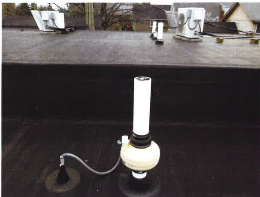
Photograph 1 – Northern SSV Mitigation Roof Fan
