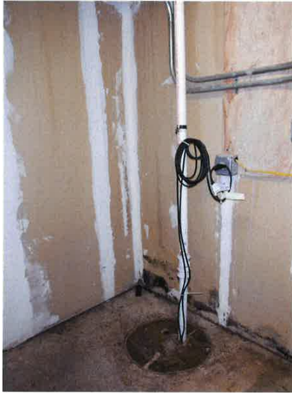
Photograph 9 – Sealed Sump in Building Basement
