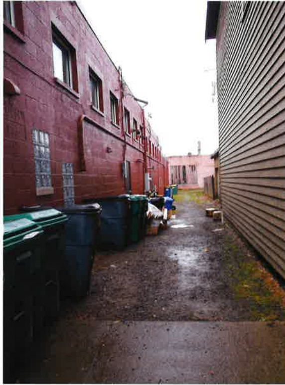
Photograph 3 – Unpaved Alleyway (North of the Building Looking West)
