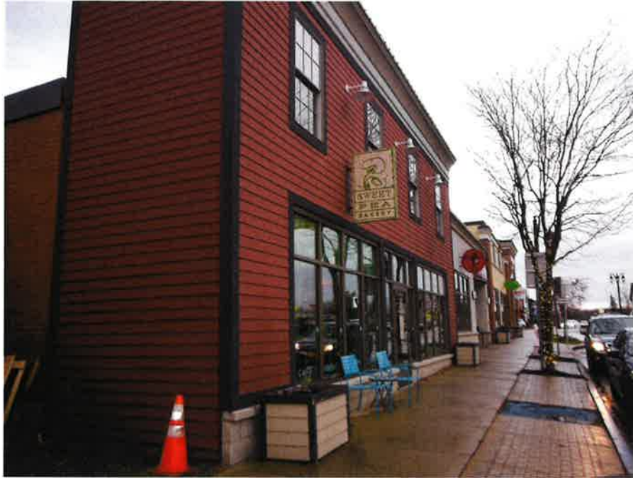
Photograph 5 – Building Exterior (Buffalo St. Looking East)
