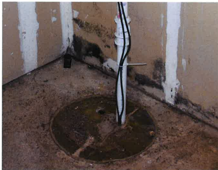
Photograph 10 – Sealed Sump in Building Basement
