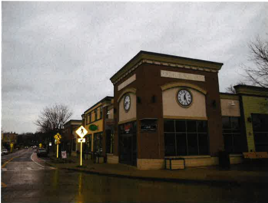
Photograph 6 – Building Exterior (Corner of One Buffalo St. & E. Main St.)
