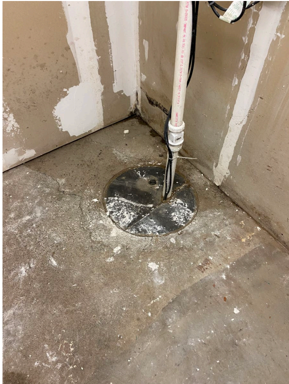
Photograph 5: Sealed sump pump in building basement (3/4/2022)
