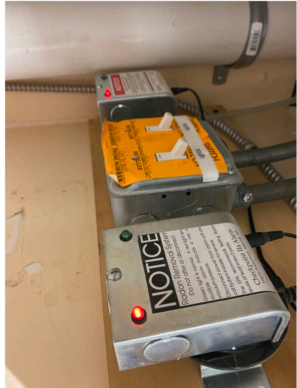
Photograph 7: SSV mitigation system controls and monitoring equipment manually tripped (3/4/2022)
