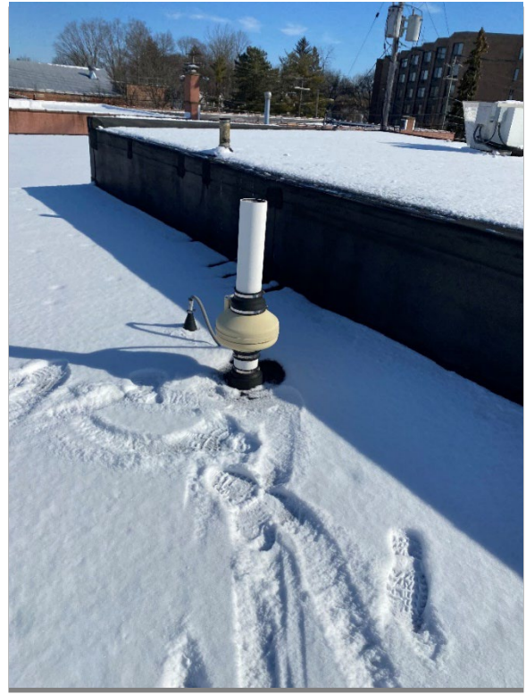
Photograph 3 North SSV Mitigation roof fan (3/4/2022)
