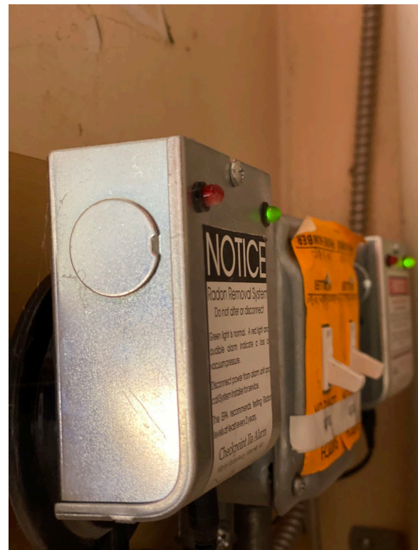
Photograph 8: SSV mitigation system controls and monitoring equipment (3/4/2022)
