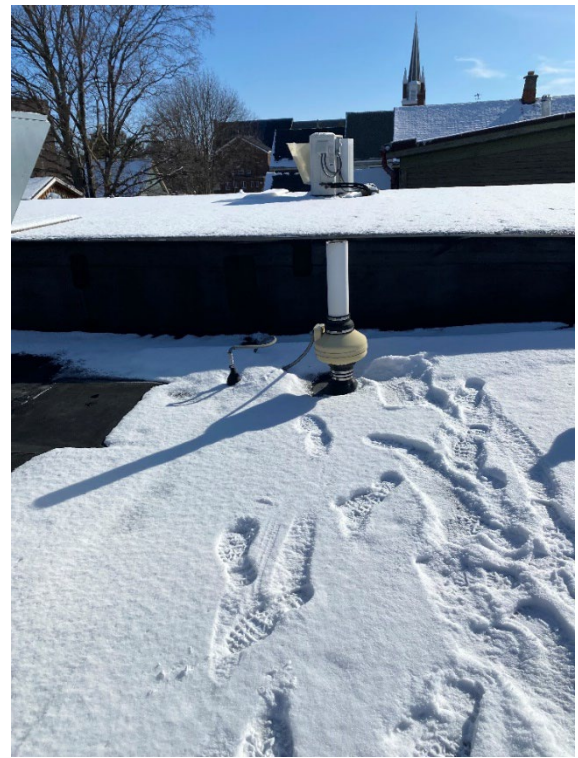
Photograph 4 South SSV mitigation roof fan (3/4/2022)
