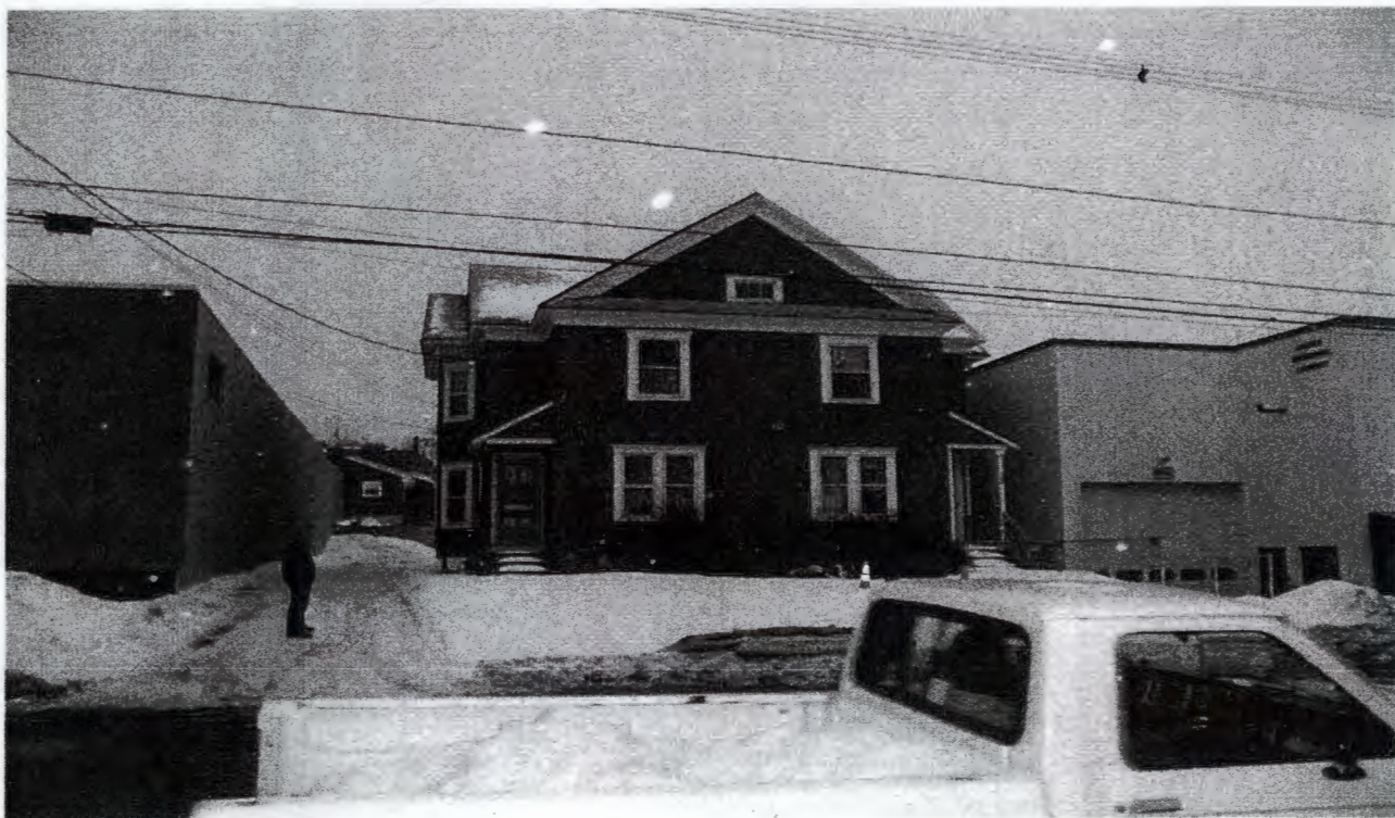
Photograph showing the Allied Industrial Laundry residence at 3009 Milton Avenue.
