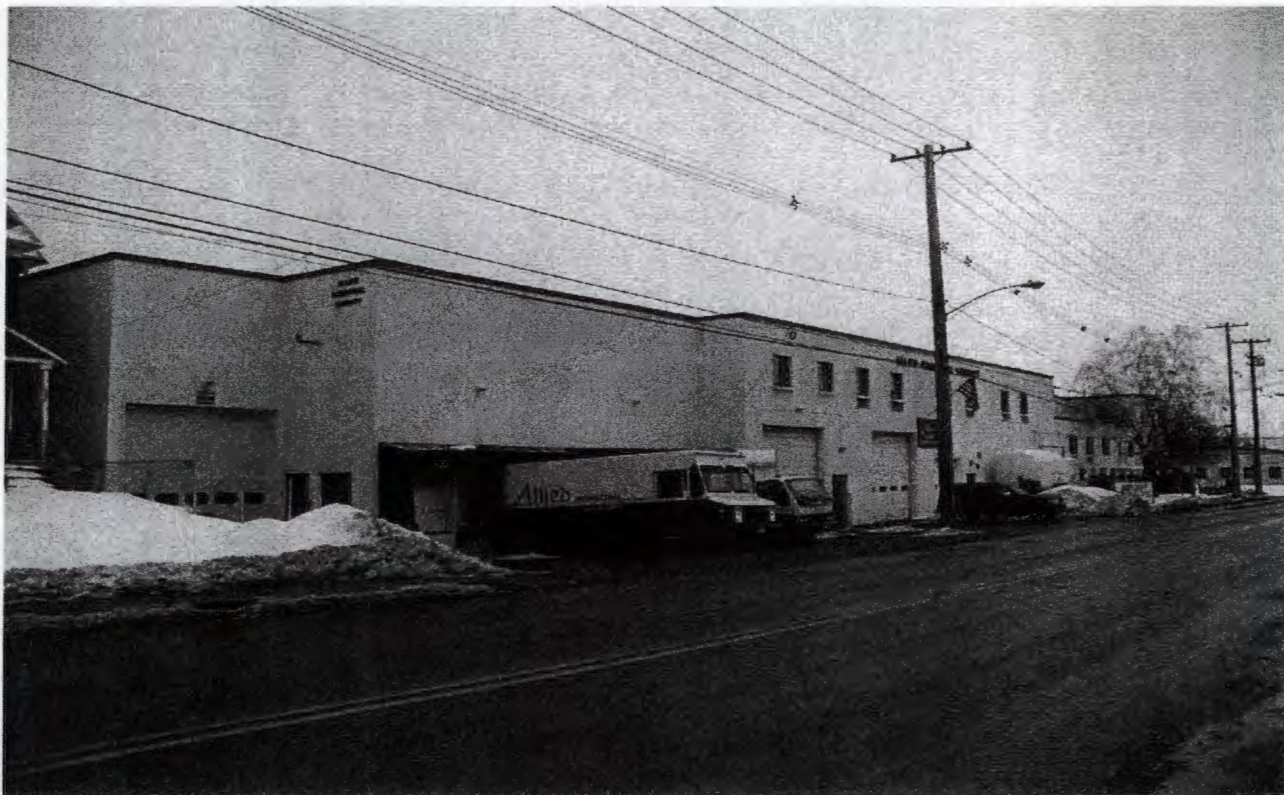
Photograph showing the Allied Industrial Laundry Plant.
