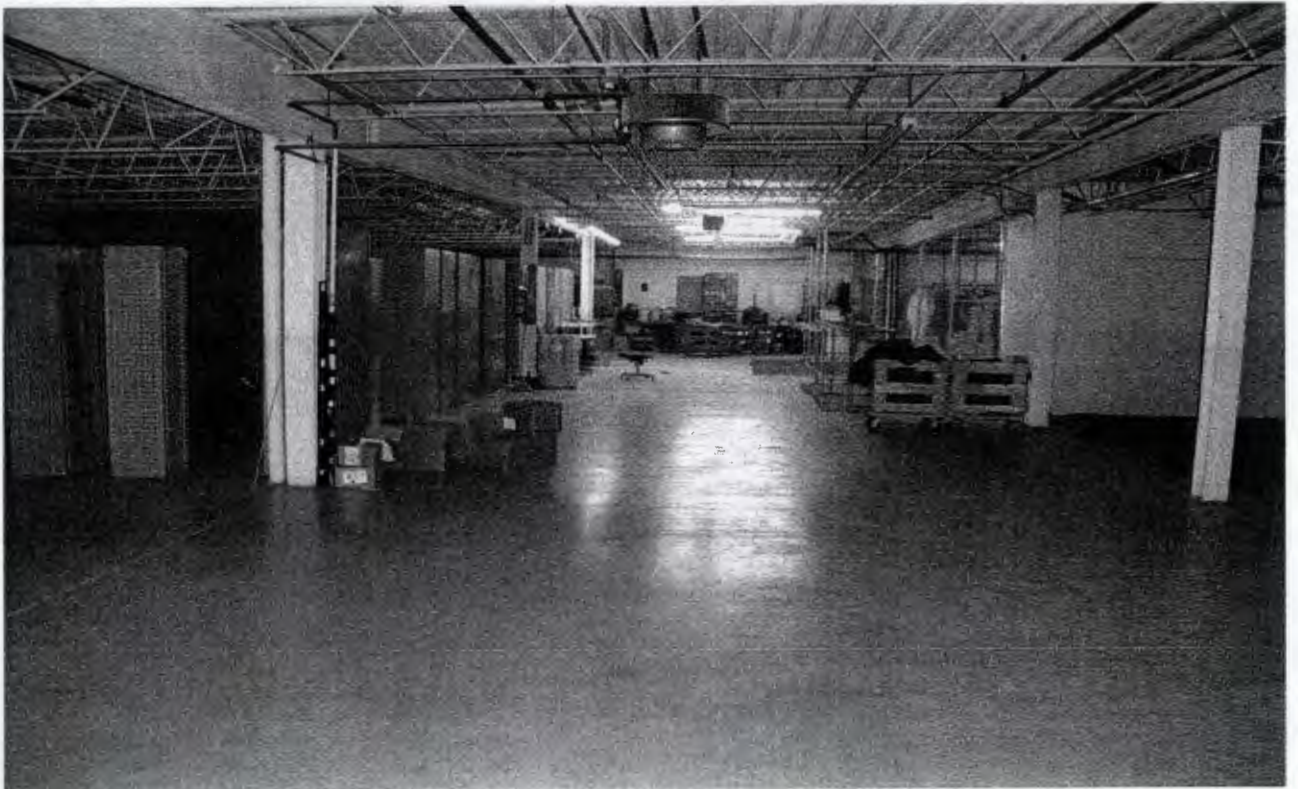
Photograph showing second floor of plant.
