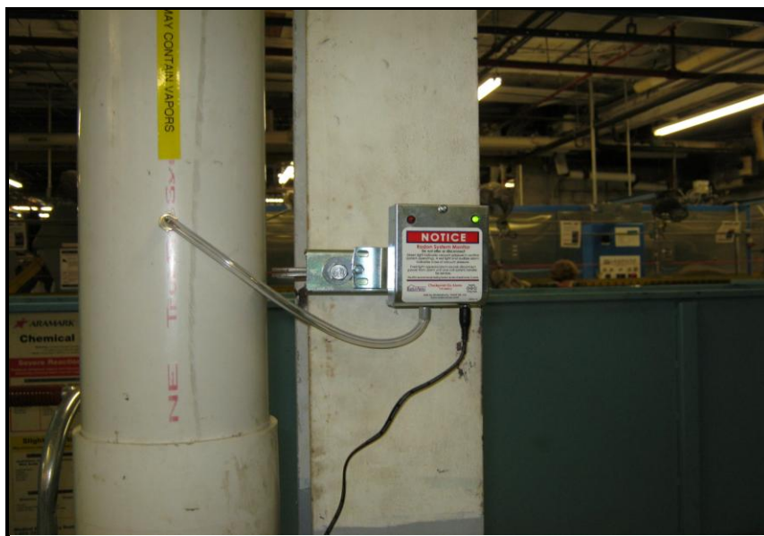
Photograph Number: 4 Photograph Description: Depressurization system riser and audible and visual alarm system.
