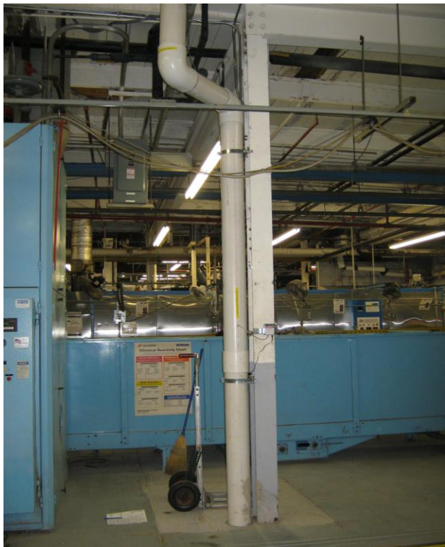
Photograph Number: 3 Photograph Description: Depressurization system riser
