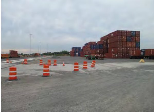
Photo 1: Environmental cap in Area 2A taken facing south.
