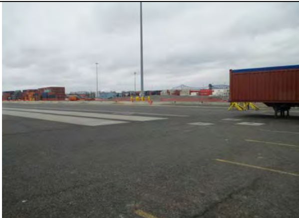
Photo 15: Asphalt cover in Site 2, Area 2A taken facing southwest.
