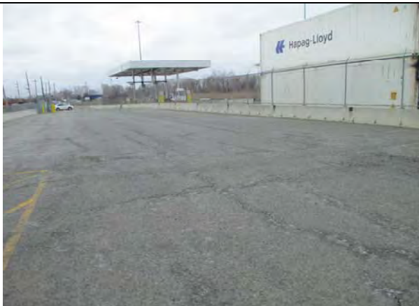
Photo 17: Asphalt cover in Site 2, Area 2A (taken facing northeast).
