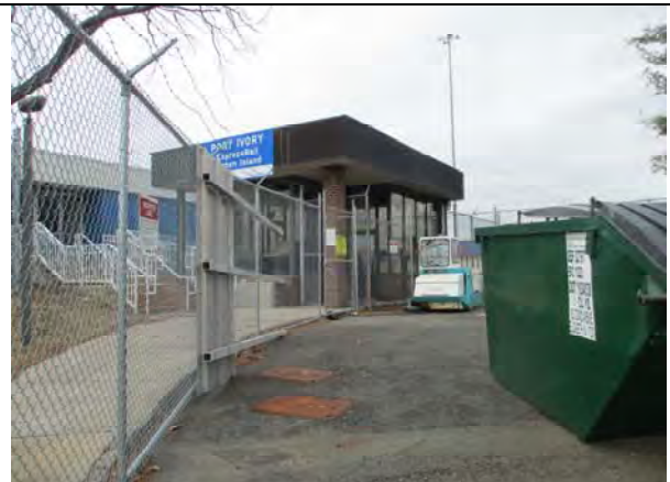
Photo 18: Building No. 40 and 45 in Site 2A.
