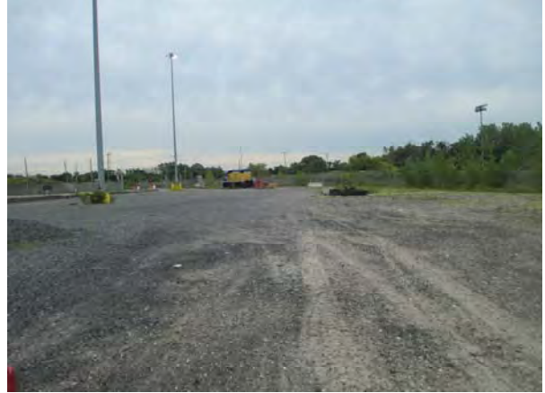
Photo 2: Environmental cap (one foot of crushed stone) in Area 2A taken facing south.
