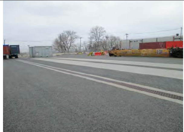
Photo 14: Asphalt cover in Site 2, Area 2A taken facing north.
