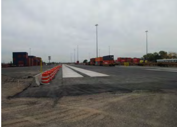
Photo 3: Asphalt and crushed stone in Area 2A taking facing north.
