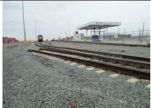
Photo 10: Railroad tracks in Site 2 Area, 2A (taken facing north).
