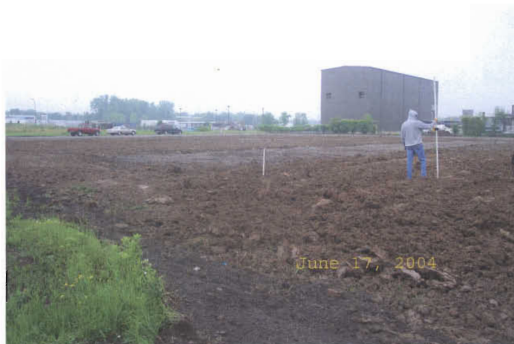
13 - Verification of 2' Cover Depth
