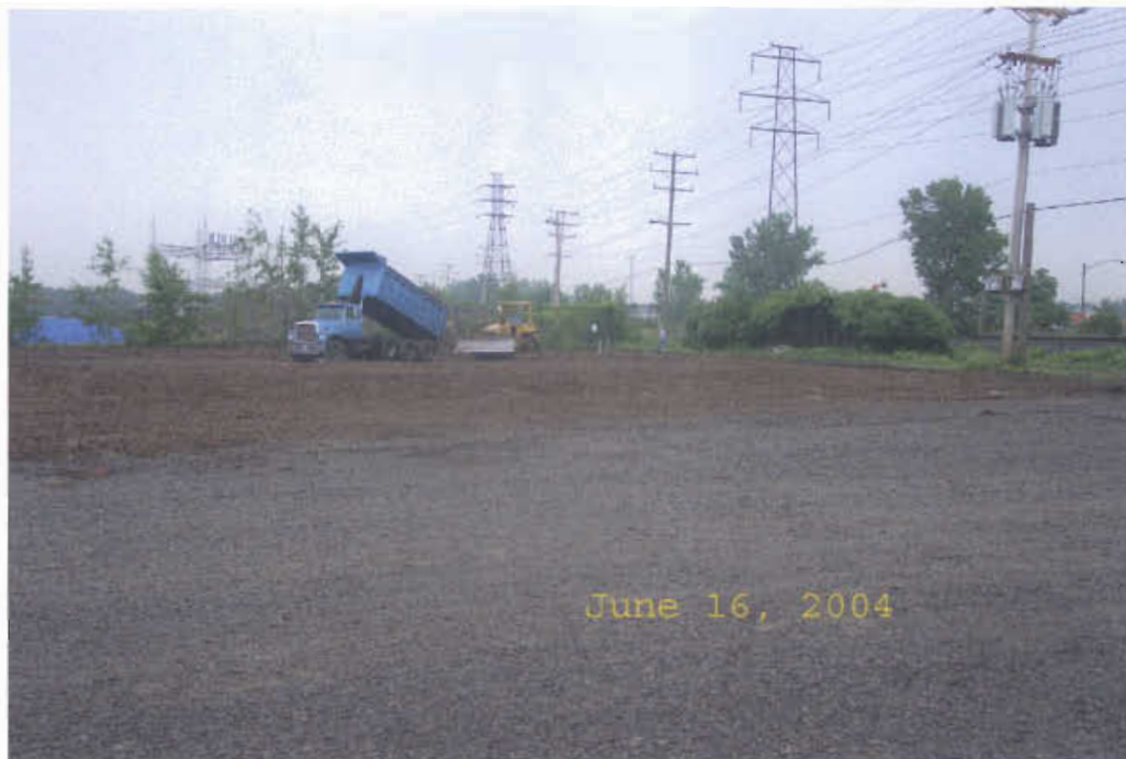
12 - Soil Backfill
