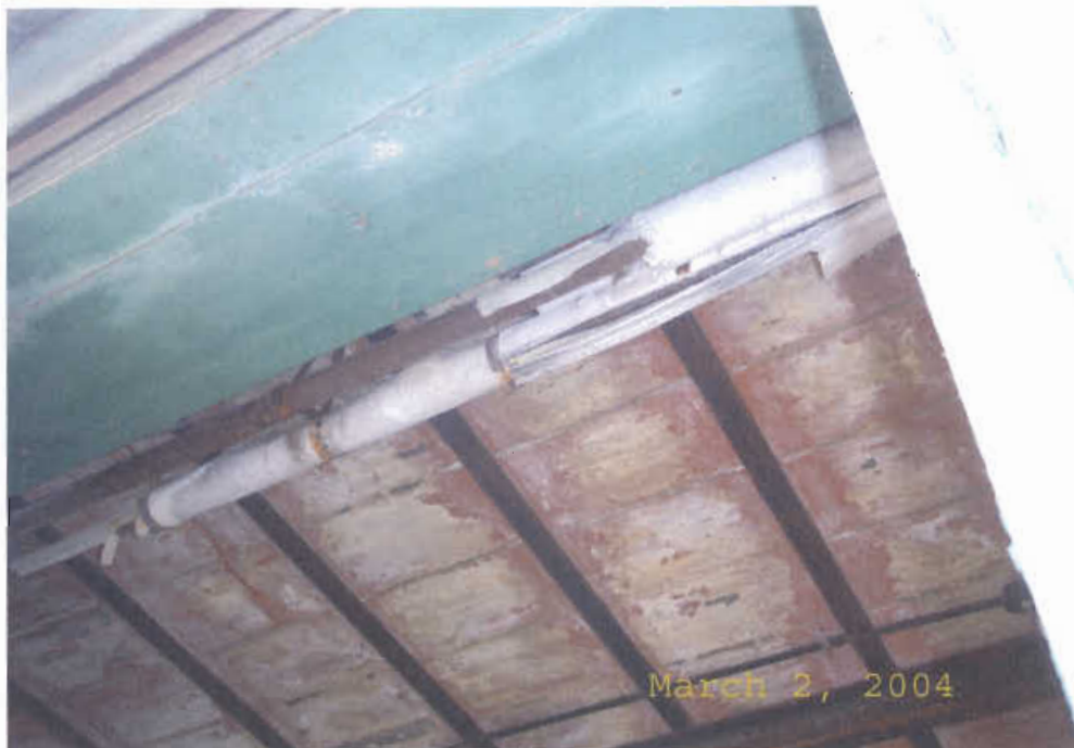
4 - ACM: Pipe Insulation
