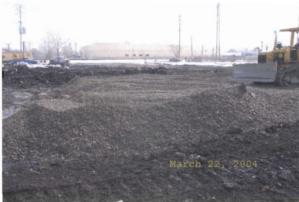
11 - #2 Stone Backfill
