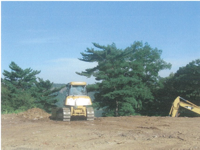
2. Site area location with machines.
