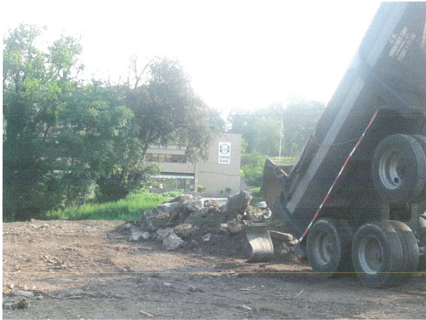
3. Trucks dumping stones for fill.
