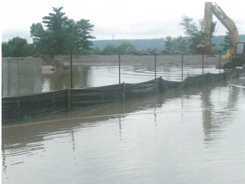
12. Rain water was helpful in reducing dust onsite.
