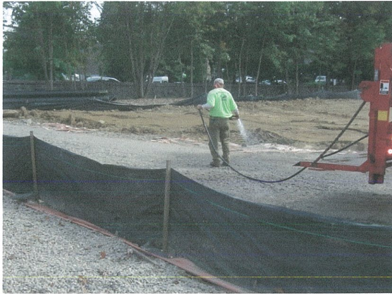
10. Spraying water as part of dust suppression.
