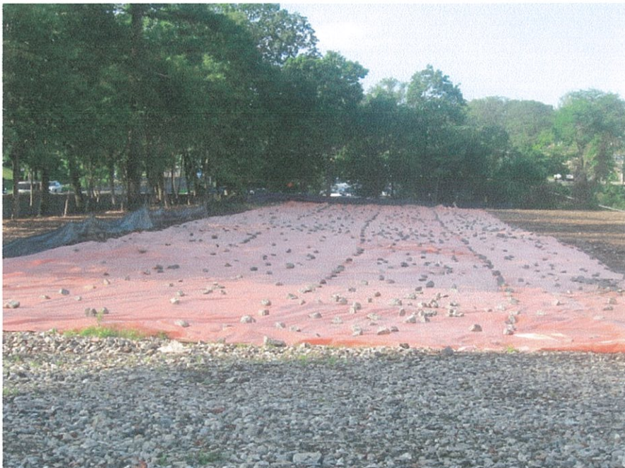
6. Using fabric paper to reduce dust.
