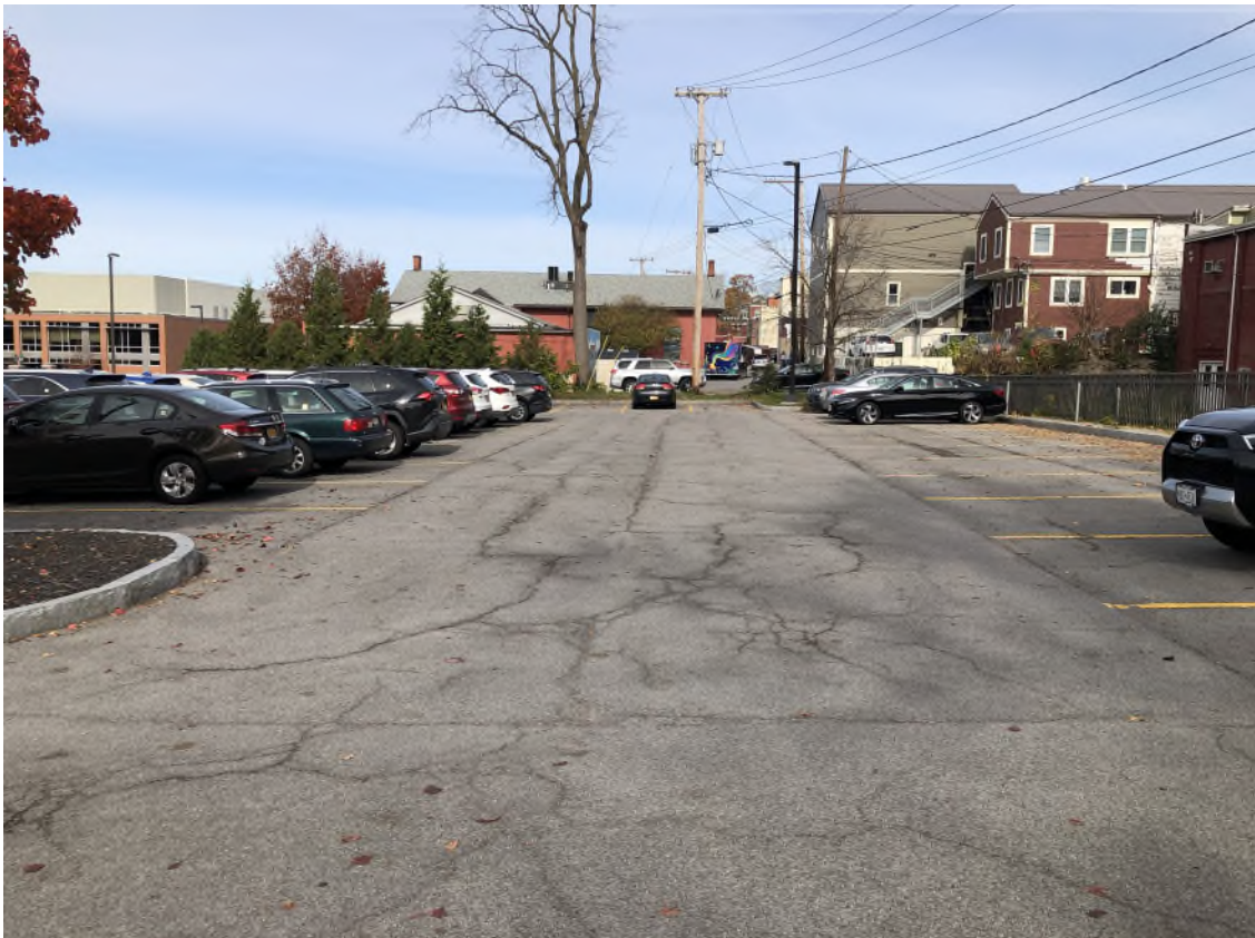
Asphalt cover, eastern portion of Parking Lot L - viewing north
